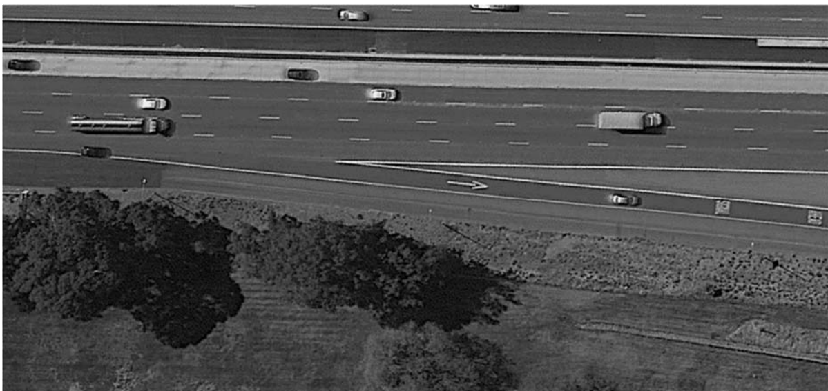
Figure 4-23. Example of California Site with No SCL (Image Credit: Google Earth™ Mapping Service).
