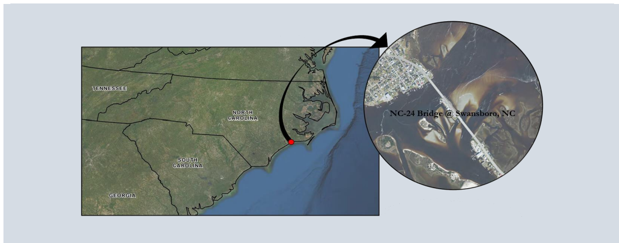
Figure 17. NC-24 Bridge at Swansboro, NC.
