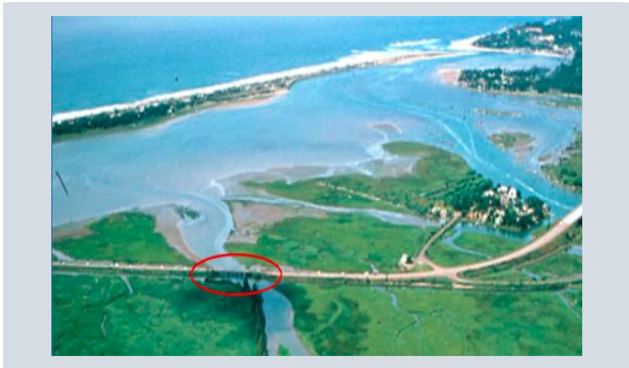
Figure 20. Millport Slough Bridge for the ODOT pilot project.
