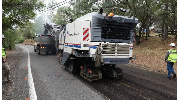
(a) (b) Figure B-5. Milling: (a) Milling Machine, (b) Tack Coat.
