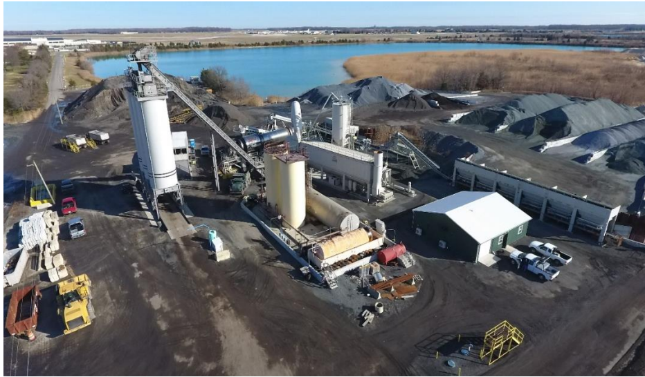
Figure A-3. Overview of the Asphalt Plant at Dover, Delaware.
