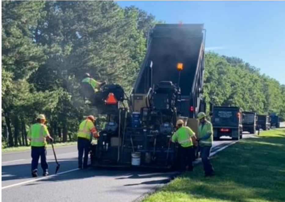
Figure A-6. Dump Trucks and Paver.
