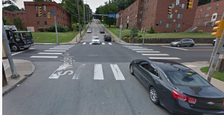
Significant uphill grade adjacent to an intersection.
