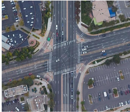
Intersection with channelized turn lanes.
