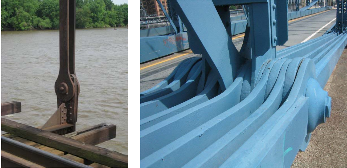
Figure C-1. Photographs of various eyebar configurations.
