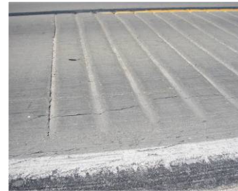
Example Rumble Strip Application (Source: Iowa DOT Design Manual, 6A-7)
