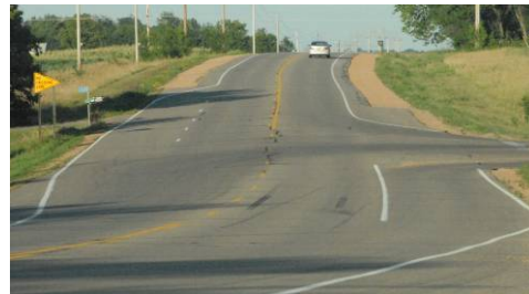
Example Bypass Lane at a T-Intersection (Source: Minnesota DOT Design Manual, Figure 5-4.01A)
