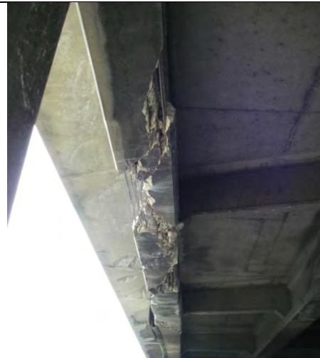
12 th Street over IH35, Austin TX AASHTO I-girder; strands appear intact (fig b), repair shown in fig d [Courtesy of the Texas Department of Transportation, © 2007 All rights reserved.]
