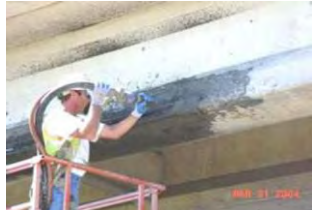
e) shotcrete patch
