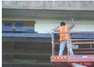
n) application of top coat
