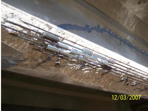
a) strand splices in situ [Courtesy of the Texas Department of Transportation, © 2007 All rights reserved.]
