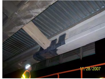
b) second repair confined with CFRP
