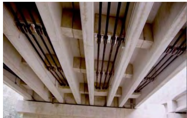
b) PT-CFRP anchored and harped by diaphragms [Mamlouk and Zaniewski Materials for Civil and Construction Engineers 2011]
