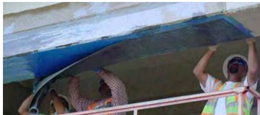
j) application of first ply of CFRP
