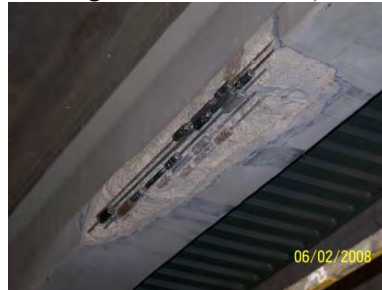
d) strand splice repair
