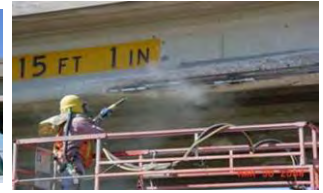
d) sandblasting in preparation for patching
