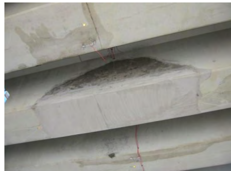
d) completed repair
