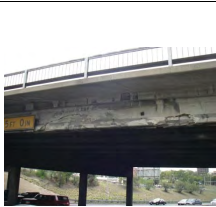
Impact damage to SC bridge structure AASHTO I-girder; bridge shown in service [Harries]
