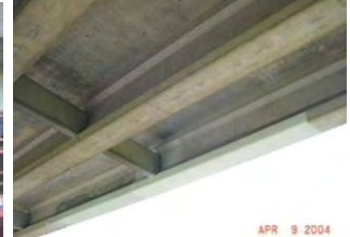
o) completed repair
