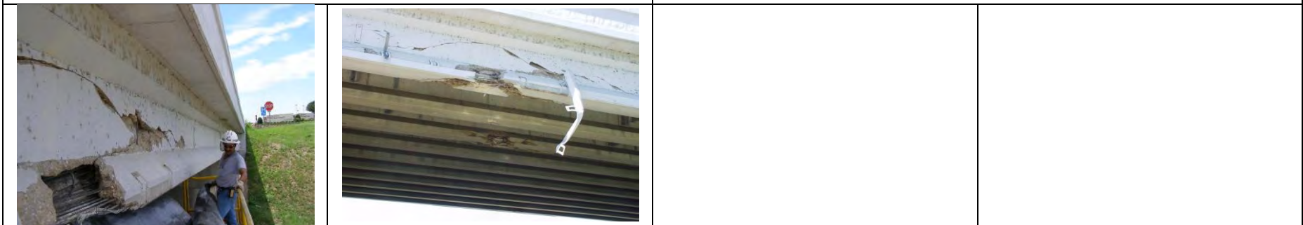
US B67 over US 67 AASHTO I-girder; reportedly repaired [Courtesy of the Texas Department of Transportation, © 2007 All rights reserved.]
