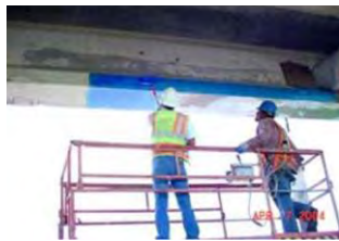
i) application of saturant
