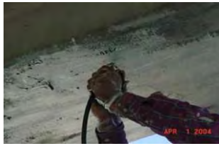
f) epoxy injection of cracks
