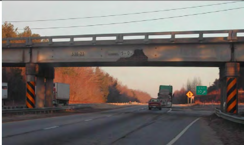
Impact damage to SC bridge structure AASHTO I-girder; bridge shown in service [Harries]
