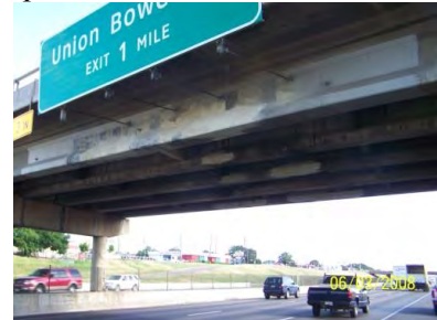
e) completed third repair
