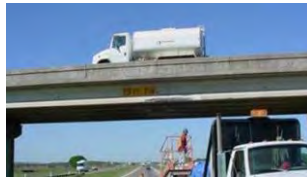
c) preload applied prior to patching
