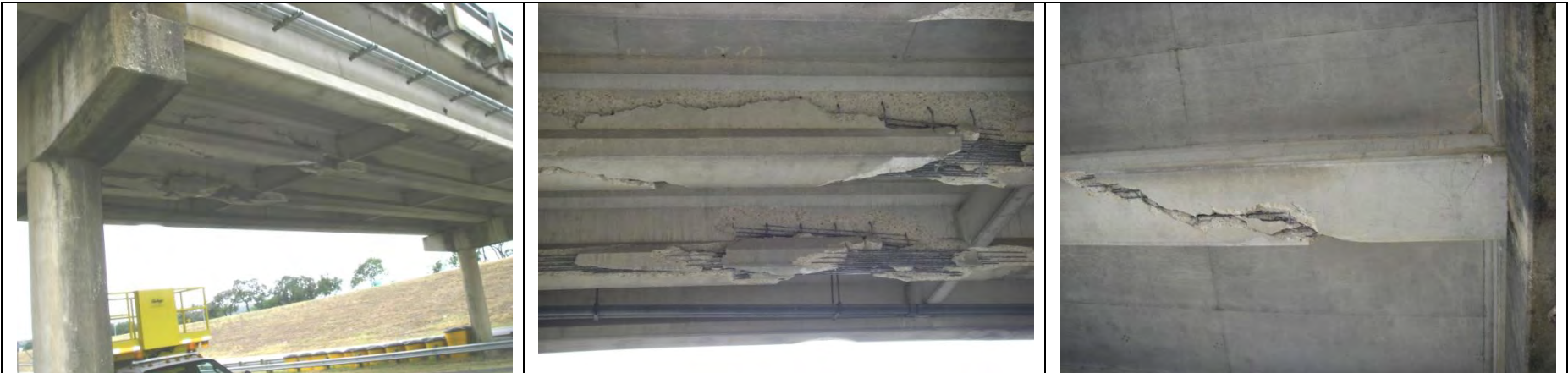
FM3351 over IH10 AASHTO I-girder; reportedly repaired [Courtesy of the Texas Department of Transportation, © 2007 All rights reserved.]
