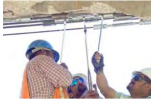
b) strand splices were tensioned
