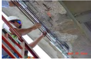
a) five strands were spliced
