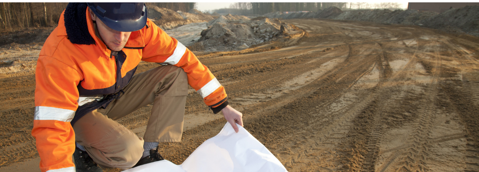
Figure 6: Engineer on worksite
