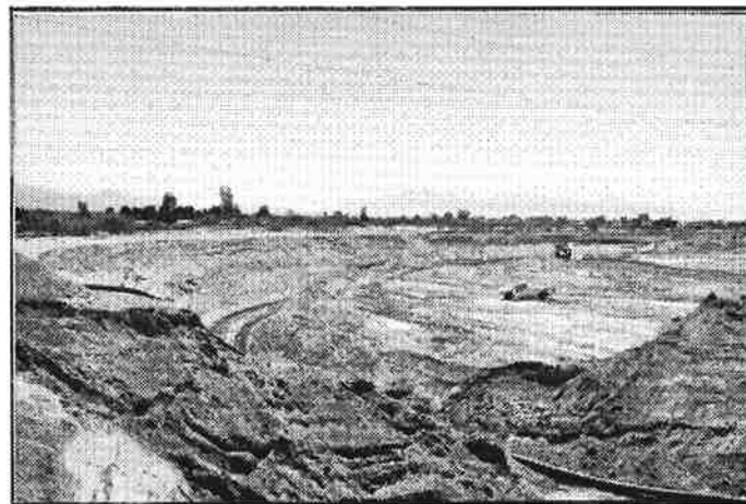
Figure 7.7. Shows a new soil-cement structure under construction.
