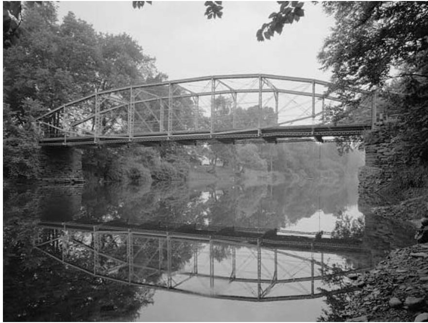
Figure 3-40. Nicholson Township Lenticular Bridge (1881), spanning Tunkhannock Creek at State Route 1029, Nicholson vicinity, Wyoming County, Pennsylvania. This bridge is an example of the through lenticular truss.
