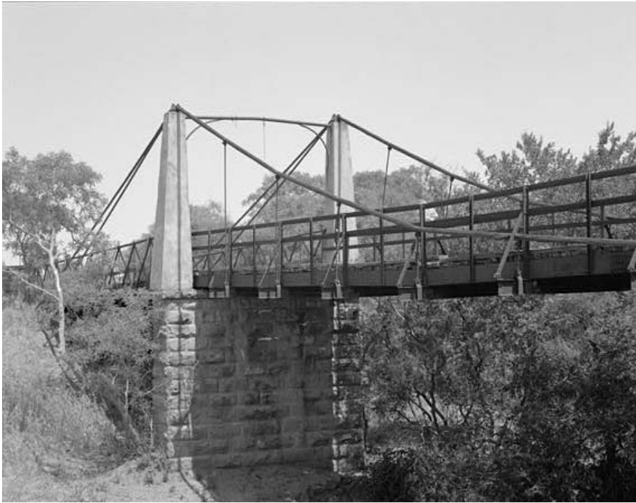
Figure 3-101. Clear Fork of Brazos River Suspension Bridge (1896), Shackelford County, Texas. The original cables have been replaced and the towers encased in concrete on this 312-foot long bridge.
