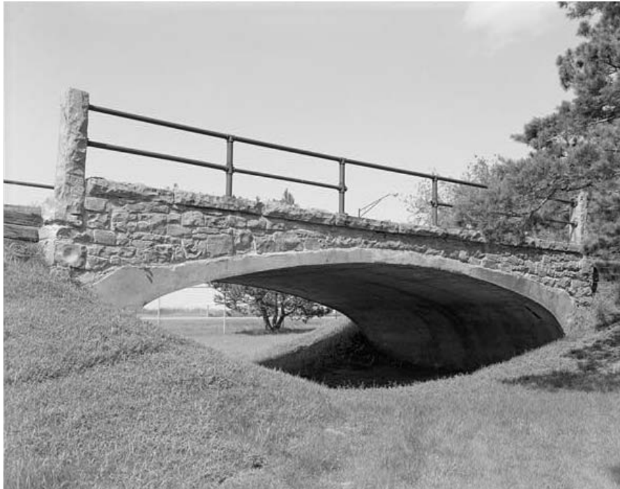
Figure 3-49. Sandy Hill Bridge, Bridge Street (1906-07), spanning Hudson River, Hudson Falls, New York. This structure was built using the Melan system.
