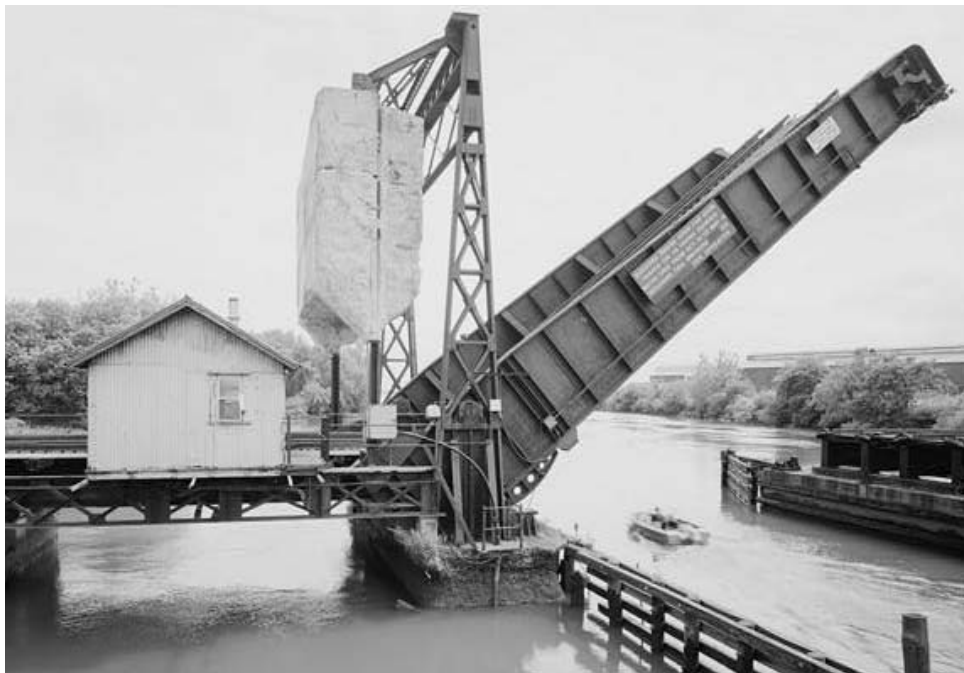
Figure 3-94. Philadelphia, Baltimore & Washington Railroad, spanning Darby Creek, Eddystone, Pennsylvania. This Strauss Bascule Bridge Company-designed structure was fabricated and built by Bethlehem Steel.
