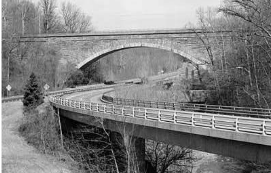
Figure 3-45. Cabin John Aqueduct Bridge (1864), MacArthur Boulevard, spanning Cabin John Creek at Cabin John, Maryland. With a single arch span of 220 feet, this bridge was the longest masonry arch bridge in the world until 1905.
