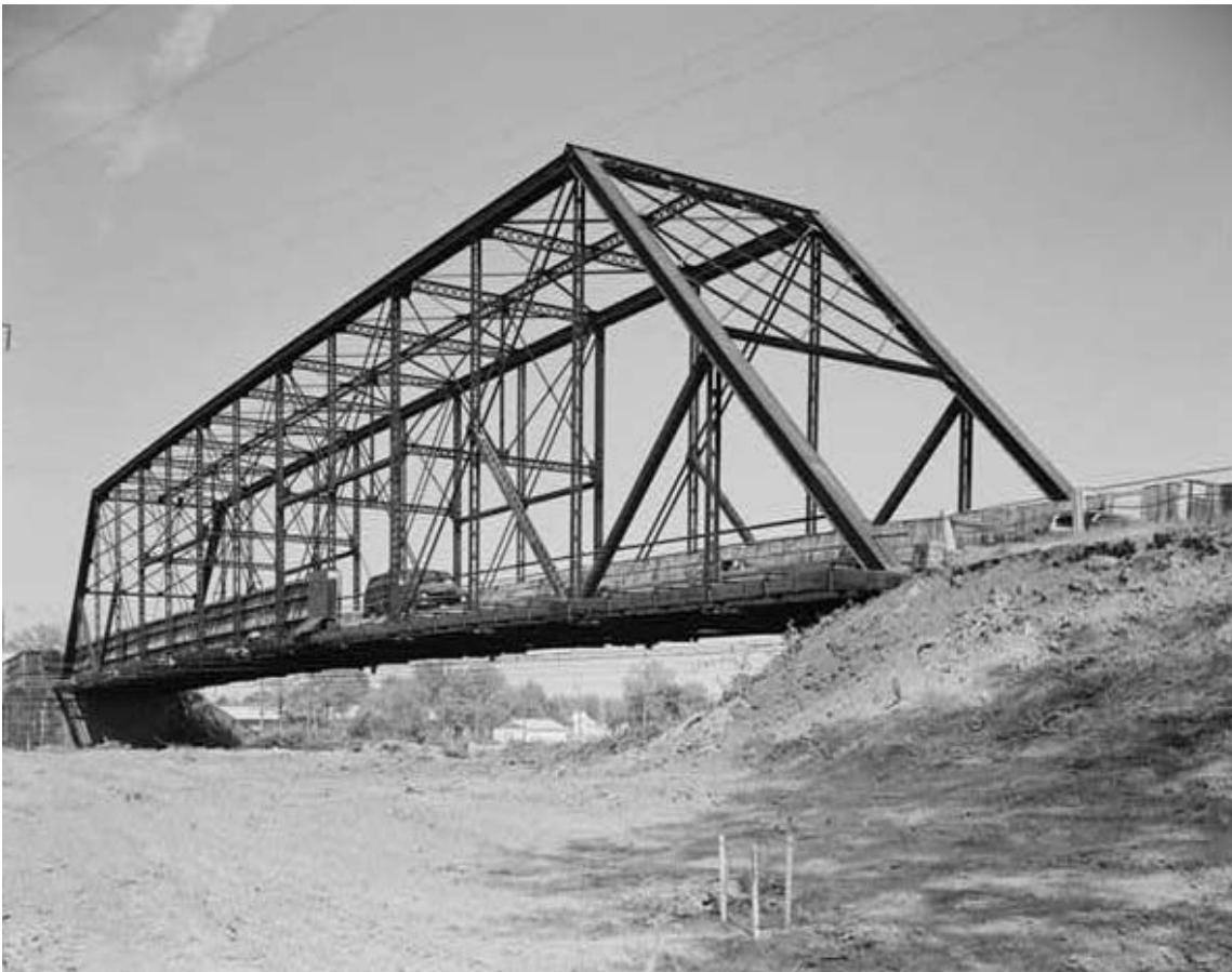
Figure 3-26. Post Road Bridge (1905), State Route 7A, Havre de Grace vicinity, Harford County, Maryland. This bridge is an example of the Baltimore truss type.
