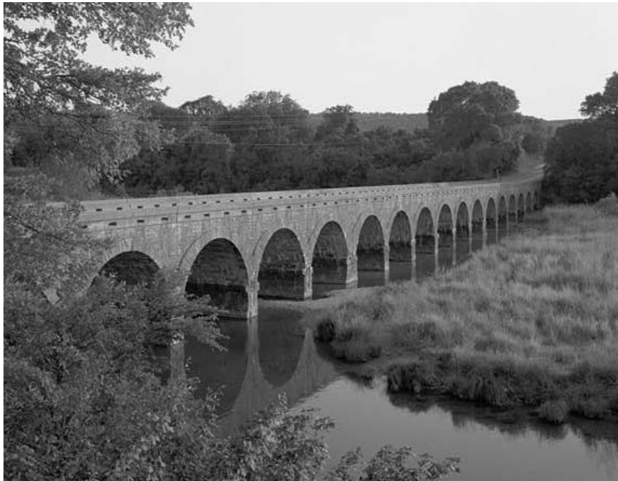
Figure 3-46. Possum Kingdom Stone Arch Bridge (1940-42), spanning Brazos River at State Route 16, Graford, Texas. This structure is an example of a Works Progress Administration-built stone arch bridge.
