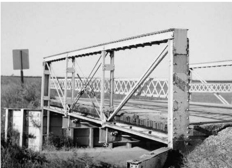
Figure 3-21. Burrville Road Bridge (1887), spanning Toti Creek Mercer County, Ohio. This structure is an example of the bedstead Pratt truss.
