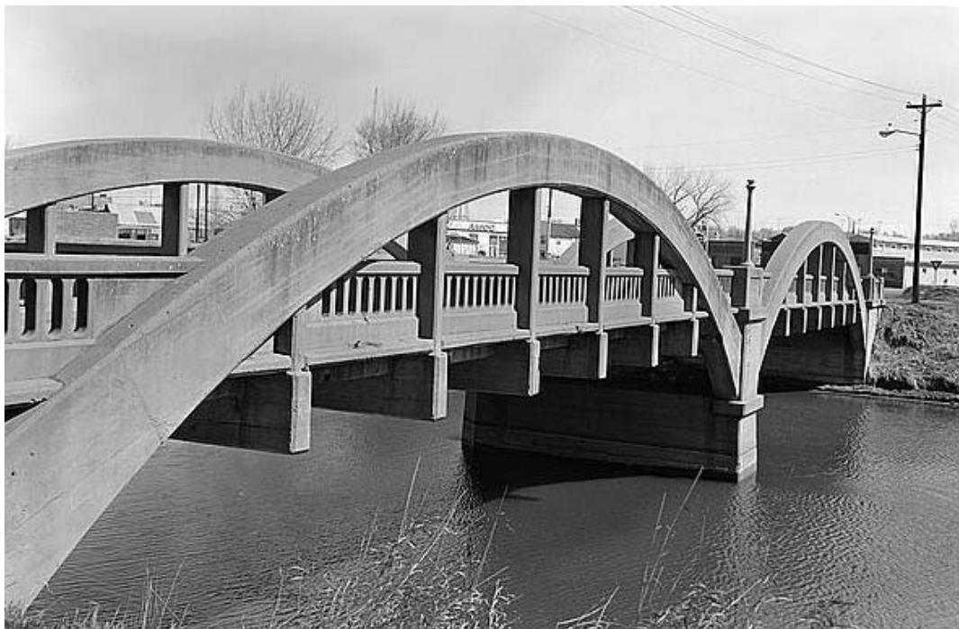
Figure 3-53. Mott Rainbow Arch Bridge (1921), spanning Cannonball River, Mott, North Dakota. This two-span bridge is an example of the patented Marsh arch.
