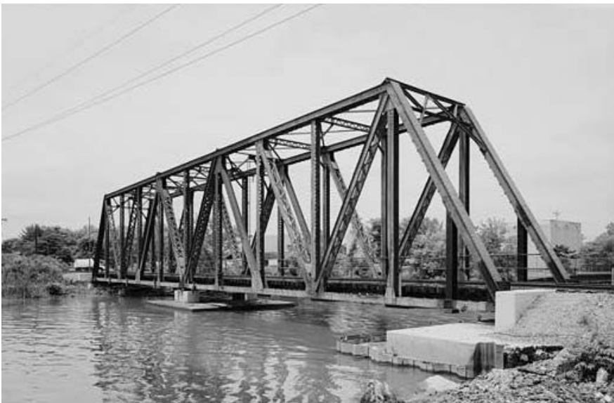
Figure 3-87. Chester & Delaware River Railroad (1907), spanning Chester Creek, Chester, Pennsylvania. When built, this swing bridge was hand operated.
