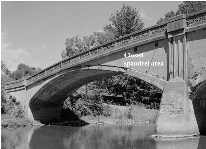
Figure 3-55. Penns Creek Bridge (1919), State Route 1014 at Penns Creek, Selinsgrove vicinity, Snyder County, Pennsylvania. This bridge is an example of a reinforced closed spandrel concrete structure.
