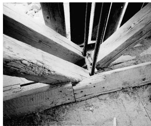
3-14b. Detail of the lower joint of the tension/compression members at the
