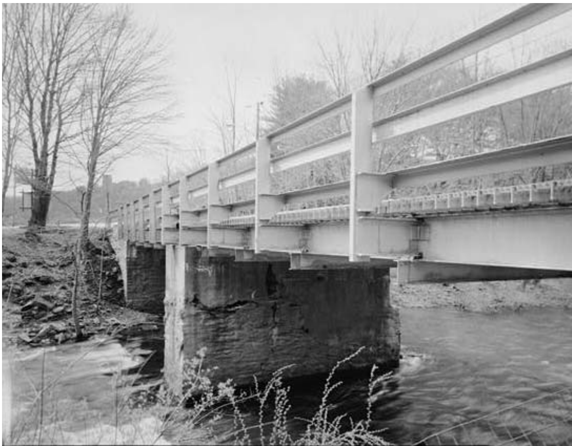
Figure 3-81. Parryville Bridge (1933), State Route 2008 over Pohapoco Creek, Parryville, Pennsylvania. This bridge is an example of the metal rolled multi-beam type.
