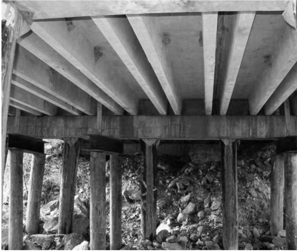
Figure 3-72. Bridge on Cannafax Farm Road over Little Potato Creek in Lamar County, Georgia. View of concrete channel beams.
