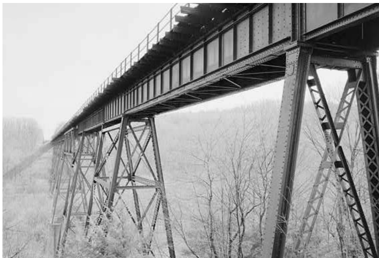
Figure 3-108. Mahoning Creek Trestle (1899), spanning Mahoning Creek, Goodville vicinity, Indiana County, Pennsylvania. This high steel structure was built to carry the railroad.
