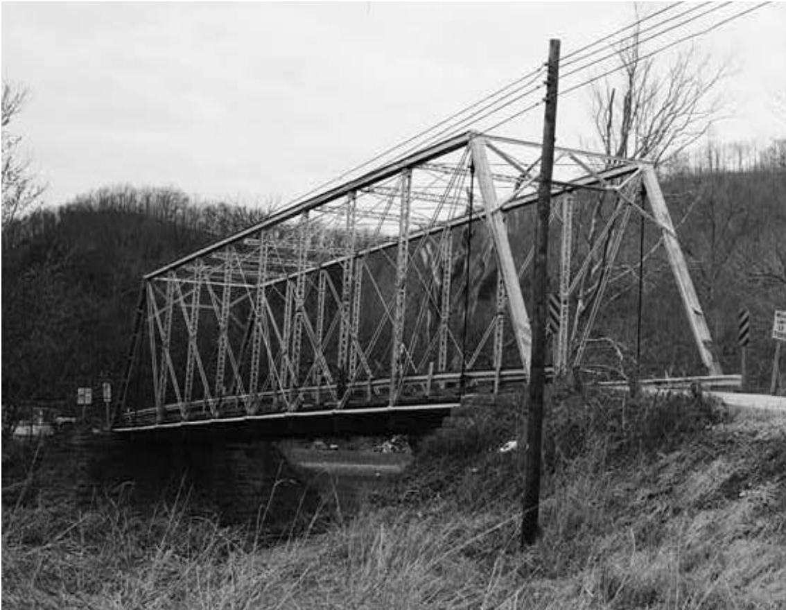
Figure 3-23. Kentucky Route 49 Bridge (1881), spanning Rolling Fork River, Bradfordsville, Marion County, Kentucky. This bridge is an example of the double intersection Whipple truss.
