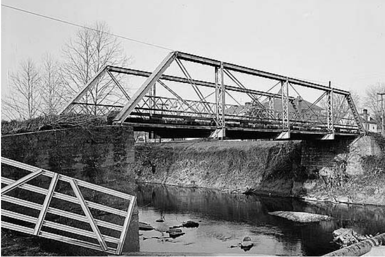
Figure 3-19. Daphna Creek Pratt Truss Bridge (ca. 1900), Rockingham County, Virginia. This Canton Bridge Company structure is an example of the pony Pratt.
