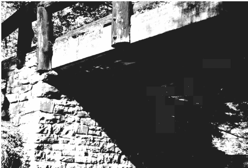
3-79b. Underside of box beams at stone abutment.
