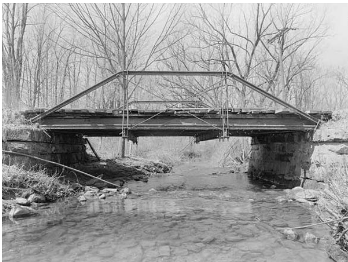
Figure 8. Mercer County Bridge No. 2631 (ca. 1894), spanning Pine Run at Cribbs Road, Mercer vicinity, Mercer County, Pennsylvania. This small structure is a late nineteenth century metal queen post truss.
