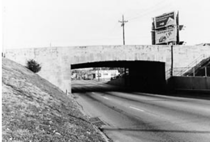
Figure 3-77. Merritt Parkway (ca. 1948), Comstock Hill Road Bridge, spanning Merritt Parkway, Norwalk, Fairfield County, Connecticut. Below is a historic (a) and current (b) photograph of one of the approximately seventy rigid frame bridges on the Merritt Parkway.
