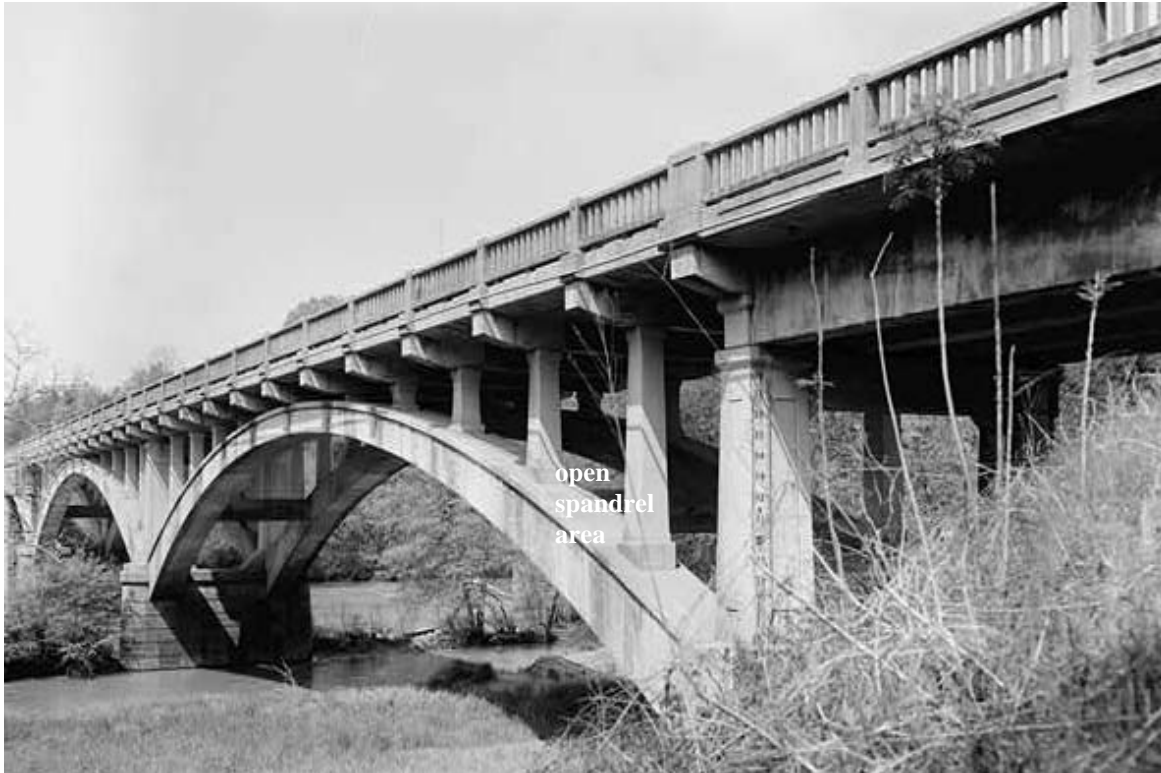
Figure 3-57. Broad River Highway Bridge (1935), State Route 72, spanning Broad River, Carlton vicinity, Madison County, Georgia. This bridge is an example of the open spandrel concrete arch.
