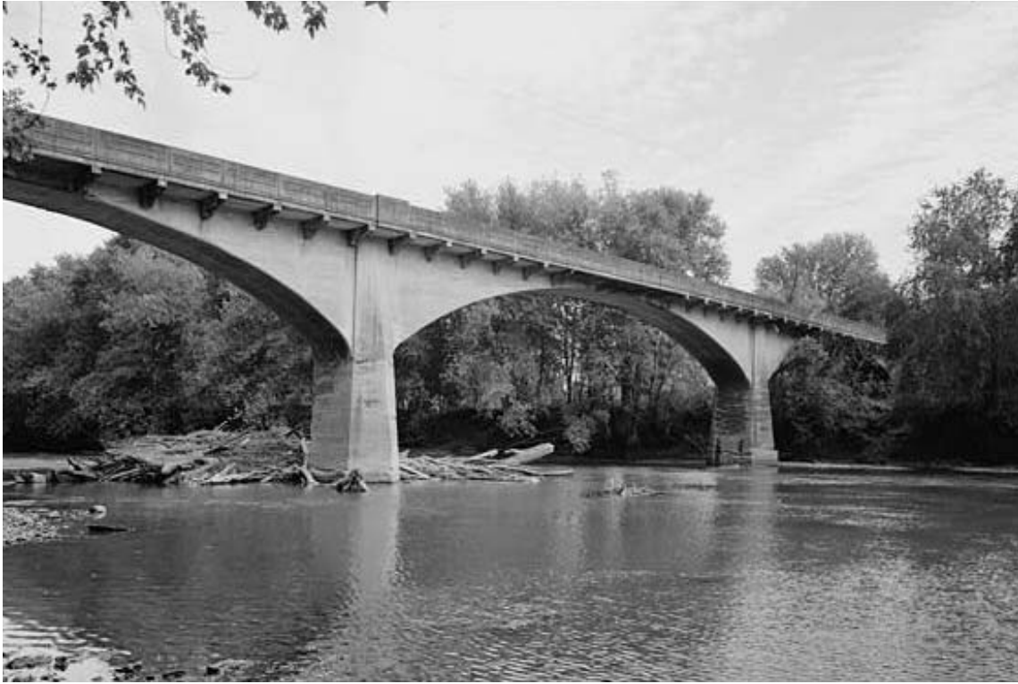
Figure 3-50. Andrew J. Sullivan Bridge (1928), spanning Cumberland River, Williamsburg vicinity, Whitley County, Kentucky. This structure is an example of a Luten closed spandrel arch.
