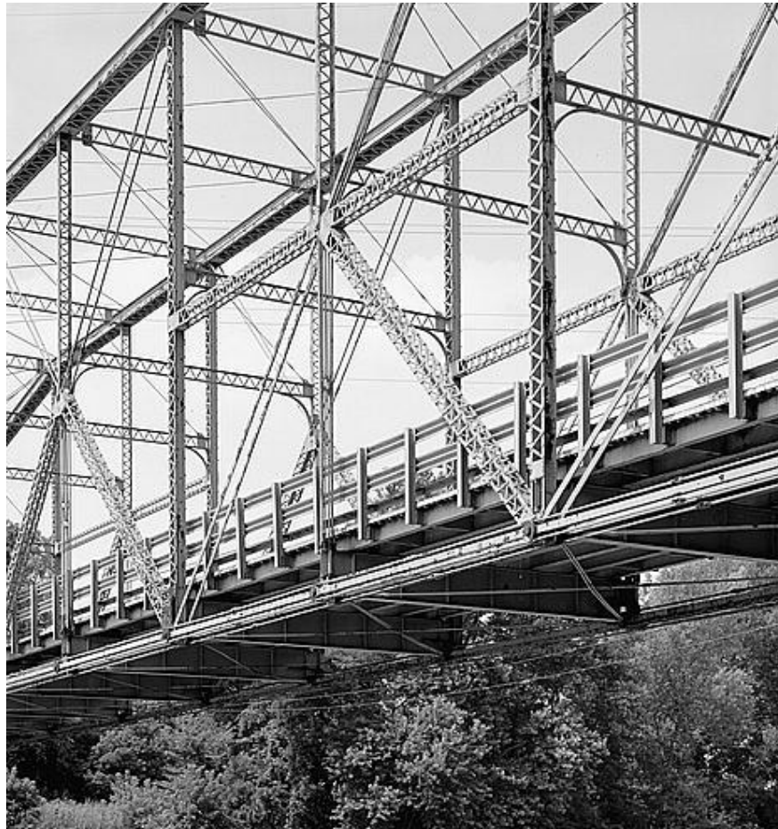
Figure 3-31. Old Colerain Bridge (1894), spanning Great Miami River at County Route 463, Hamilton County, Ohio. Detail of panel configuration, bottom chord, floor beams, and stringers of Pennsylvania truss bridge.
