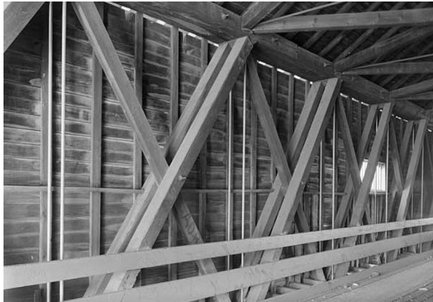
3-15b. The interior of the structure. Note the Howe truss's heavy wood diagonal members (in compression) and lighter, vertical cylindrical iron members (in tension).
