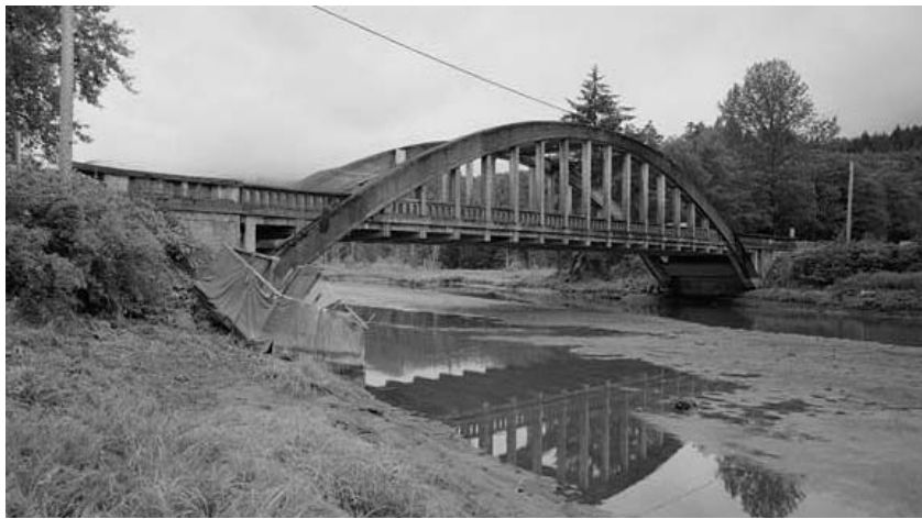
Figure 3-63. North Hamma Hamma River Bridge (1923); Mason County, Washington. This structure is a three-hinged concrete arch bridge built by Washington State Highway Department.
