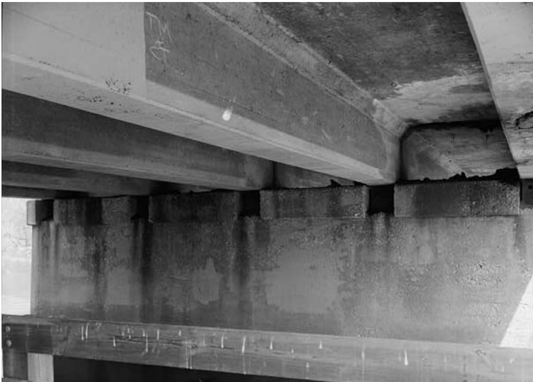
3-71b. View of T-Beams on underside of superstructure.
