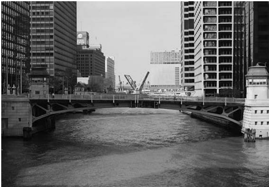
Figure 3-91. Chicago River Bascule Bridge (1916), Jackson Boulevard, Chicago, Illinois. This simple trunnion, double leaf bascule was a product of the Strauss Bascule Bridge Company.
