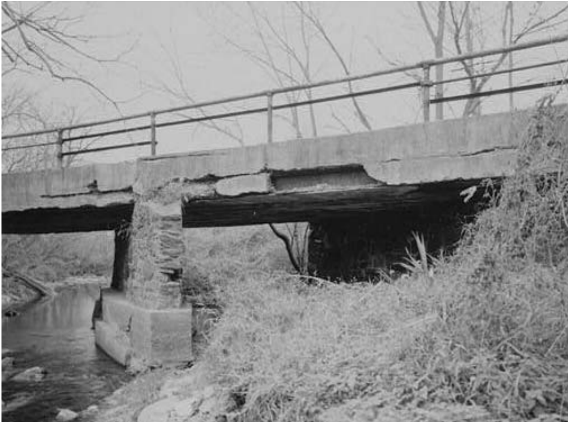
Figure 3-69. Hartford Road (1943) over a branch of West Creek on Hartford Road (CR 5), Sebastian County, Arkansas. This concrete slab bridge has a stone substructure and an open concrete rail and was built by the Works Progress Administration during World War II. (Photographs from Historic Bridges of the Midwest , found at http://bridges.midwestplaces.com/ .)
