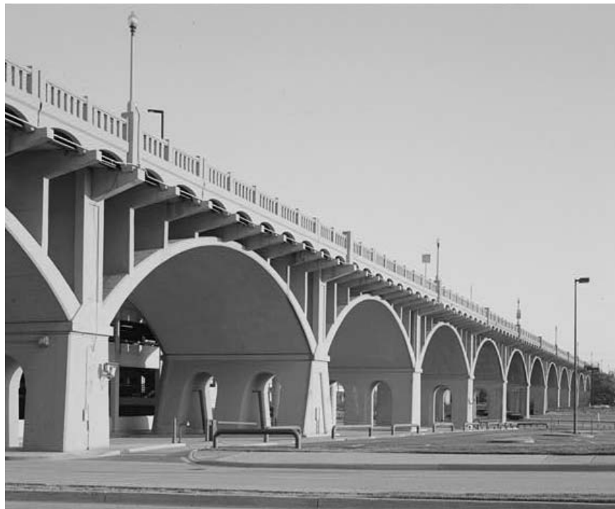
Figure 3-105. Dallas-Oak Cliff Viaduct (1910-12), spanning Trinity River at Houston Street, Dallas, Texas. This early twentieth century viaduct is a concrete open spandrel arch.
