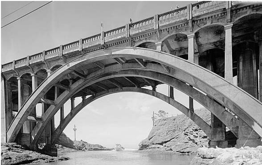
Figure 3-64. Depoe Bay Bridge (1927), Lincoln County, Oregon. This Oregon coast hinged concrete arch bridge spans the bay between Newport and Lincoln City.
