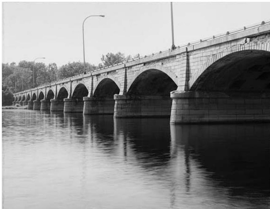
Figure 3-49. Sandy Hill Bridge, Bridge Street (1906-07), spanning Hudson River, Hudson Falls, New York. This structure was built using the Melan system.
