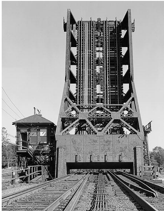
3-97b. Detail of control house and lift in open position.
