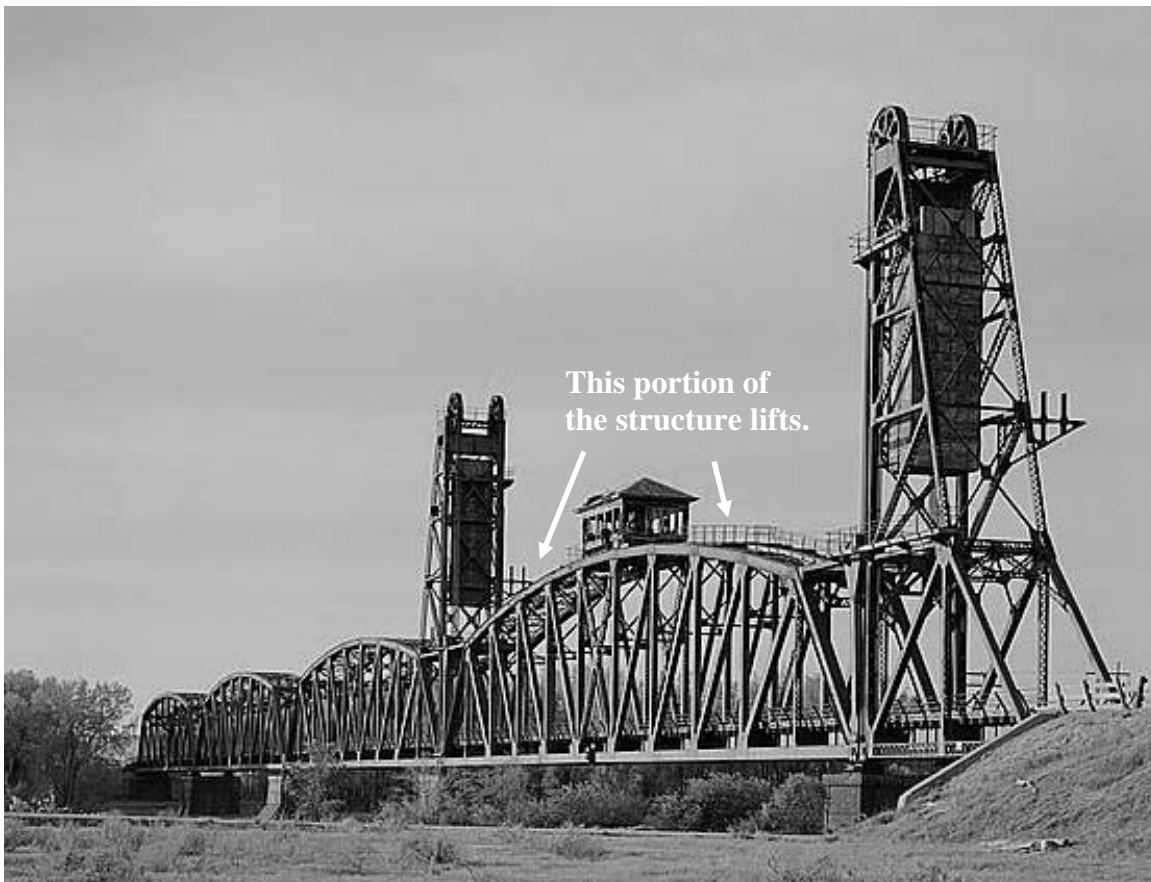
Figure 3-90. Snowden Bridge (1913), spanning Missouri River, Nohly vicinity, Richland County, Montana. This structure is an example of a vertical lift.
