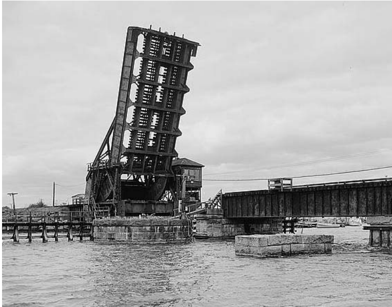
3-97a. Scherzer rolling lift in open position.
