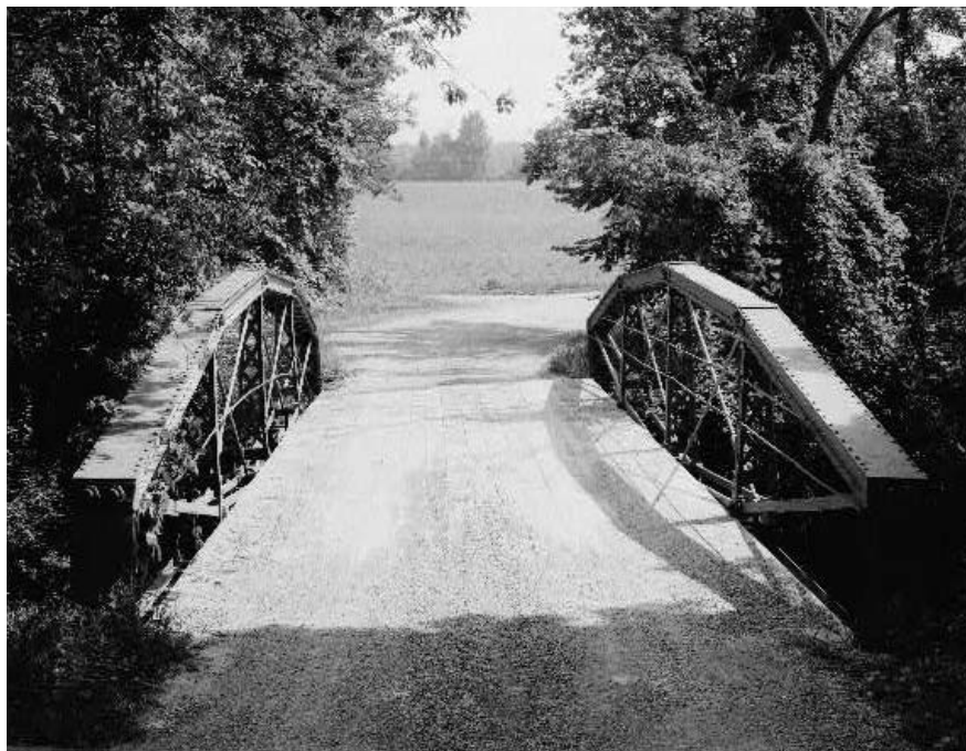
Figure 3-41. Nicholson Bridge (1888), Cemetery Road spanning Black Creek, two miles Southwest of Salem, Washington County, New York. This bridge is an example of the pony lenticular truss.
