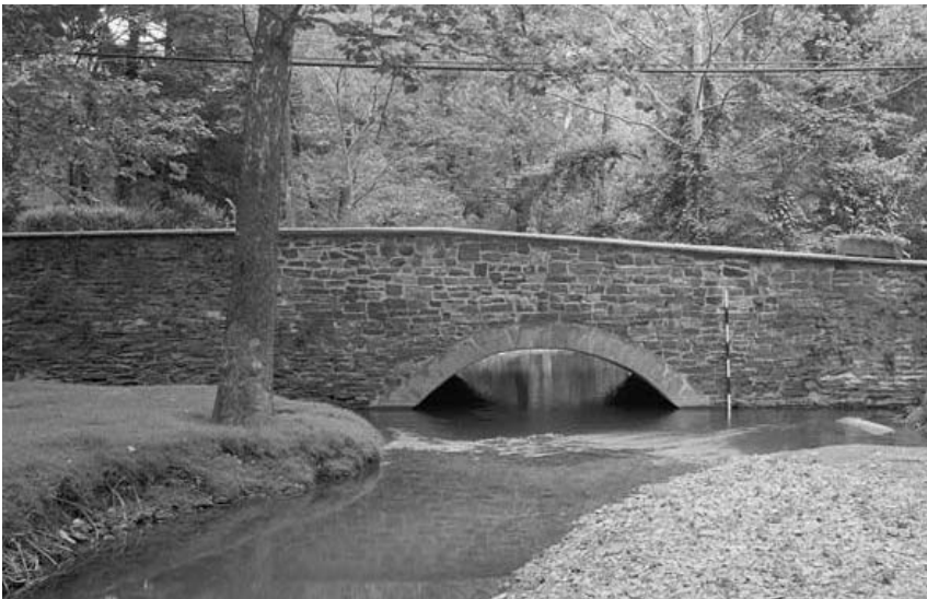
Figure 3-43. Gulph Creek Stone Arch Bridge (1789), Old Gulph Road, Upper Merion, Montgomery County, Pennsylvania. This eighteenth century stone arch bridge is one of the oldest surviving bridges in Pennsylvania.
