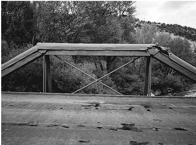
Figure 7. Hortense Bridge, spanning Chalk Creek on State Highway 162 (1880), Nathrop vicinity, Chaffee County, Colorado. This bridge is an example of a queen post truss built by Denver South Park & Pacific Railroad.
