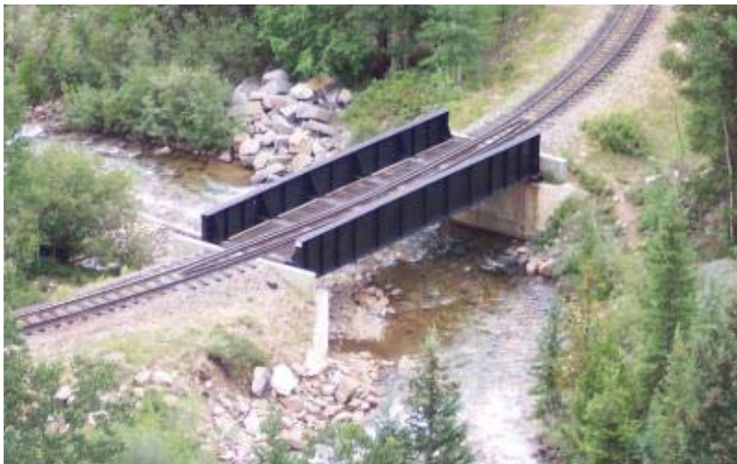
Figure 3-82. Georgetown Loop Plate girder Bridge (n.d.), Clear Creek County, Colorado. This railroad bridge is a metal built-up girder. Photograph from Historic Bridges of the Midwest .
