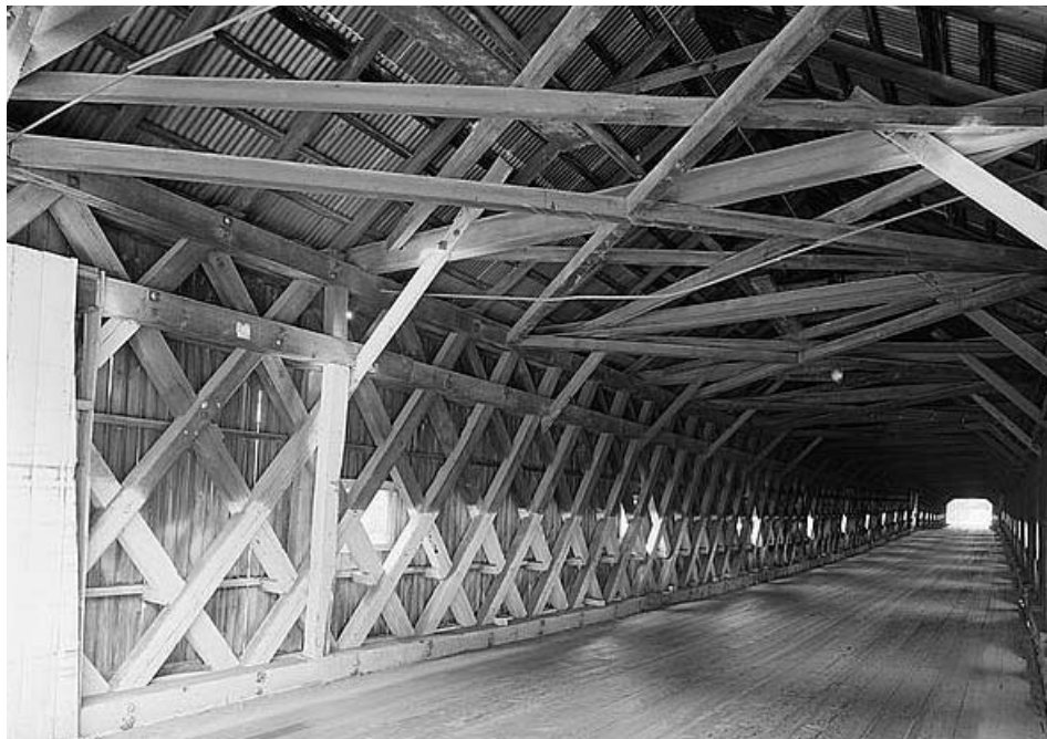
3-12b. Interior view of Cornish-Windsor covered bridge showing the intersecting diagonals that form a web between the top and bottom chords.
