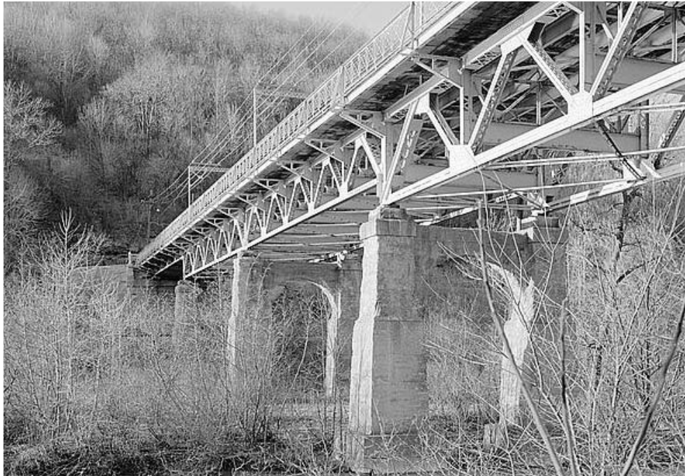
Figure 3-35. Fifficktown Bridge (1910), spanning Little Conemaugh River, South Fork, Cambria County, Pennsylvania. This structure is an example of the Warren deck truss.
