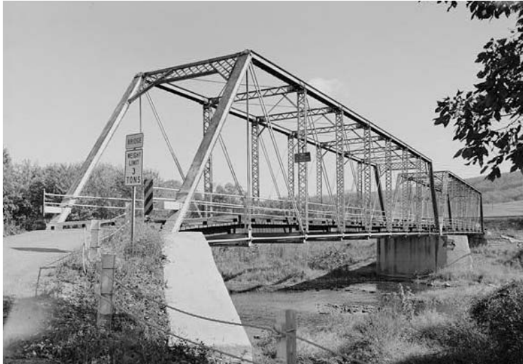
Figure 3-20. Runk Bridge (n.d.), Shirleysburg, Huntingdon County, Pennsylvania. This structure is an example of a through Pratt truss.
