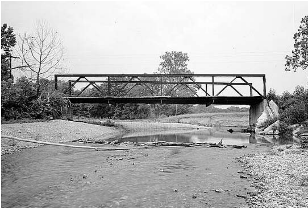
Figure 3-36. Spavinaw Creek Bridge (1909), Benton County Road 29 spanning Spavinaw Creek, Gravette vicinity, Benton County, Arizona. This structure is an example of the Warren bedstead truss.
