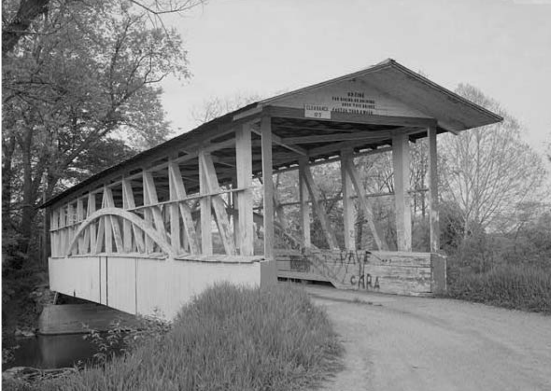
Figure 3-10. Raystown Covered Bridge (1892), Township Route 418 spanning Raystown Branch, Manns Choice vicinity, Bedford County, Pennsylvania. The uncovered sides of this structure reveal the Burr arch.
