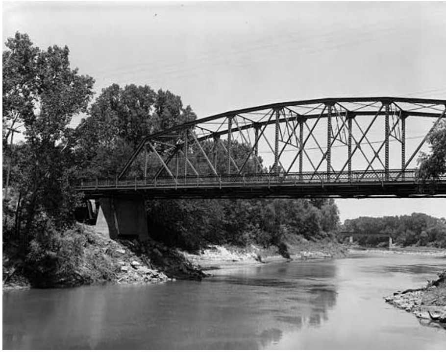
Figure 3-28. Enterprise Bridge (1924-25), spanning Smoky Hill River on K-43 Highway, Enterprise, Dickinson County, Kansas. This structure is an example of a Parker truss.
