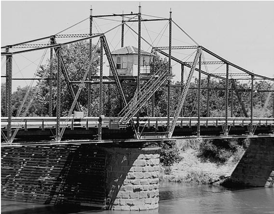
Figure 3-86. Colusa Bridge (1901), spanning Sacramento River, Colusa, California. The swing span of this bridge is pin connected.
