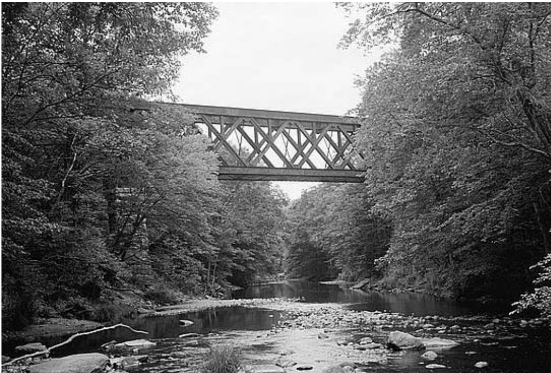
Figure 3-38. Bridge spanning Blackledge River (1907), Solchestes, New London County, Connecticut. This abandoned railroad bridge is an example of a double intersection Warren truss.
