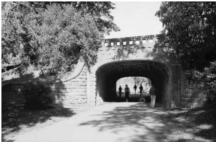
Figure 3-47. Alvord Lake Bridge (1889), San Francisco, San Francisco County, California. Designed by Ernest Ransome, this is the first reinforced concrete bridge in the United States.
