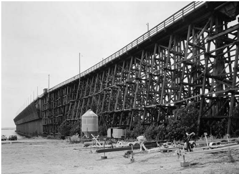
Figure 3-107. Marquette Ore Dock No. 6 Timber Trestle (1931-32), between East Lake Street & Ore Dock No. 6, Marquette City, Marquette County, Michigan. This structure is an example of a high timber trestle.
