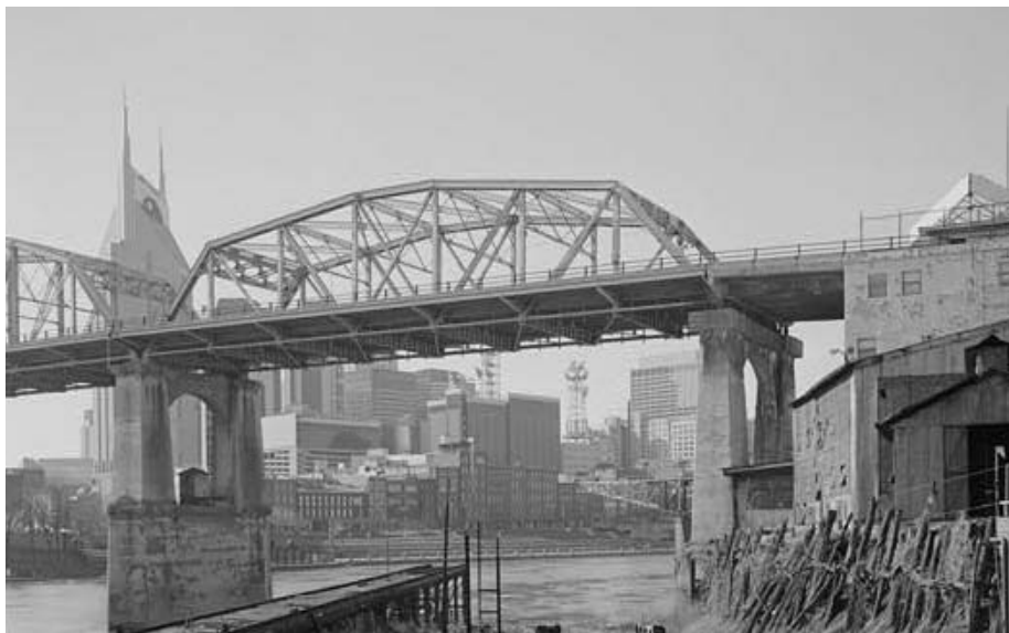
Figure 3-29. Sparkman (Shelby) Street Bridge (1907-09), spanning the Cumberland River, Nashville, Davidson County, Tennessee. This span is an example of the camelback variation of the Parker truss. Note the characteristic five slopes in the upper chord and end posts.
