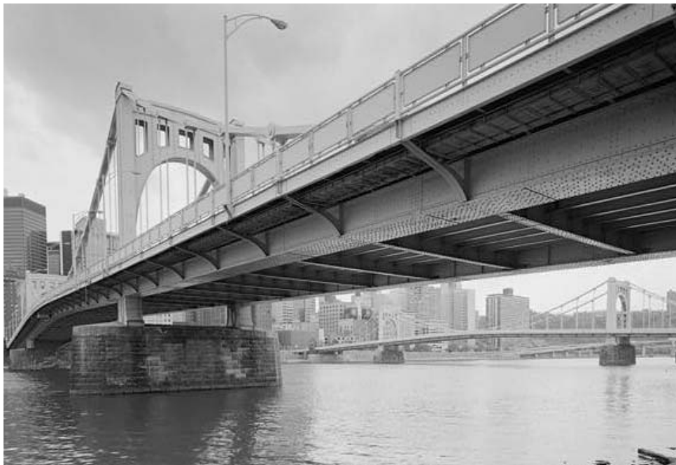
Figure 3-100. Seventh Street Bridge (1924-26), spanning Allegheny River at Seventh Street, Pittsburgh, Pennsylvania. One of the Three Sisters bridges, this self-anchored suspension bridge was designed by the Allegheny Department of Public Works and built by the American Bridge Company.
