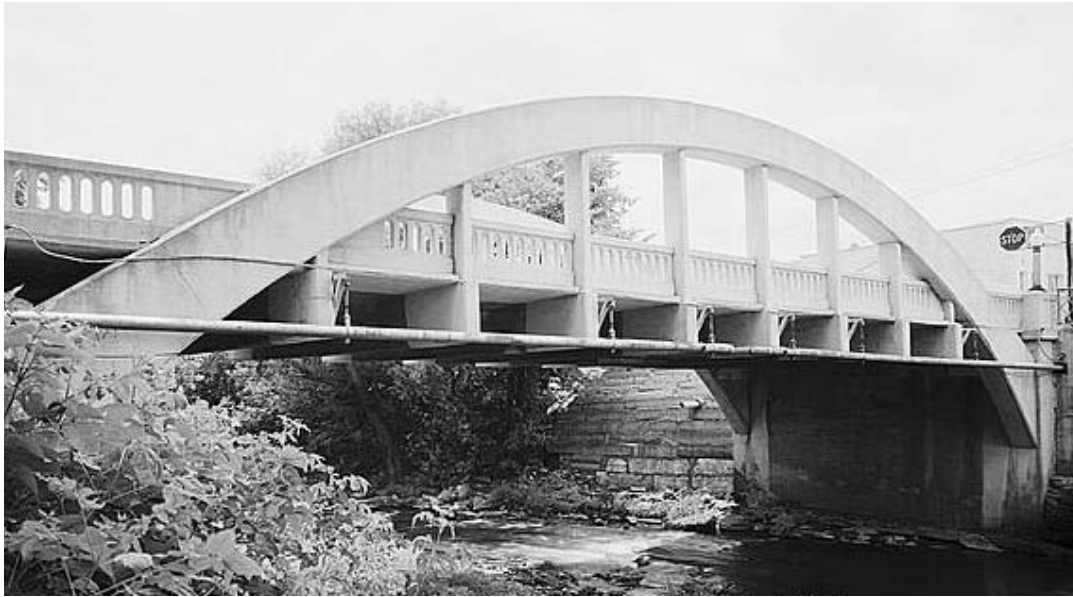
Figure 3-53. Mott Rainbow Arch Bridge (1921), spanning Cannonball River, Mott, North Dakota. This two-span bridge is an example of the patented Marsh arch.
