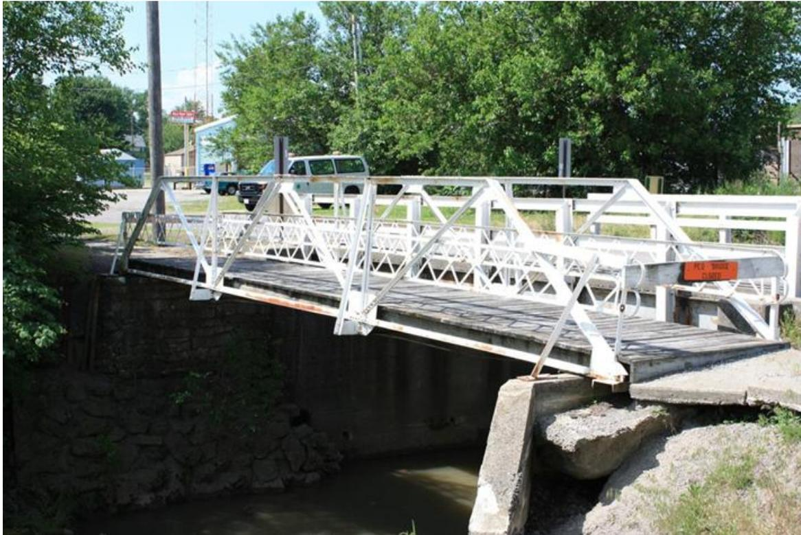
**Figure D-8:** Van Wert, Van Wert County, Ohio Petite Pony Truss Pedestrian Bridge
