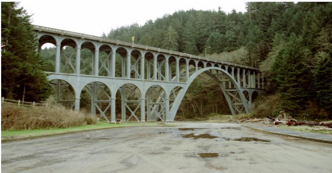
**Figure D -6-:** The Cape Creek Bridge (1927), Oregon, was the first bridge rehabilitated with full cathodic protection.
