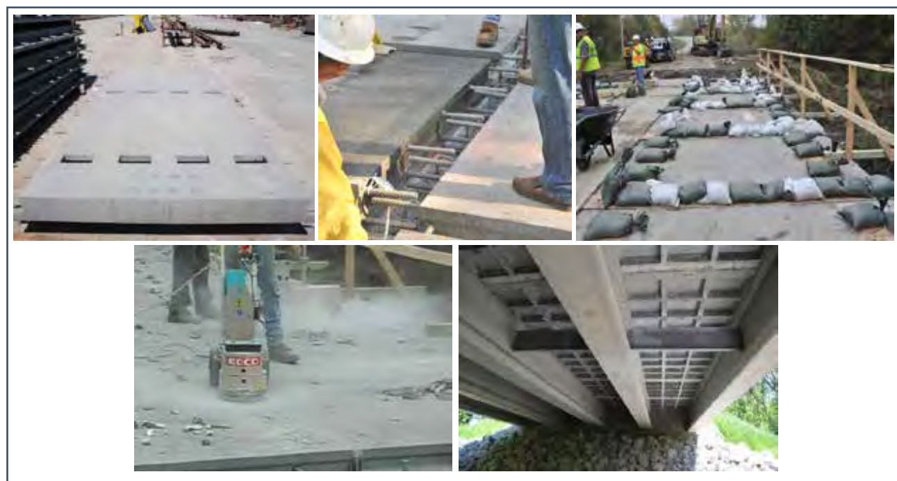
Figure 11. Prefabricated UHPC two-way ribbed (waffle shaped) bridge deck from Wapello County, Iowa
