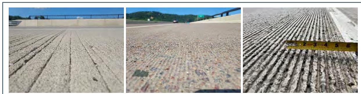
Figure 3. Transverse tining (left), longitudinal planing (middle), longitudinal groove (right) in Minnesota
