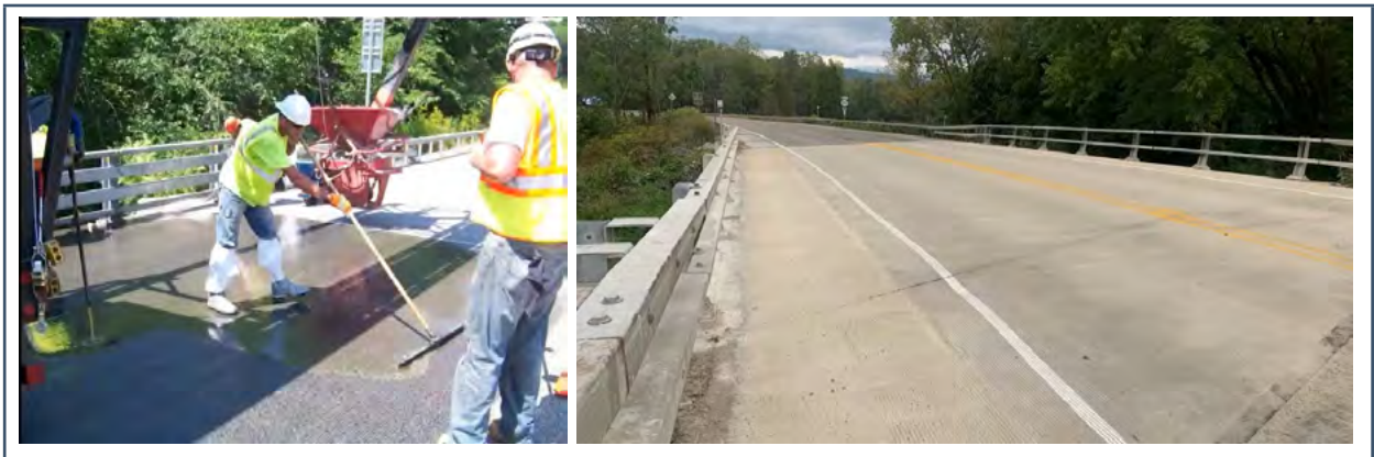
Figure 4. Thin polymer overlay, hybrid composite synthetic concrete (New York State)
