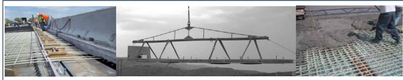
Figure 15. GFRP bars used for a redecking project in Kansas DOT, precast concrete deck panel with GFRP bars by Utah DOT, GFRP top mat with epoxy coated rebar bottom mat in Virginia
