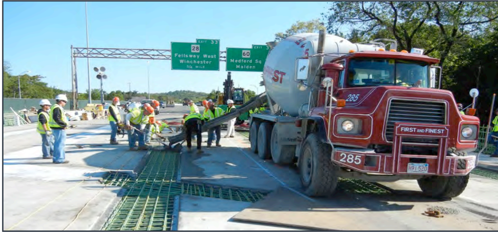
Figure 2.13 Deck closure pour construction in Massachusetts Fast 14
