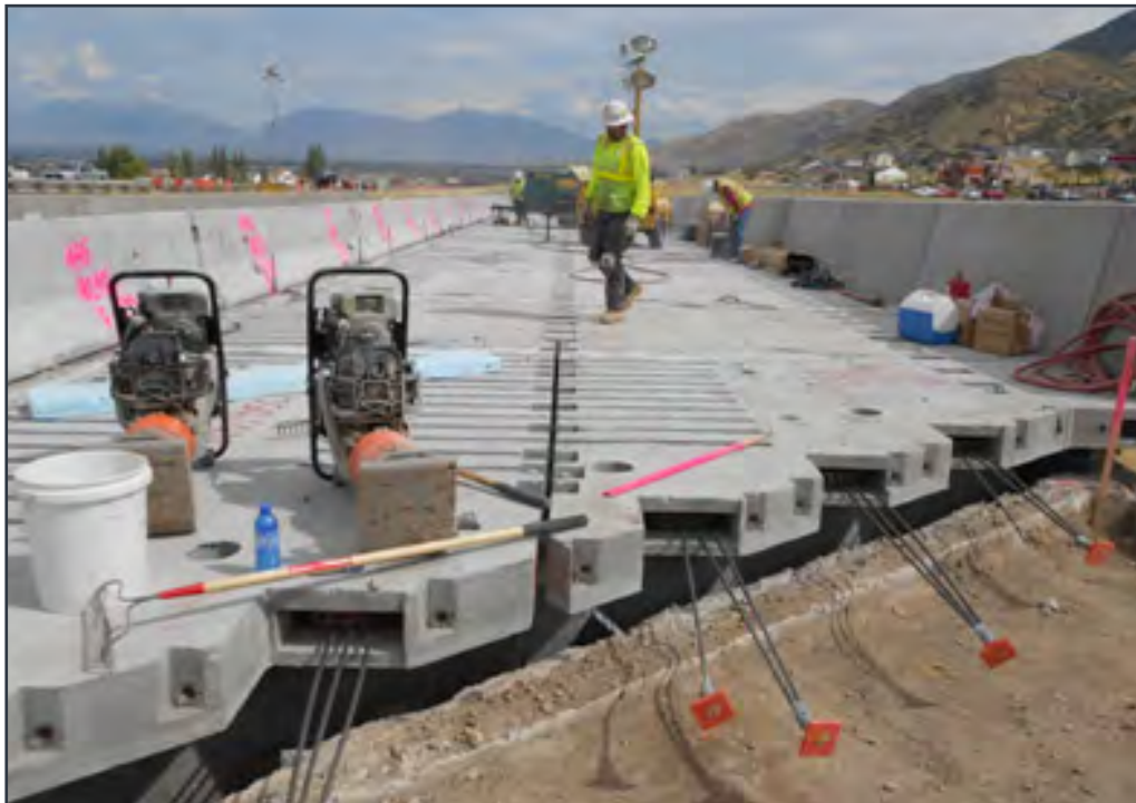
Figure 2.14 Deck post-tensioning in Utah
