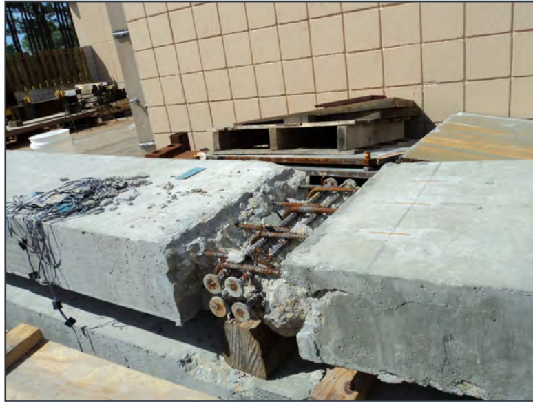
Figure 2.33 Full-depth deck slab connection model tested at the FDOT Testing Structure Research Center
