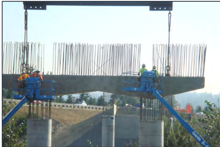
Figure 2.24 Placement of cap beam on column bars inserted in corrugated ducts in Washington State
