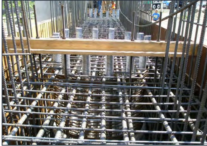
Figure 2.23 Corrugated ducts in precast cap beam in Washington State
