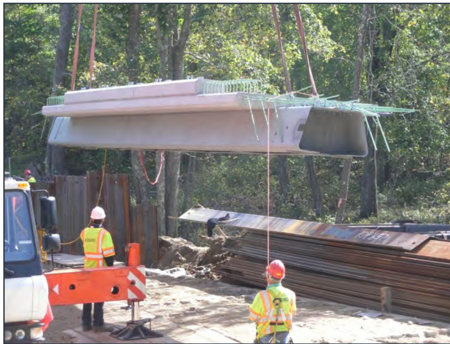
Figure 2.54 Folded plate girder bridge in Massachusetts
