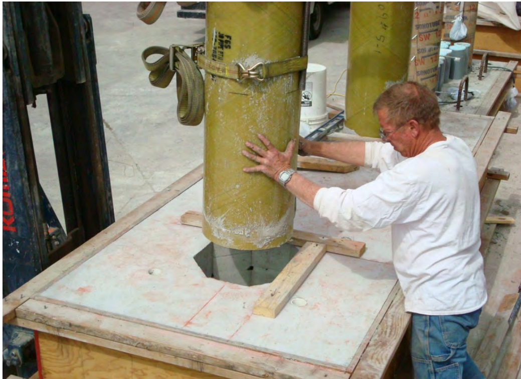
Figure 2.48 Precast concrete-filled FRP tube column at UNR
