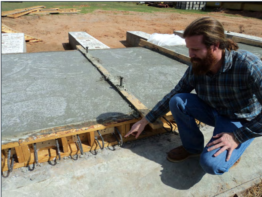
Figure 2.12 Full-depth precast deck panel connection
