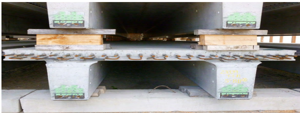
Figure 2.53 NEXT double-T girder used in Massachusetts
