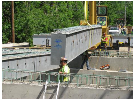
The hybrid-composite beam uses a tested technology to make structures lightweight, strong, and corrosion resistant.
