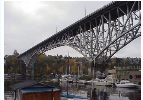
The Aurora Avenue Bridge in Seattle was seismically retrofitted with base isolation bearings. (Image courtesy of WSDOT)
