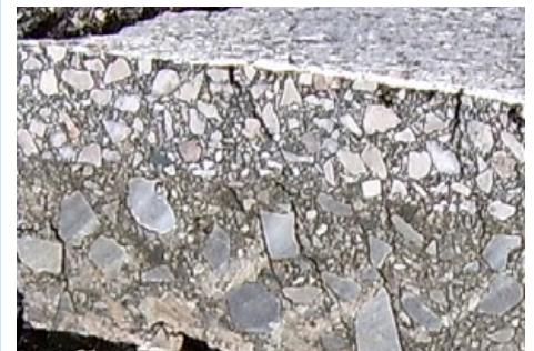
The MEPDG software helps designers select appropriate pavement layer thicknesses for specific site conditions.
