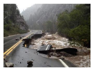
Figure 57. US 34 2013 Flood Damage
