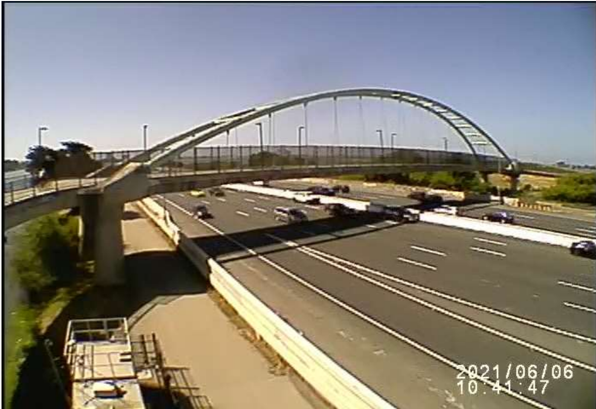
Figure 23. Wiltec traffic counting view on I-80 east-bound (looking south).
