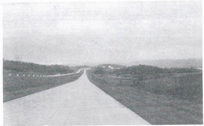
a. View looking toward array 1
