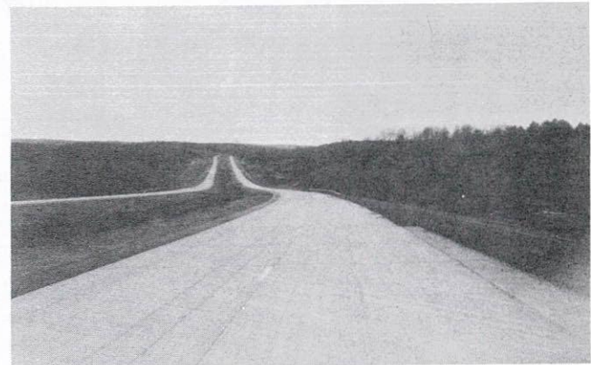
b. View looking toward array 2
