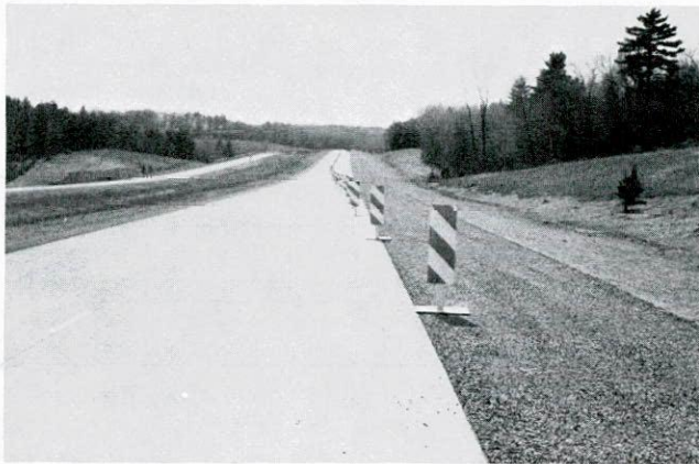
a. 12" x 36" panels at array site 2
