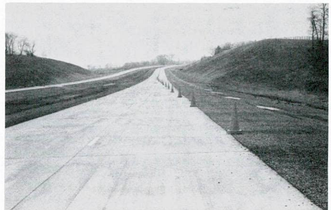
b. 36" cones at array site 1
