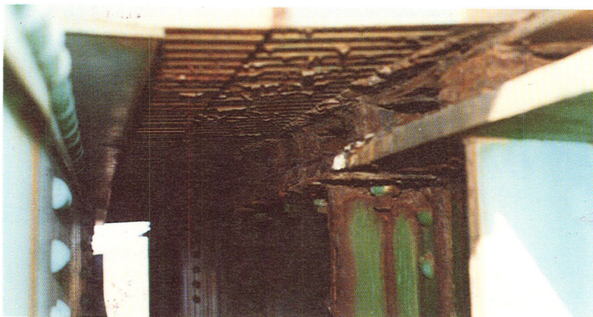
Figure 55(c). Photograph 1 shows typical condition of top flange and web of end floor beams beneath expansion dams. (See also cursory reports—Figures 55a, 55b)
