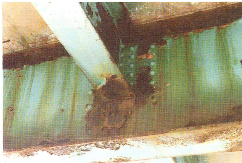
Figure 57(l). Photograph 7 shows typical area of deterioration of floorbeams, top flange and web at stringer connections. (See also detailed reports—Figures 57a through 57e)
