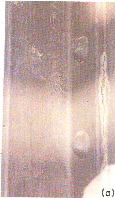
Figure 4. Photographs illustrating the effects of environmental exposure on corrosion. Opposite sides are shown of the same vertical member at the same level. The angle in (b) is on the windward side of the member, exposed to the prevailing wind carrying salt mist from the ocean. The angle in (a) is on the leeward side of the member, protected from the wind.
