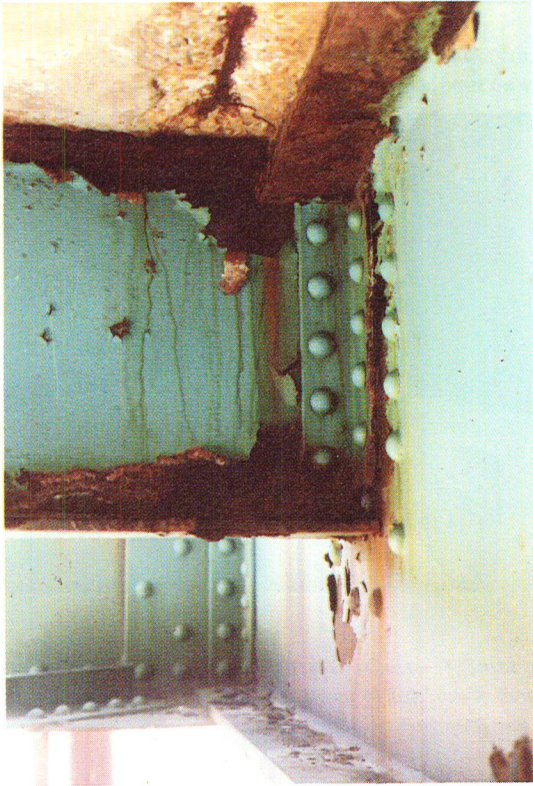
Figure 56(g). Photograph 3 shows typical areas of section loss to stringer flanges and web. (See also general reports—Figures 56a, 56b, 56c)
