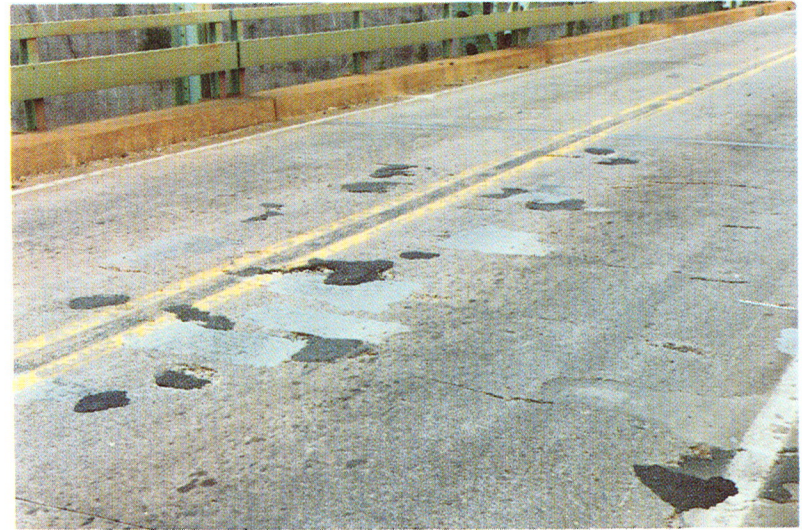
Figure 57(f). Photograph 1 shows typical patched, cracked condition of concrete deck on approaches, which allows leakage. (See also detailed reports—Figures 57a through 57e)
