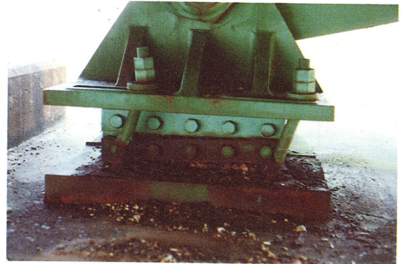
Figure 57(k). Photograph 6 shows typical condition of expansion bearings. Many bolts have bent or sheared off. Note the extent of corrosion in the roller nest. (See also detailed reports—Figures 57a through 57e)
