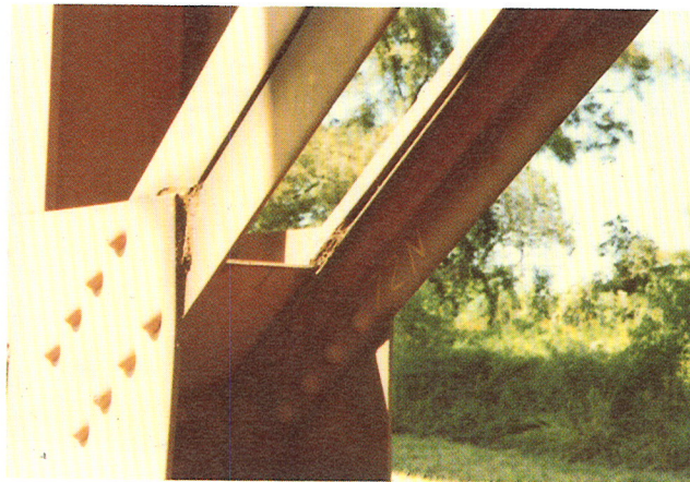
Figure 7. Photograph shows crevice corrosion between back to back angles and gusset plate.
