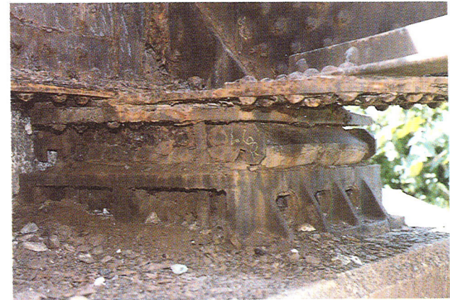
Figure 83. Photograph shows frozen bearings.
