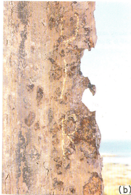
Figure 4. Photographs illustrating the effects of environmental exposure on corrosion. Opposite sides are shown of the same vertical member at the same level. The angle in (b) is on the windward side of the member, exposed to the prevailing wind carrying salt mist from the ocean. The angle in (a) is on the leeward side of the member, protected from the wind.
