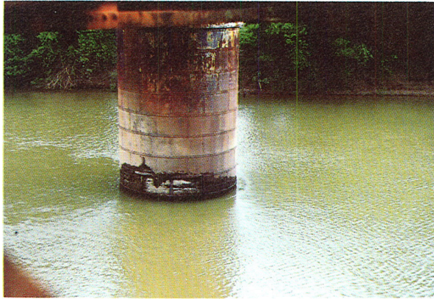
Figure 15. Photograph shows potential erosion corrosion location of a steel-encased pier in a river carrying abrasive particles.
