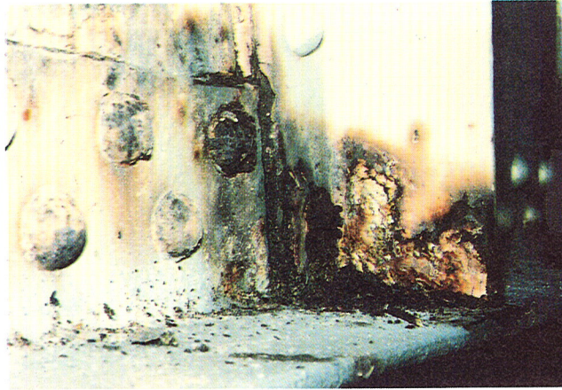
Figure 10. Photograph shows corrosion due to deposit attack at stiffener-to-flange connection. Debris accumulation was removed for photograph.
