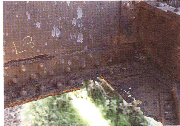
Figure 81. Photographs show flange losses.
