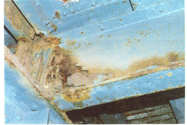
Figure 50(c). Photograph shows progression of deterioration—rating 4.
