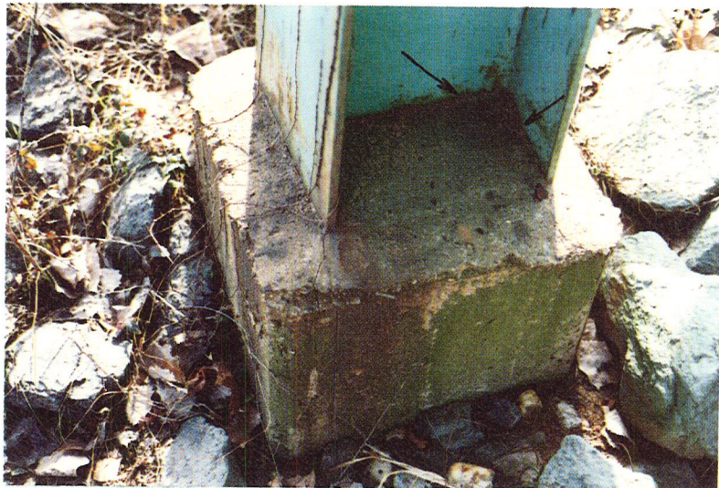
Figure 57(i). Photograph 4 shows typical area of metalwork deterioration at H-pile encasements. Crack in concrete from flange of H-pile is from expansion of deteriorating flange metalwork at interface with the concrete. (See also detailed reports—Figures 57a through 57e)
