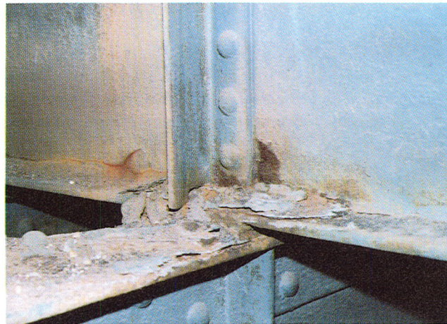
Figure 48. Photograph shows stringer with corrosion and debris accumulation.
