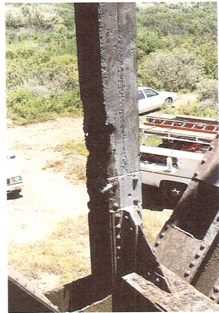
Figure 80. Photographs show truss bridge losses.
