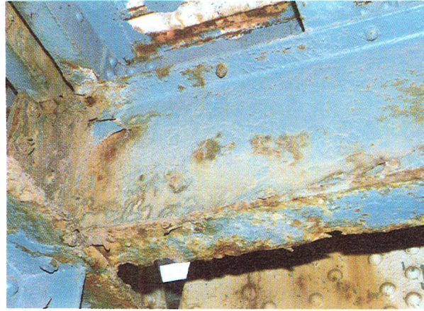
Figure 50(b). Photograph shows progression of deterioration—rating 5.
