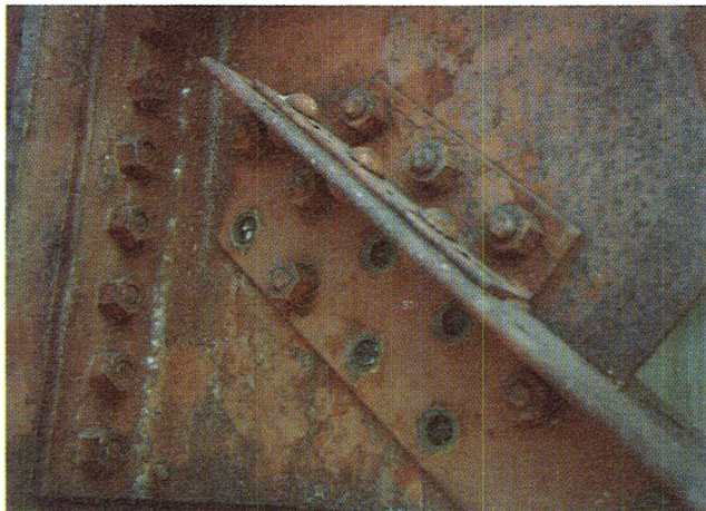
Figure 18. Photograph shows corrosion cracking of bolts in industrial environment.
