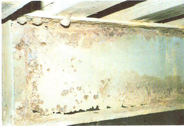
Figure 50(d). Photograph shows deterioration of web at support—rating 1.
