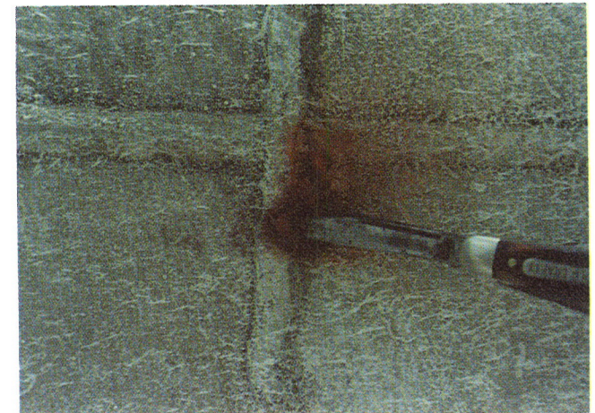
Figure 14. Photograph shows weld decay.
