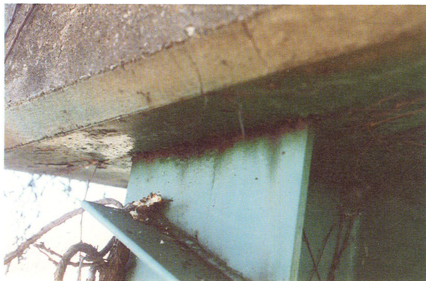
Figure 56(f). Photograph 2 shows typical area of deteriorating metalwork at bottom of bent cap concrete. (See also general reports—Figures 56a, 56b, 56c)
