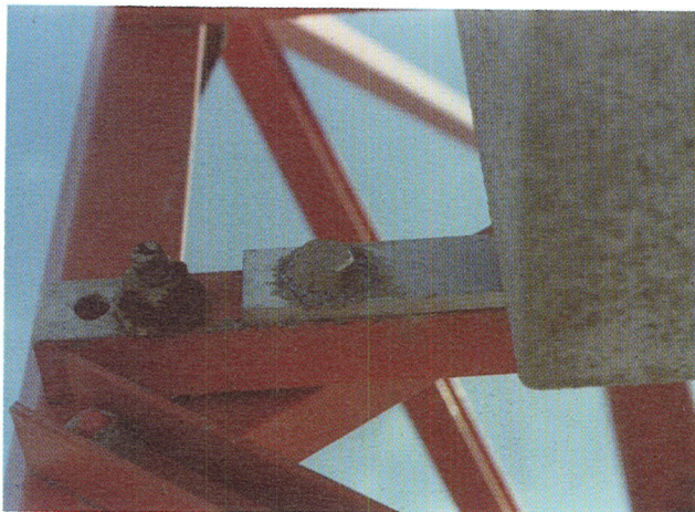
Figure 6. Photograph shows galvanic corrosion—aluminum bracket with carbon steel bolt.
