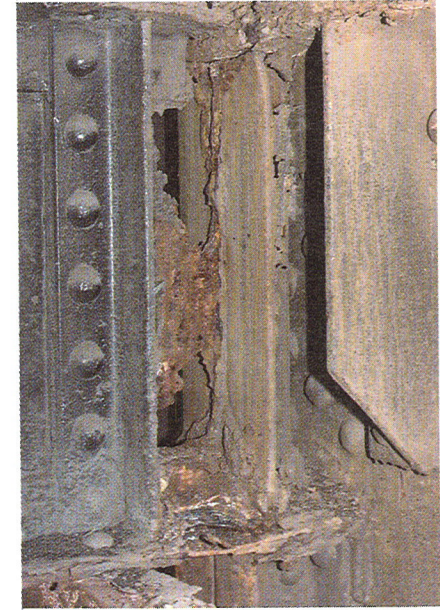
Figure 82. Photograph shows web losses.
