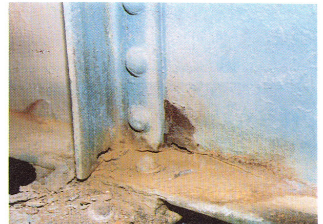
Figure 49. Photograph shows same stringer after cleaning, revealing crack and hole.
