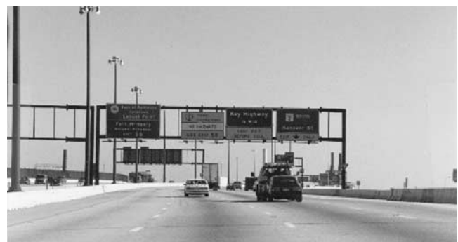
Figure 34. Example of potential DIO situation due to multiple sign panels at one location.
