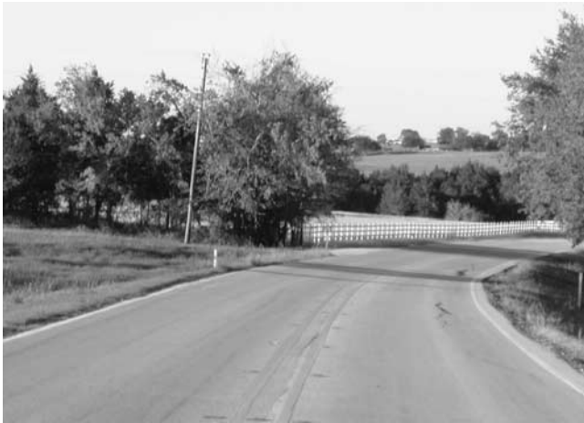
Figure D-1. Case Study A roadway.
