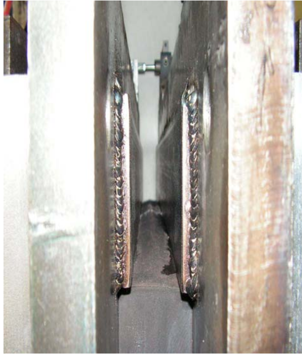
Figure C-6 Bearing Support Plate Improvements
