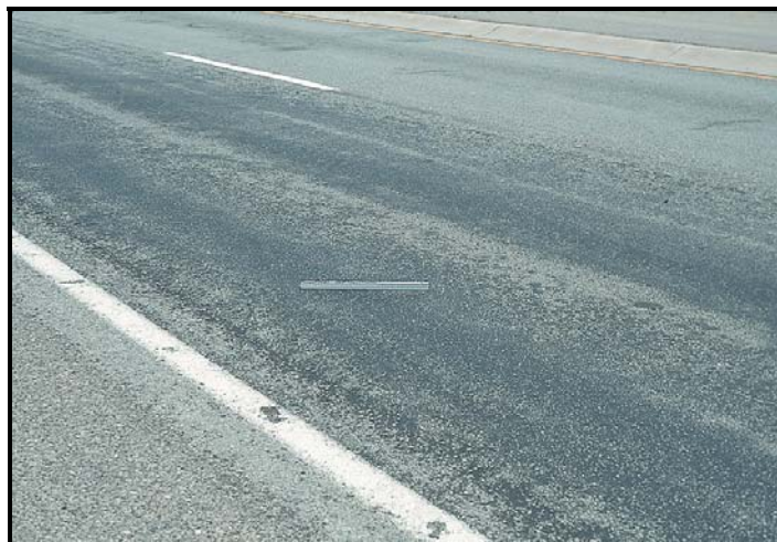
FIGURE B12 Loss of texture.
