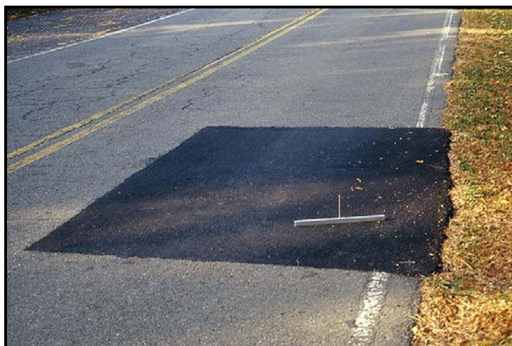
FIGURE B7 Patch/patch deterioration.
