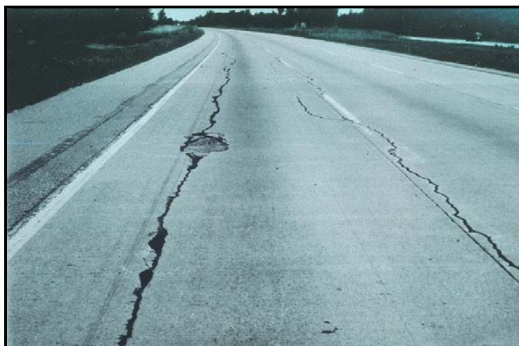
FIGURE B39 Longitudinal cracking.
