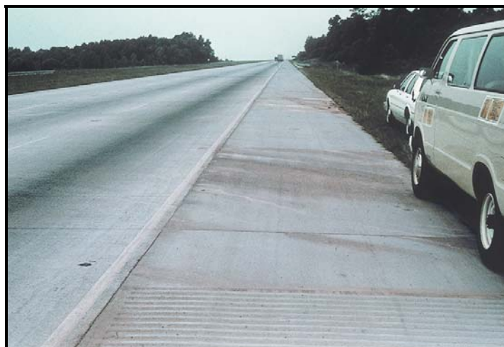
FIGURE B50 Water bleeding and pumping.
