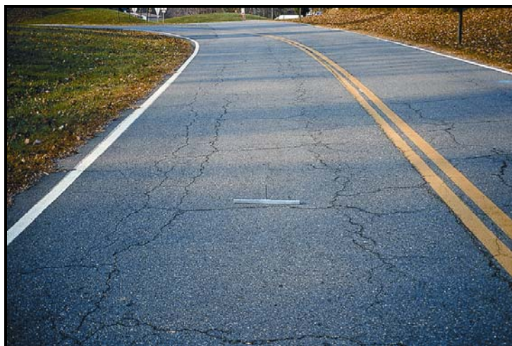
FIGURE B2 Block cracking.
