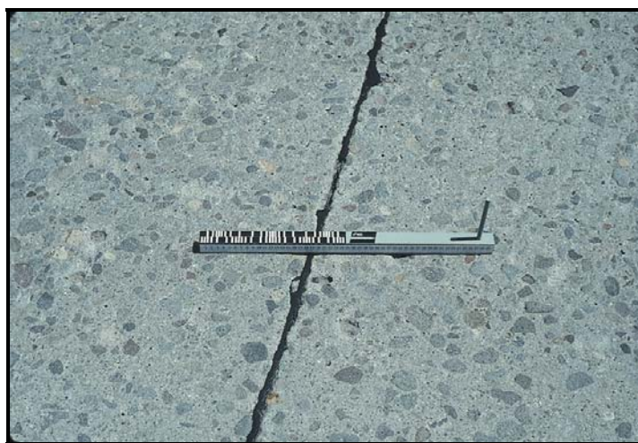
FIGURE B25 Longitudinal joint seal damage.
