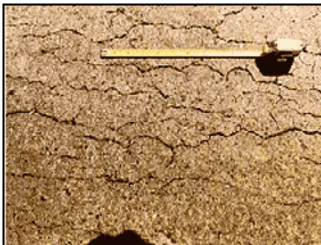
FIGURE B37 Alkali–silica reaction.
