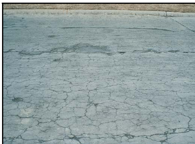
FIGURE B28 Map cracking.
