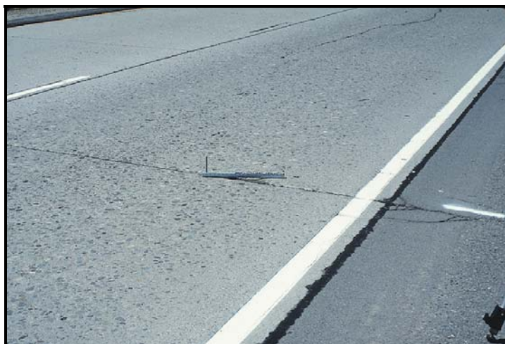
FIGURE B27 Spalling of transverse joints.
