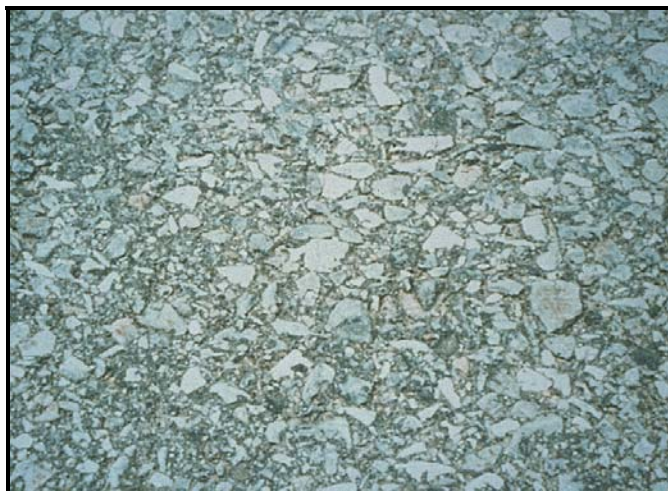
FIGURE B14 Polished aggregate.
