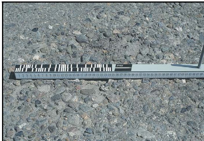
FIGURE B17 Loss of coarse aggregate.
