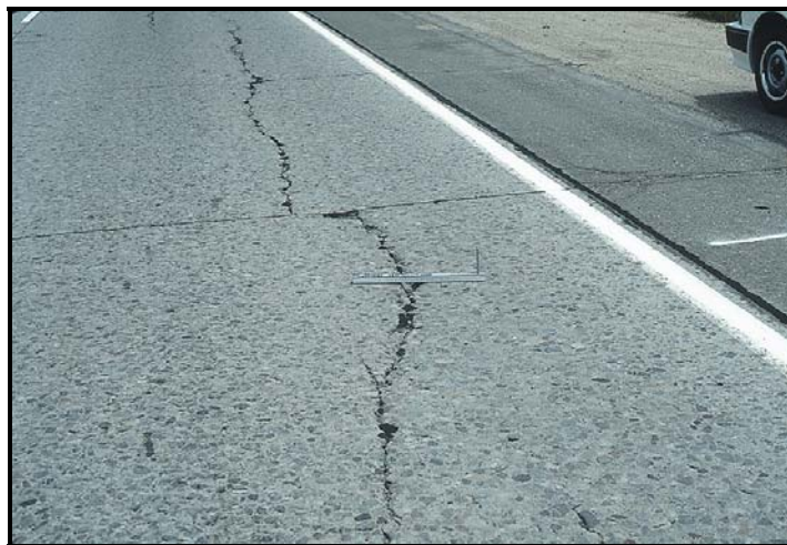
FIGURE B22 Longitudinal cracking.
