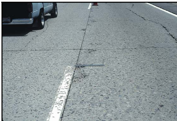
FIGURE B26 Spalling of longitudinal joints.
