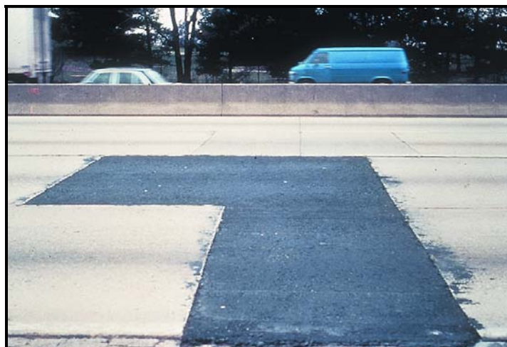
FIGURE B34 Patch/patch deterioration.
