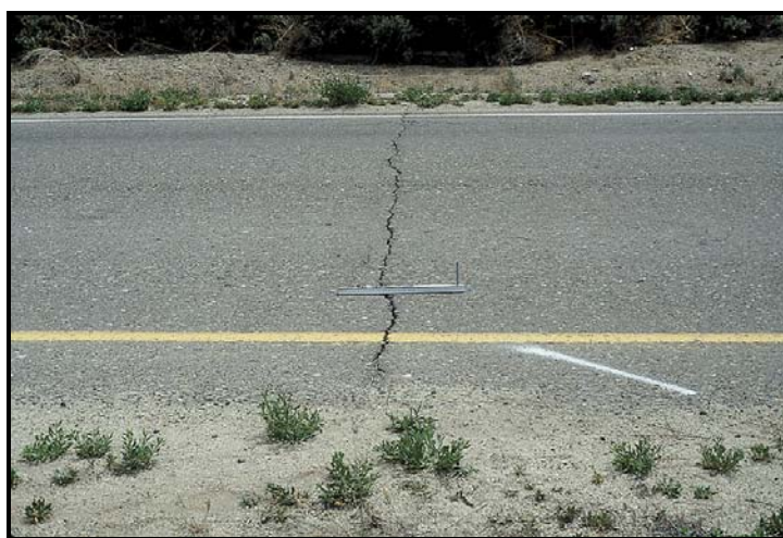
FIGURE B6 Transverse cracking (HMA surfaces).
