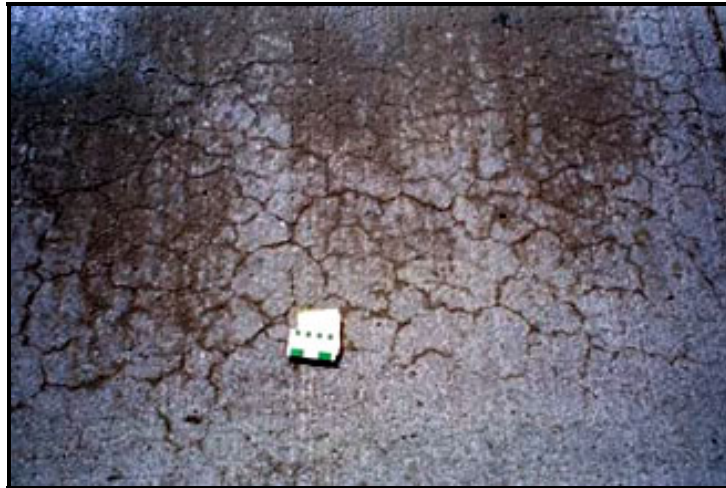
FIGURE B52 Alkali-silica reaction.
