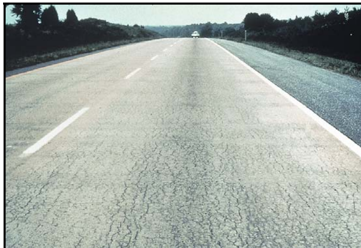
FIGURE B41 Map cracking.
