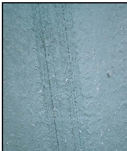
FIGURE B13 Aggregate obscured.
