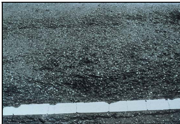
FIGURE B16 Loss of fine and some coarse aggregate.
