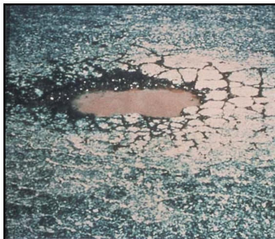
FIGURE B8 Potholes.
