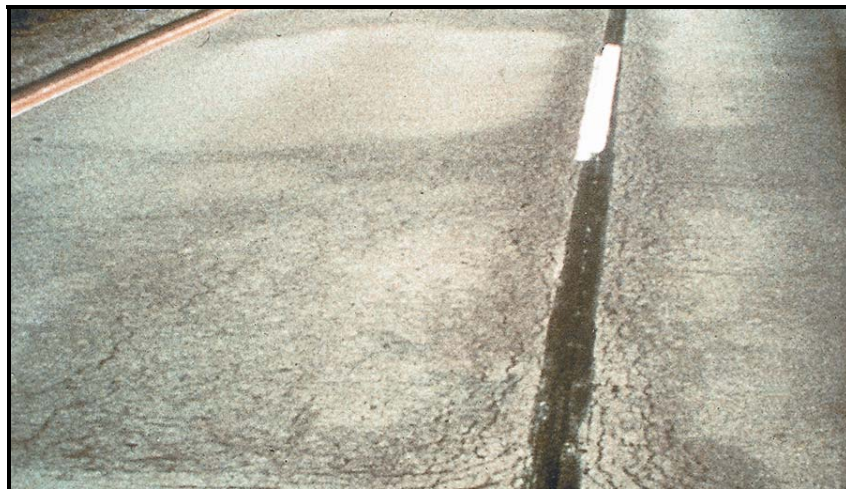
FIGURE B38 Durability cracking (D-cracking).
