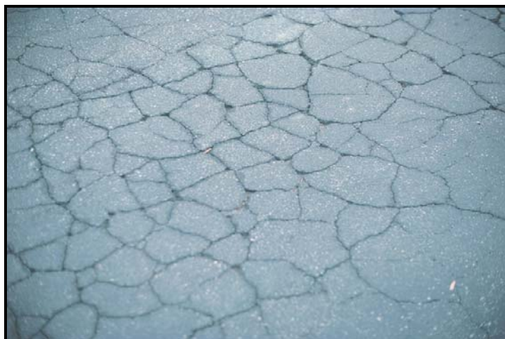
FIGURE B1 Fatigue cracking.
