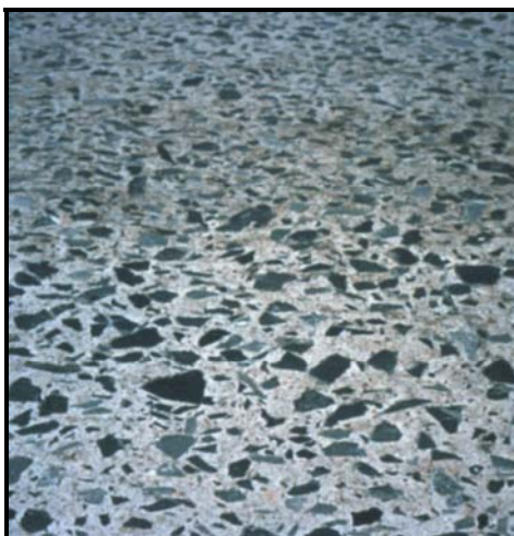
FIGURE B30 Polished aggregate.
