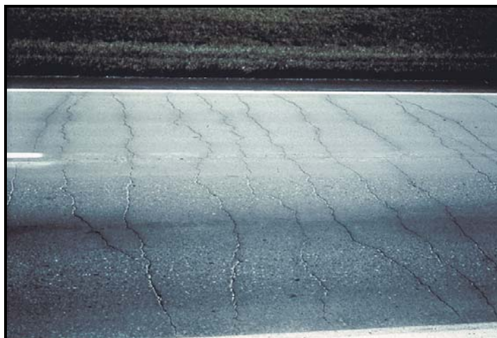
FIGURE B40 Transverse cracking.
