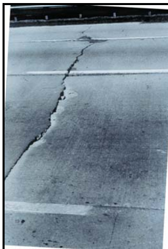
FIGURE B33 Faulting of transverse crack.
