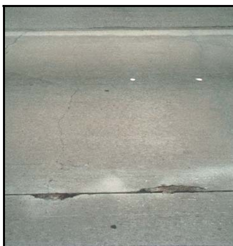
FIGURE B49 Spalling of longitudinal joints.
