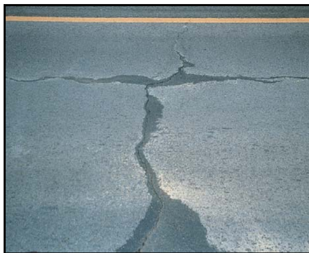
FIGURE B18 Water bleeding and pumping.
