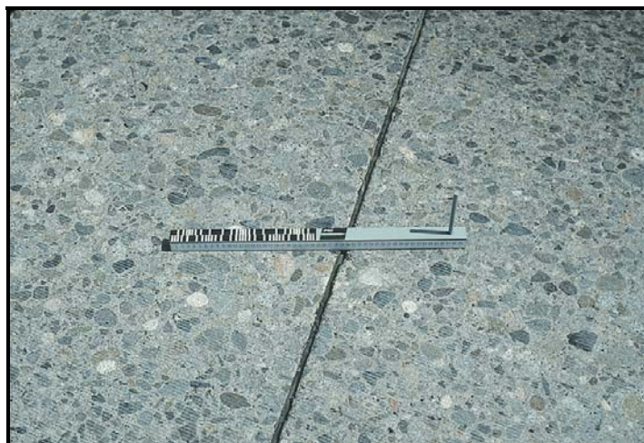
FIGURE B24 Transverse joint seal damage—Low severity.
