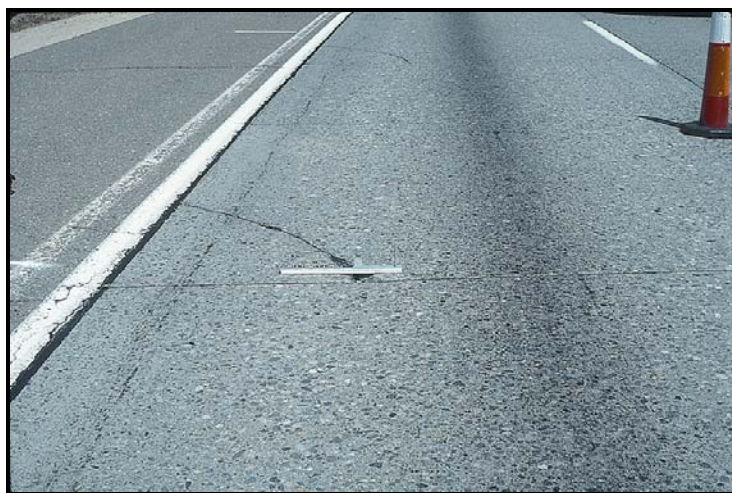
FIGURE B20 Corner breaks.
