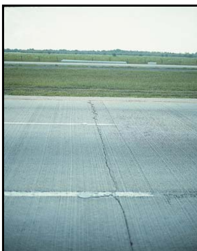
FIGURE B46 Transverse construction joint deterioration.
