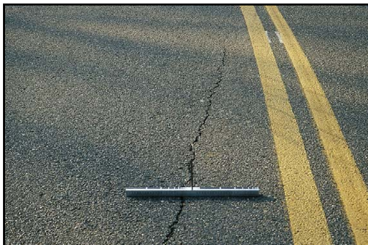
FIGURE B4 Longitudinal cracking.
