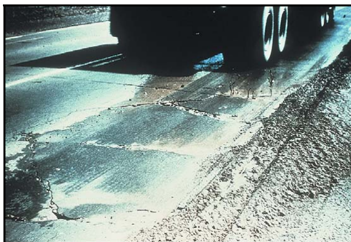
FIGURE B35 Water bleeding and pumping.
