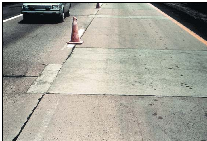
FIGURE B47 Patch/patch deterioration.
