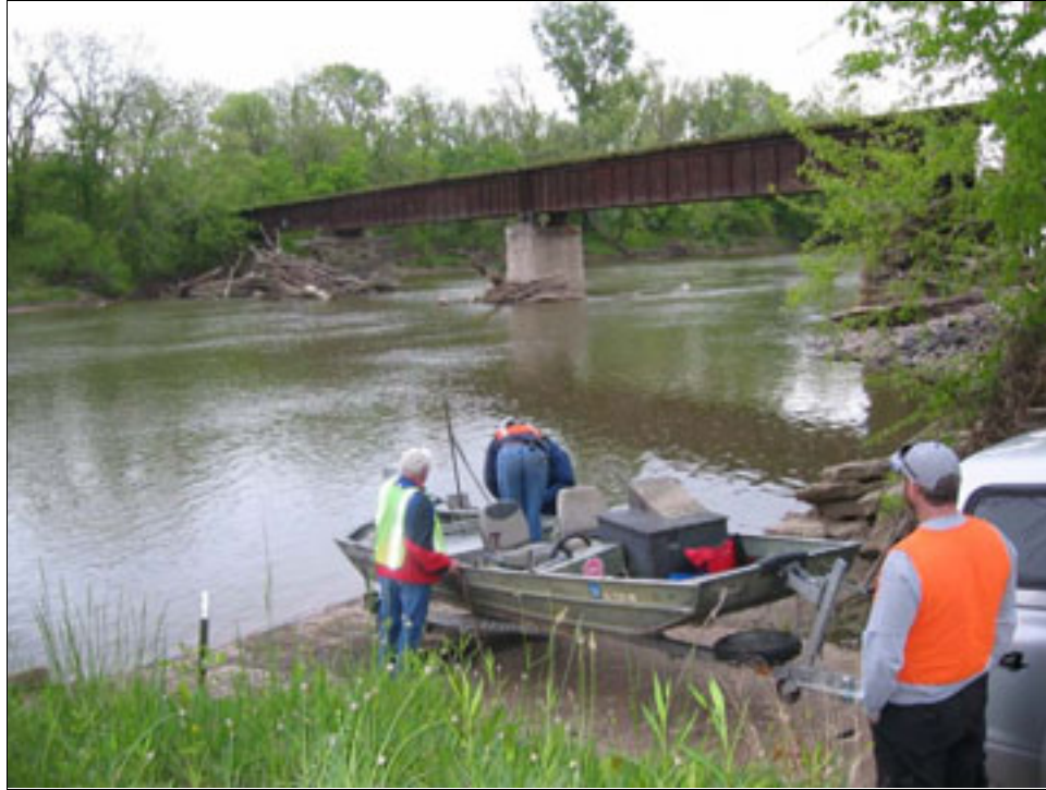
Figure 2.3. Railroad Bridge adjacent to the boat launch.
