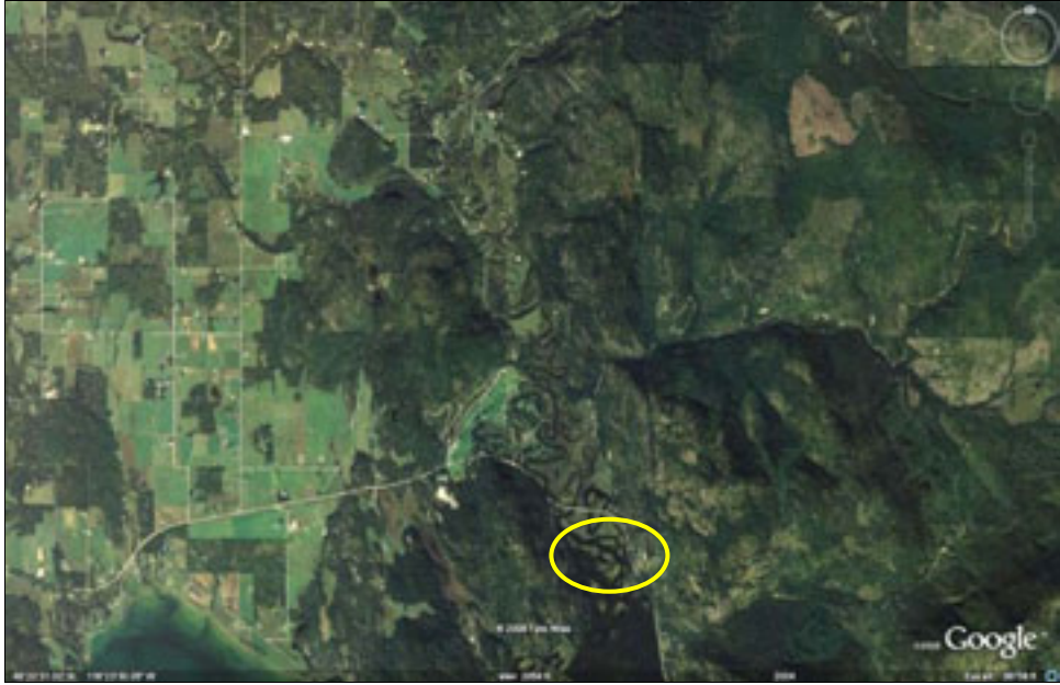
Figure A.2. Aerial view of State Highway 200 over the Pack River.
