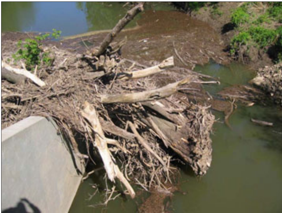
Figure 3.6. Key log on left extension pier.
