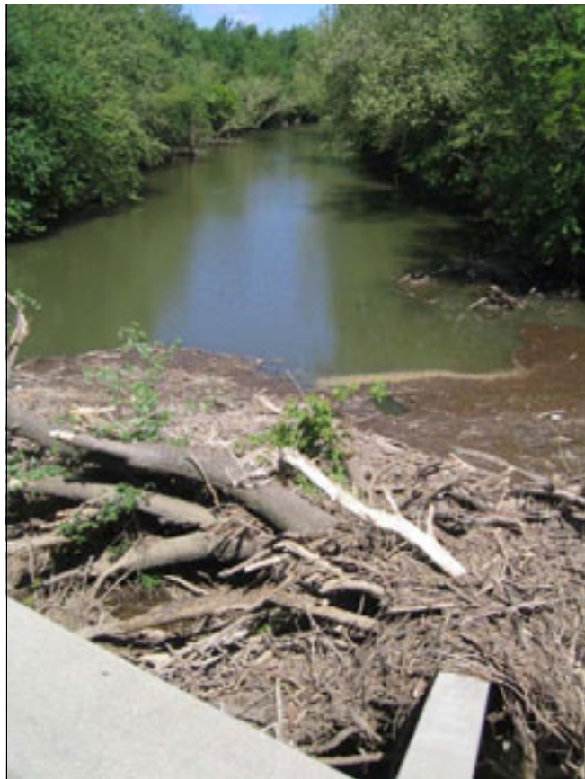
Figure 3.8. Looking upstream from the bridge deck.
