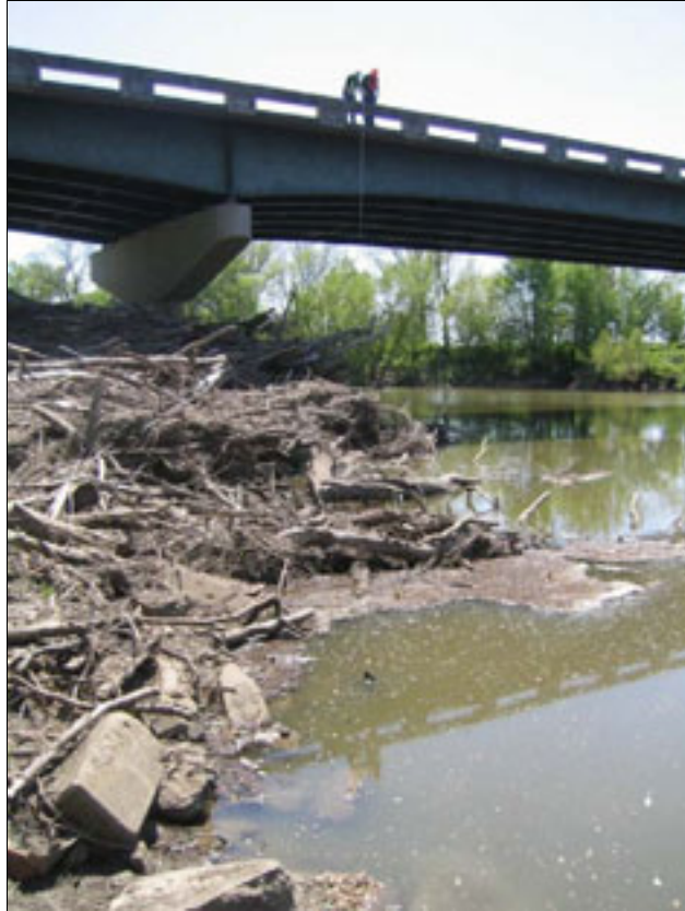
Figure 5.7. Measuring the water surface from the bridge deck.
