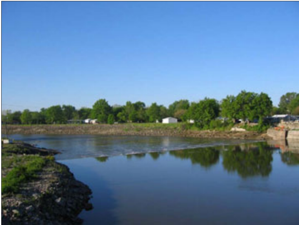
Figure 1.4. Spillway downstream of the bridge.
