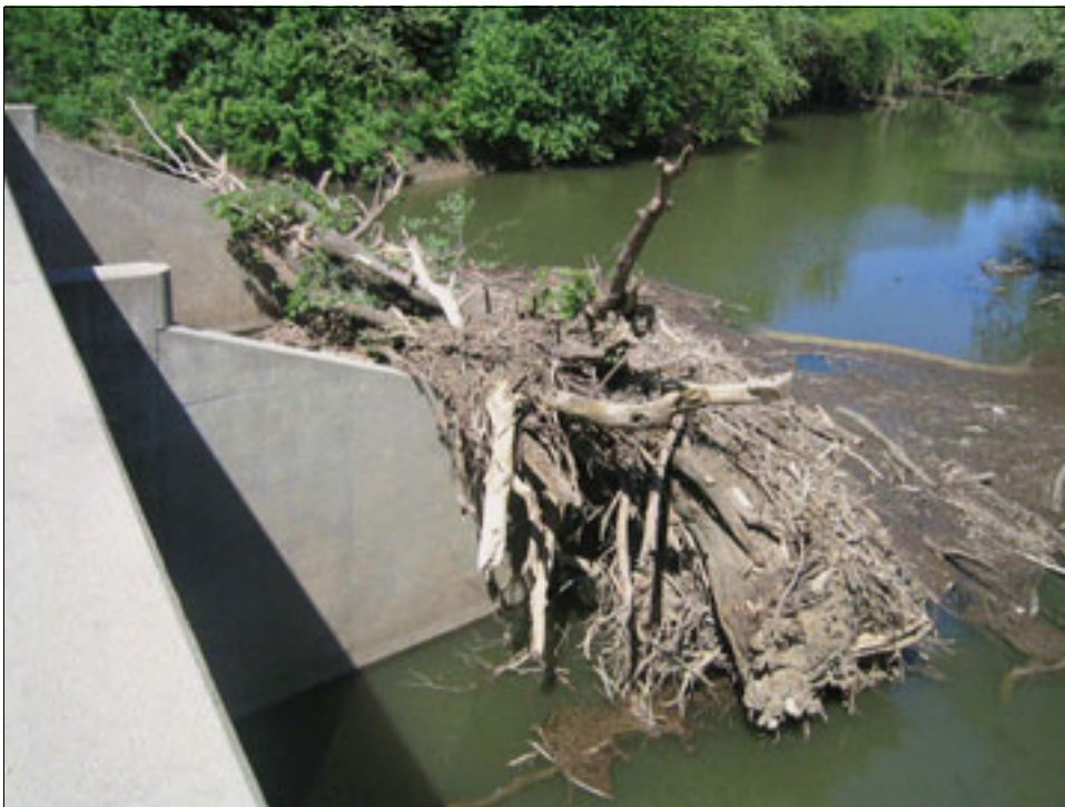
Figure 3.4. Extension walls, skewed to flow.
