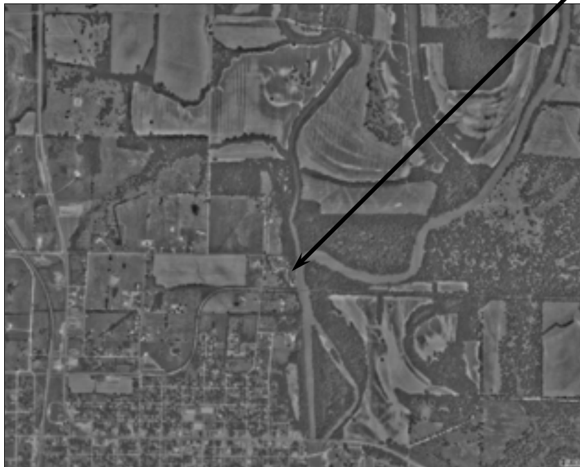
Figure 2.2. Aerial view of Railroad Bridge.
