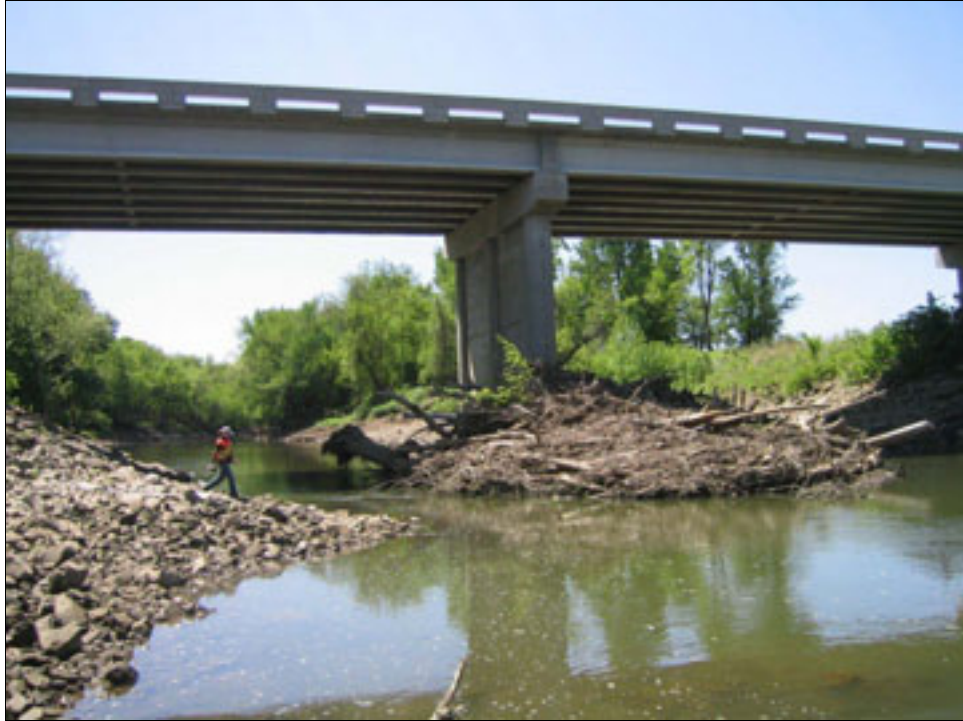
Figure 4.2. Looking downstream toward the bridge.
