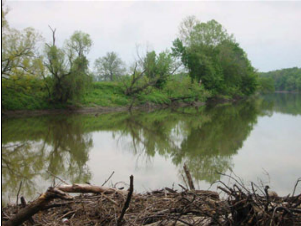
Figure 5.3. Looking upstream from debris pile. Note the eroding banks and trees leaning into the channel.
