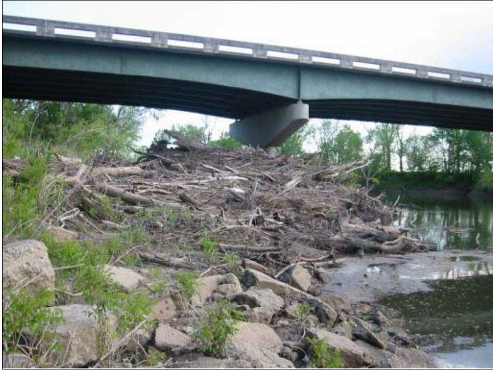
Figure 5.5. Looking downstream at debris pile.
