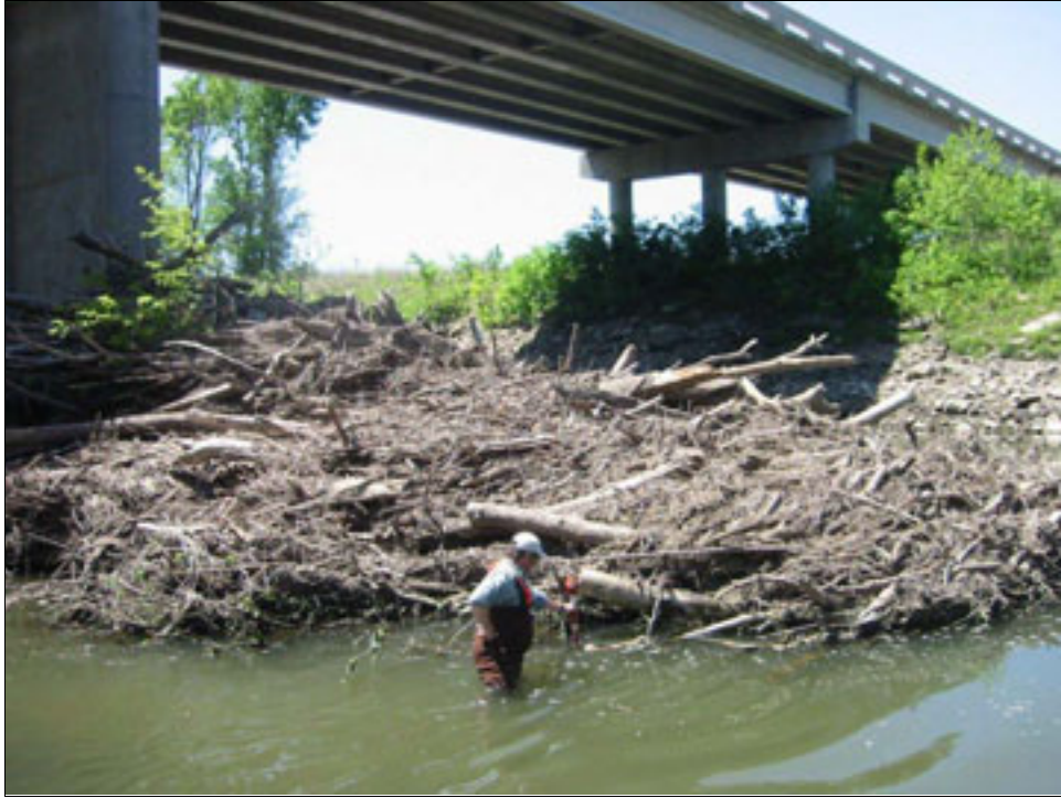
Figure 4.4. Surveying the edge of the debris pile.
