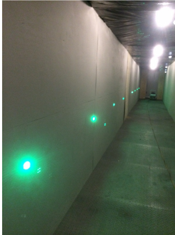
Figure 9. LED path lights in simulated tunnel.
