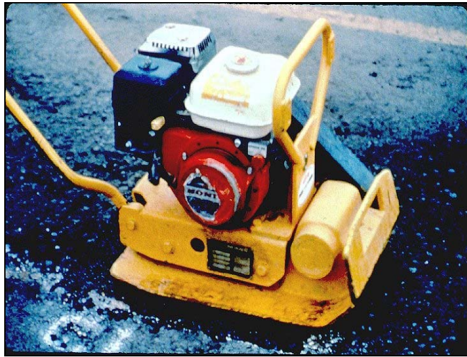
Figure B-2. Vibratory compaction of asphalt patch. 4
