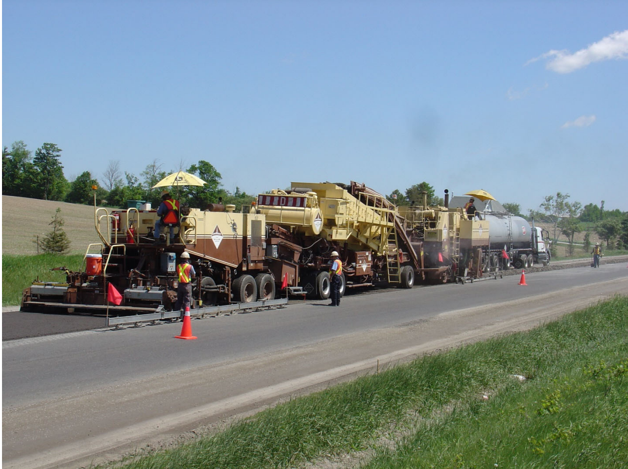
Figure 13 Multi-unit train (courtesy ARRA)
