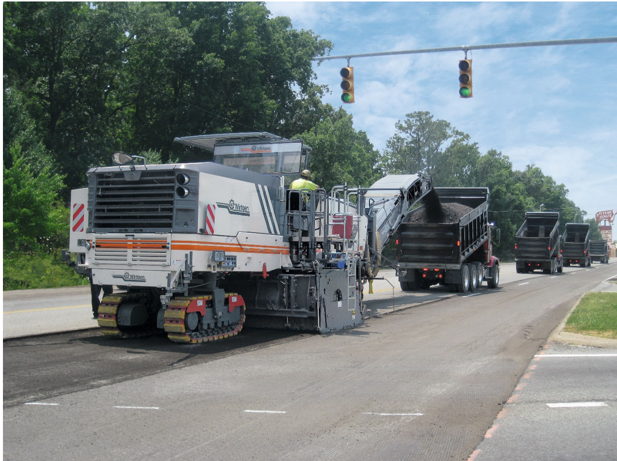
Figure 9 Milling machine depositing RAP into haul trucks. (courtesy ARRA)
