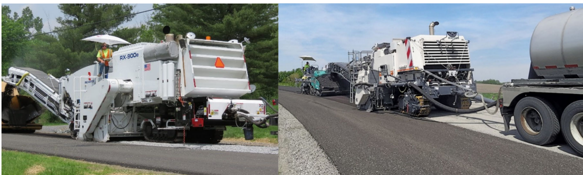
(a) (b) Figure 11 Single unit CIR Trains (courtesy ARRA)
