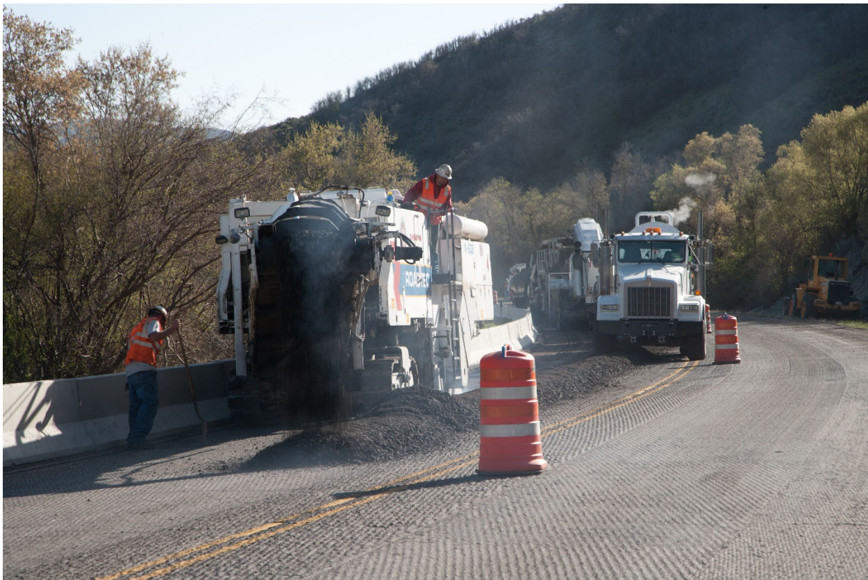
Figure 8 Recycling the shoulder plus full lane width by using a second milling machine. (courtesy ARRA)
