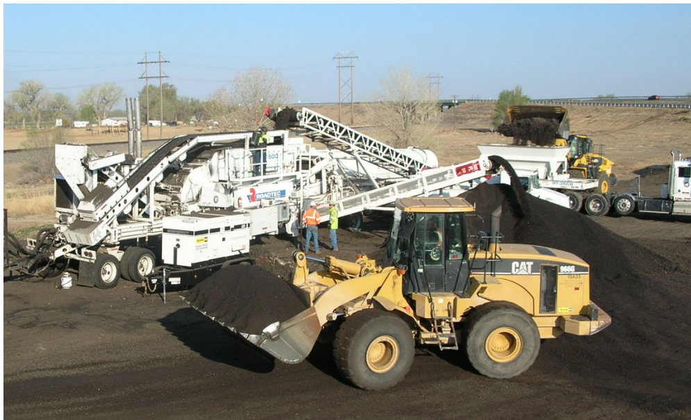
Figure 15 Processing unit from multi-unit train producing CCPR mix (ARRA 2015)
