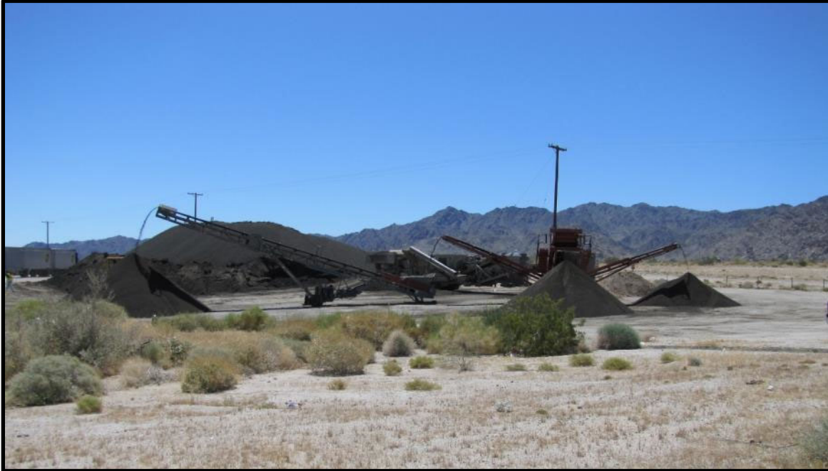
Figure 5 Fractionating RAP (Courtesy ARRA)
