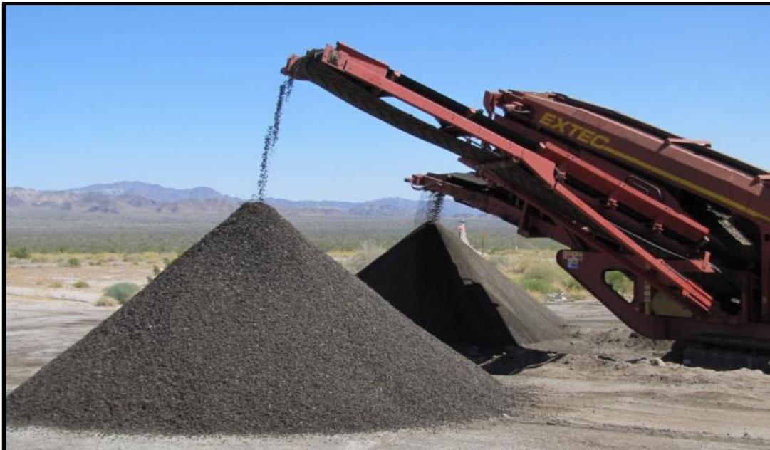
Figure 4 Fractionating RAP (Courtesy ARRA)
