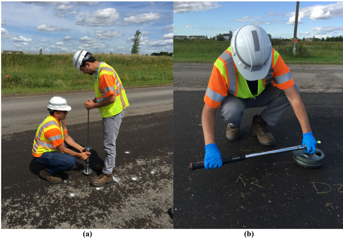
Figure 17. (a) Dynamic Cone Penetrometer weight being used to drive the long-pin shear device into the cold recycled mat while counting the number of blows and (b) torque being applied to the long-pin shear device and recorded.
