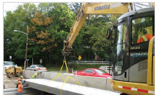
A hybrid-composite beam is lowered into place as a New Jersey bridge takes shape. The NCHRP IDEA Program (Project 20-30) helped put the innovative new bridge beam concept into practice.
