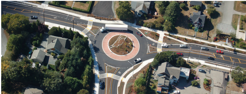
Roundabouts, which help increase safety and reduce congestion, are becoming more common in the United States through the implementation of NCHRP Project 03-65.
