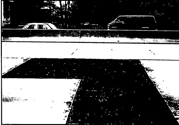
FIGURE 86 JCP 15. Large, Low Severity Asphalt Concrete Patch
