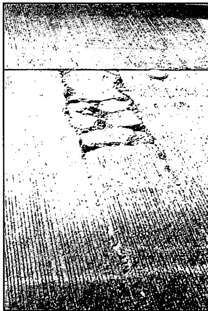
FIGURE 126 CRCP 12. High Severity Punchout
