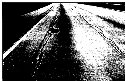
FIGURE 95 CRCP 2. High Severity Longitudinal Cracking
