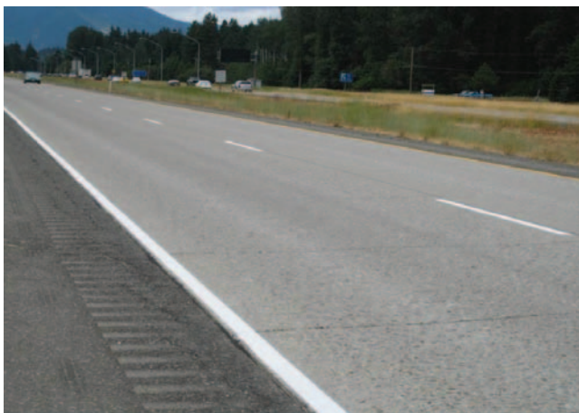
Figure 3: Photo of 35-year-old unbonded PCC overlay on I-90 in Washington
