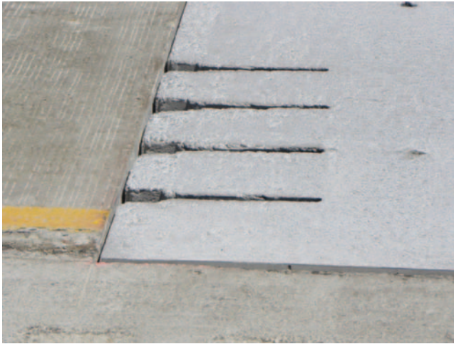
Figure 1: SHRP 2 narrow-mouth slot system installed by Illinois Tollway Authority
