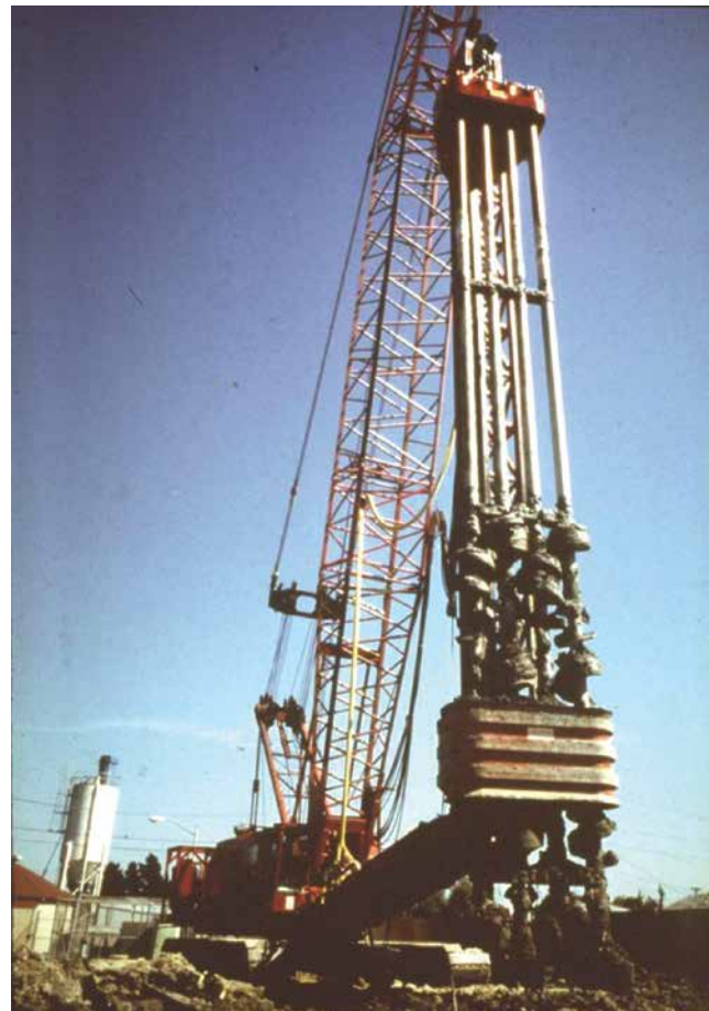
Deep soil mixing
