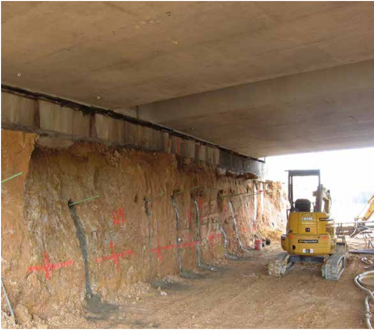
Roadway widening at abutment constrained by limited headroom and existing piles
