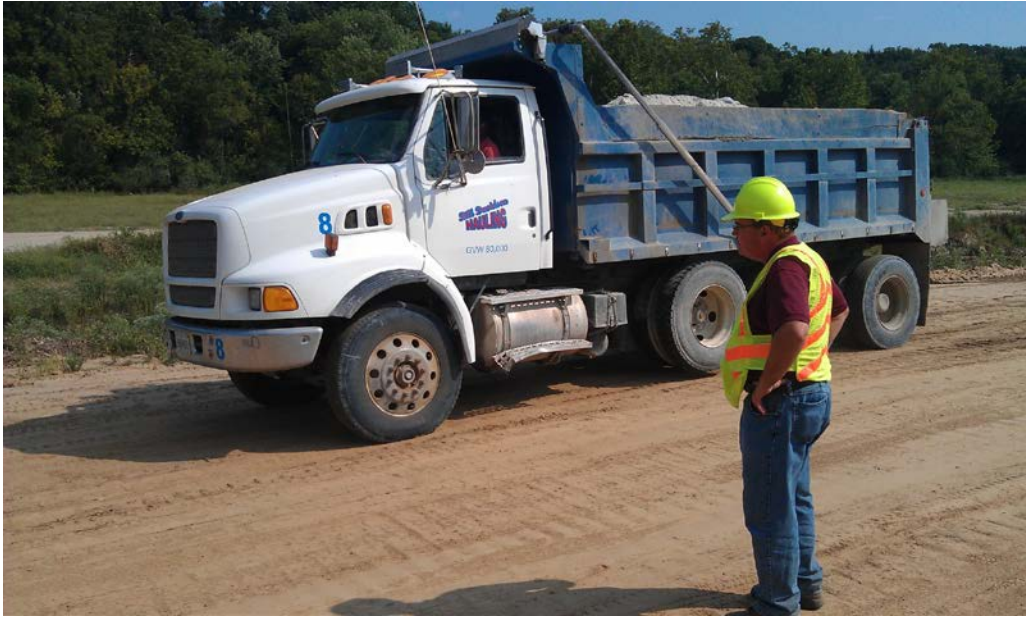
Figure 616: Loaded dump truck for traditional proof roll to determine rut depth
