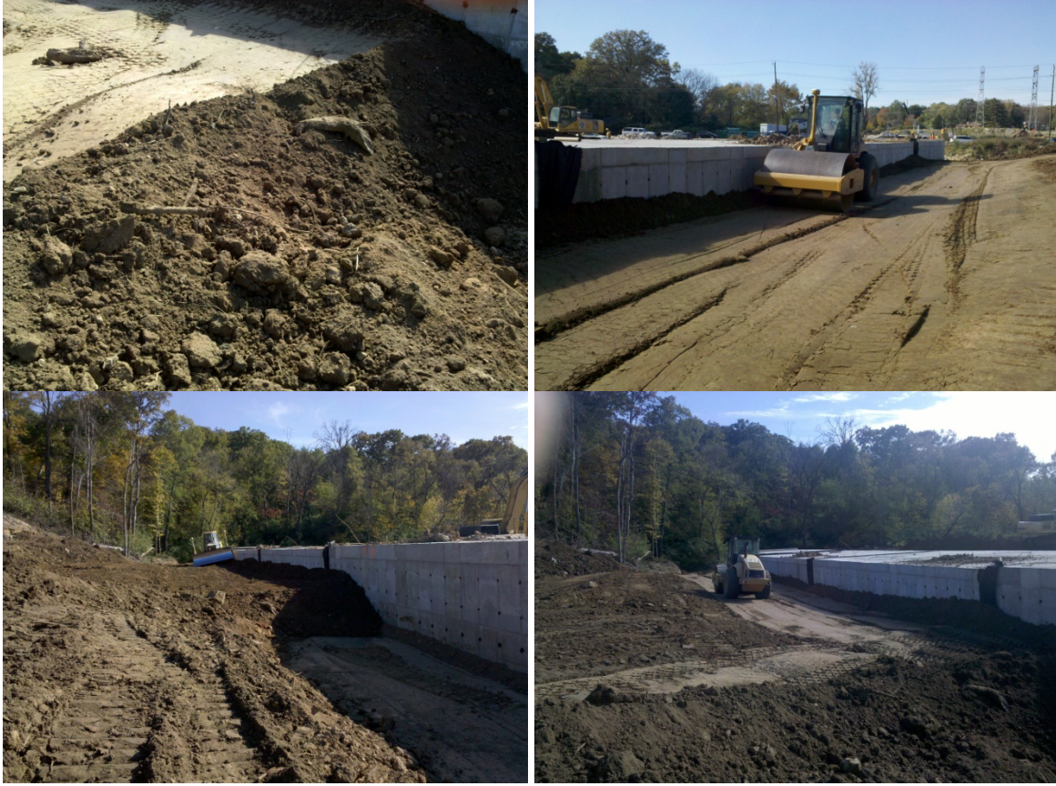
Figure 17: Test Area #3 at double box culvert at south end of project
