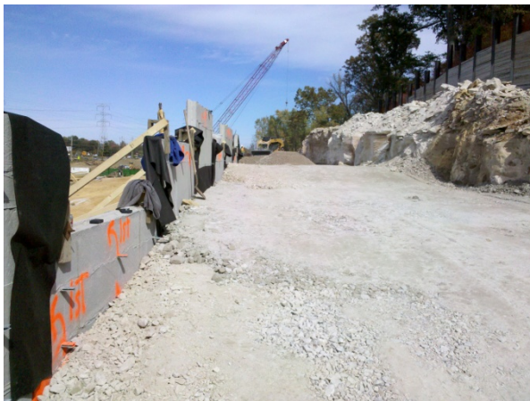
Figure 35: Test area #5 Two-tiered retaining wall backfill
