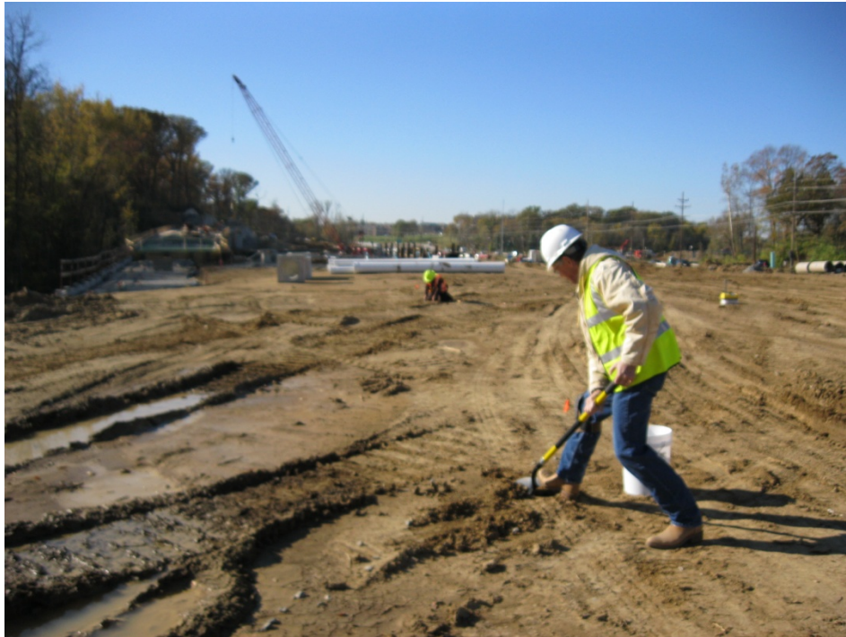
Figure 48: Test area #7 Subgrade proof mapping metzer4
