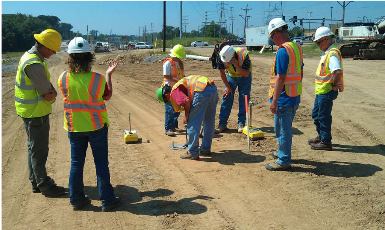
Figure 83: QA/QC operations to conduct nuclear density tests
