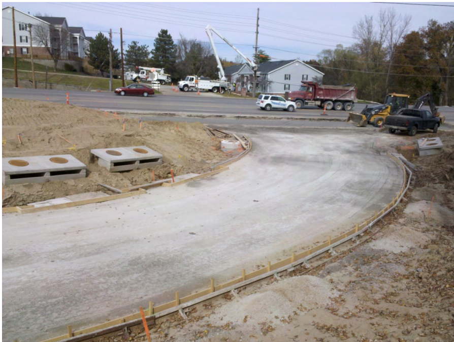
Figure 42: Tets Area #6 at Tuador frontage road compaction on aggrgeate base
