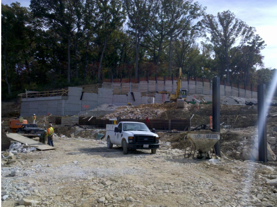
Figure 36: Test area #5 Multiple tiered MSE wall construction
