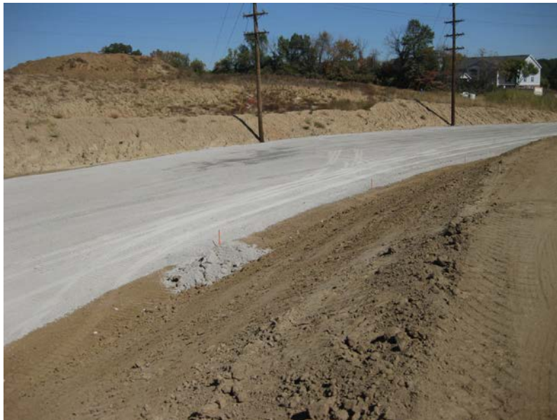
Figure 10: Test area #2 on north end temporary detour road on aggregate base
