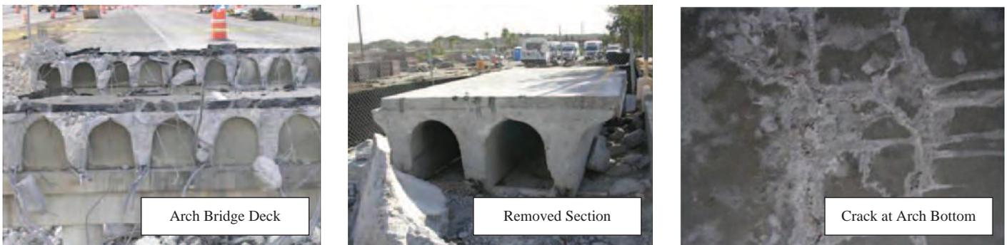
Figure 5.19. Bridge with arch deck.
