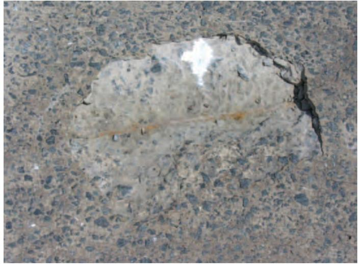
**Figure 2.1. Deck deterioration.**
