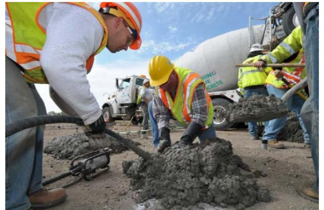
**Figure H.26.** Concrete was placed around the sensors to protect the sensor before the passing of the paver.
