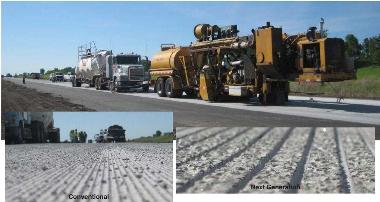
**Figure F.37.** The initial learning portion of the EAC texture was diamond ground using conventional grinding in the passing lane and next-generation grinding in the driving lane.
