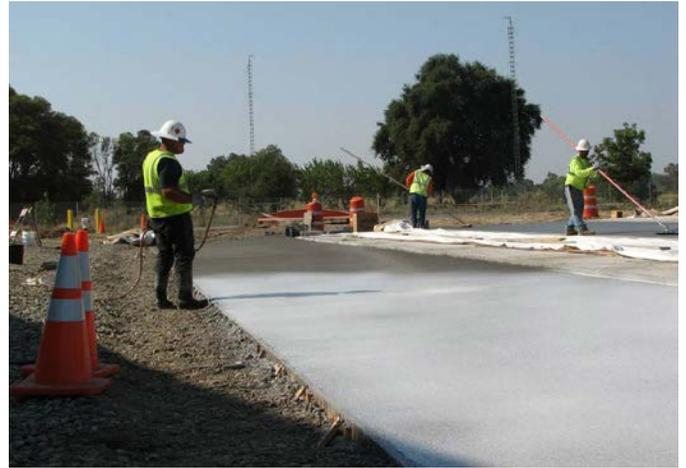
**Figure G.31. Applying the first coat of curing compound on Lane D.**
