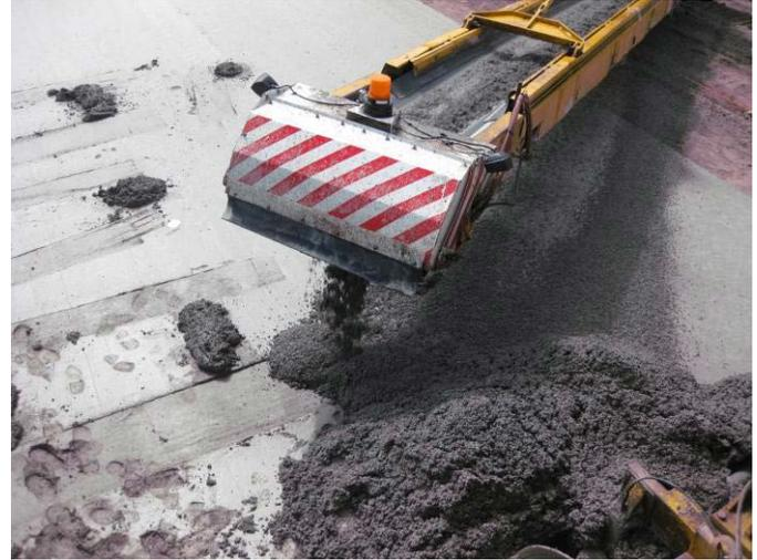
**Figure F.33. Placement of the upper PCC mix on the lower PCC layer.**
