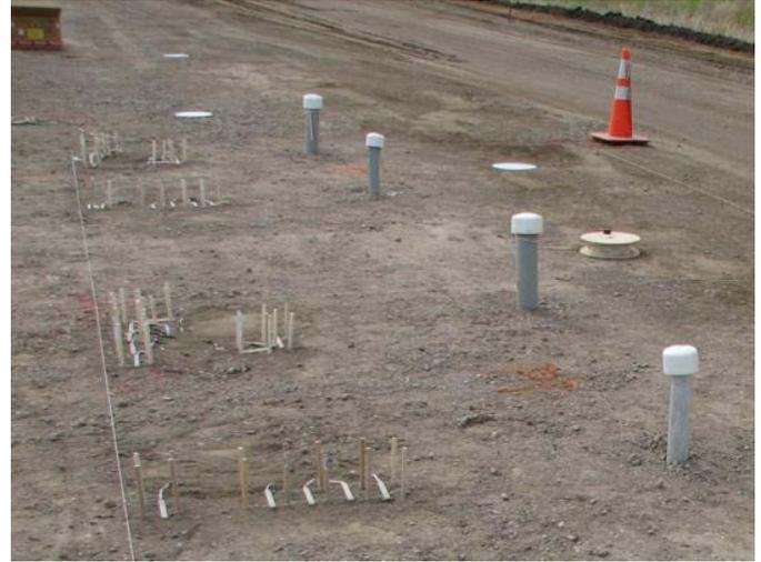
**Figure H.16. Example of the vertical PVC pipe where the dynamic strain gauges were stored until after the pass of the first paver for Cells 71 and 72.**
