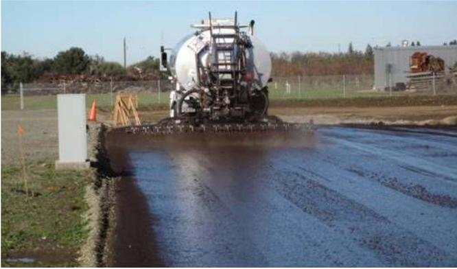
Figure G.13. Completed application of prime coat.
