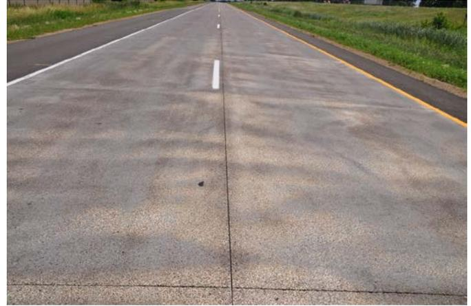
**Figure V.21. Marbled EAC surface resulting from saturation during construction.**
