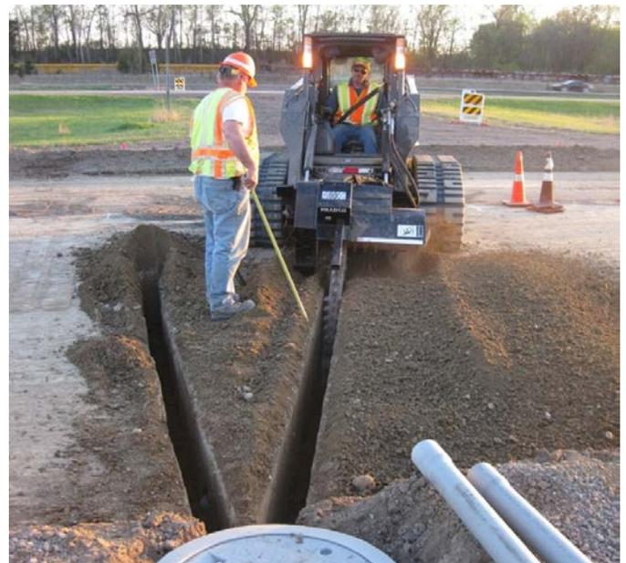
**Figure F.14. Installing conduits to carry and protect the instrumentation cables.**
