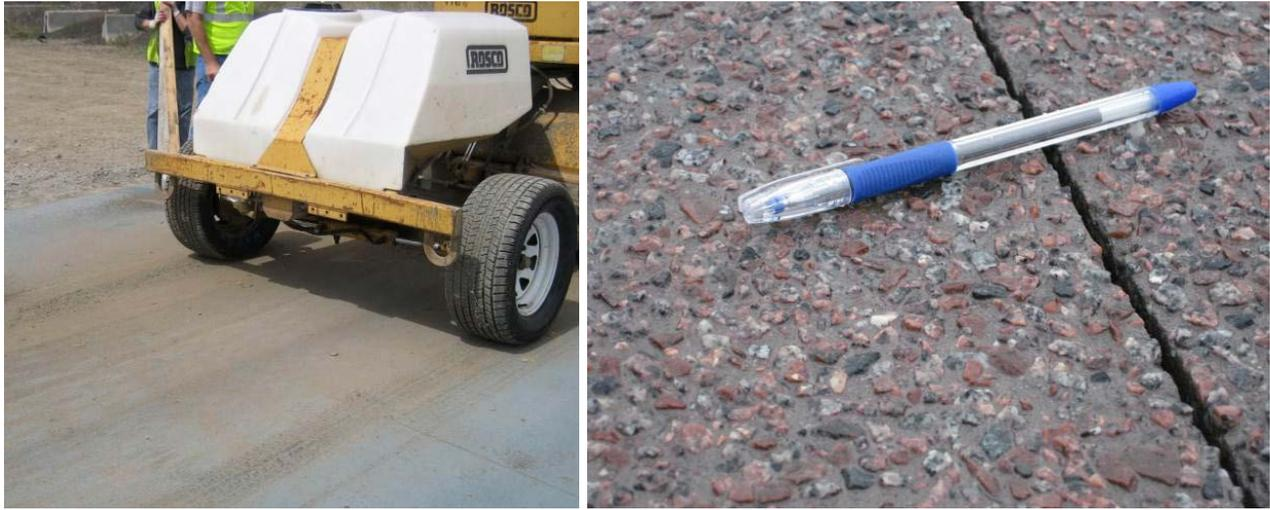
**Figure F.35. Surface after first pass with brush (left); finished EAC surface after wash (right).**
