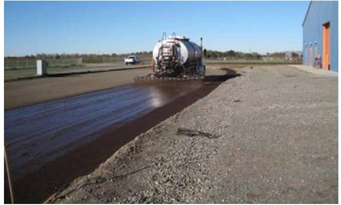
**Figure G.11. Initial pass of prime coat application on eastern side of track.**
