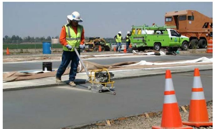
**Figure G.32. Early entry saw cutting joints on Lane D.**
