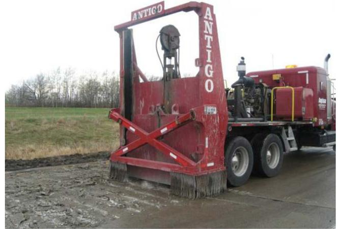
**Figure F.4. Guillotine crusher breaking existing concrete for recycling into the PCC layer of the HMA/PCC composite pavement.**
