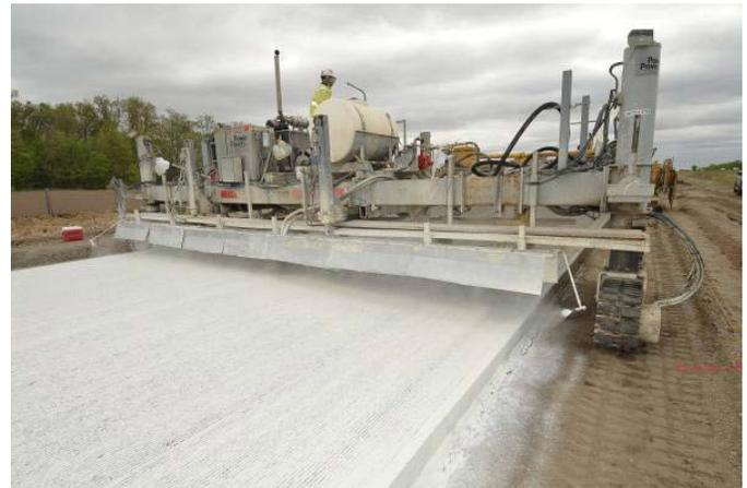
**Figure F.23. Applying curing compound to the surface of the PCC to control surface drying of the PCC and minimize early-age distresses.**
