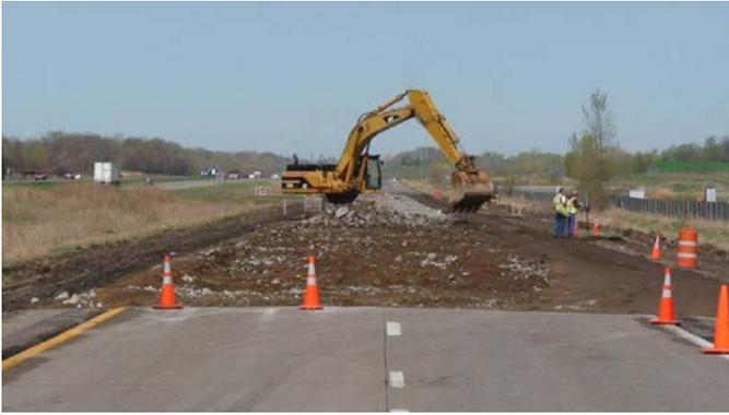
**Figure F.6. Removal of existing concrete pavement for recycling.**
