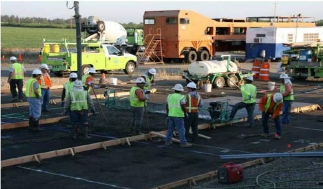
**Figure G.29. Motorized screed on Lane C, Day 1 of PCC paving.**
