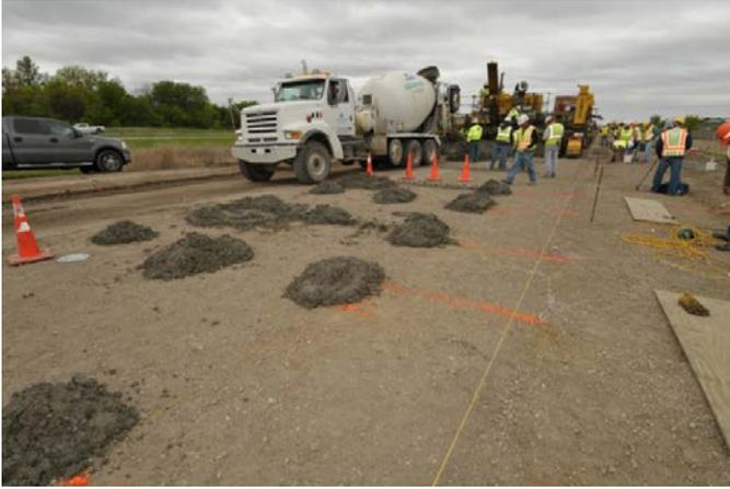
**Figure H.27.** Mounds of concrete placed around the sensors before the passing of the paver.
