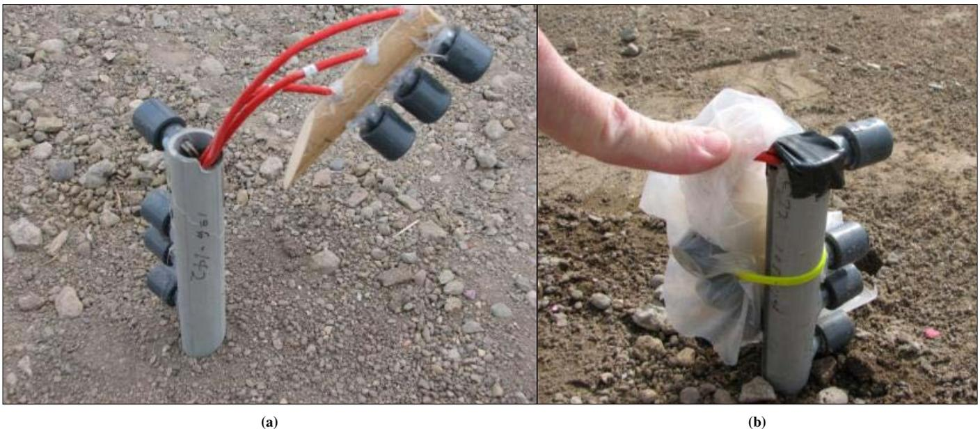
**Figure H.9. Concrete relative humidity sensors installed in Cells 71 and 72. (a) Sensors to be installed in the upper and lower PCC layers and (b) installation just before the passing of the first paver.**
