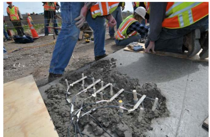
**Figure H.17. Example of the installation of the dynamic strain gauges in the upper concrete layer for Cells 71 and 72.**
