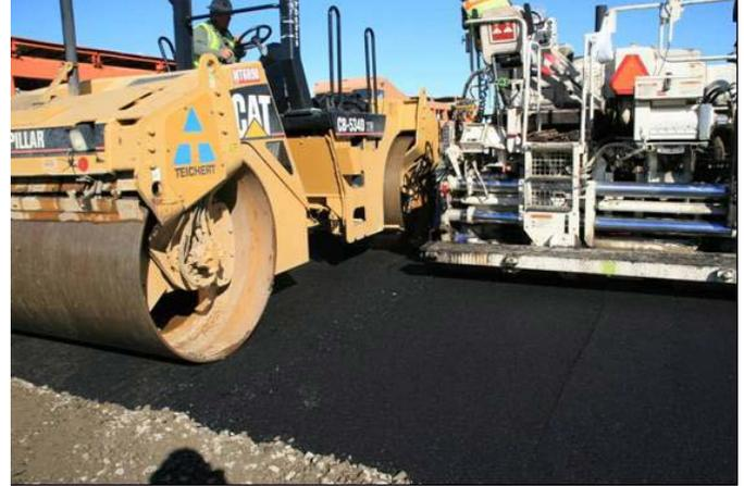
**Figure G.40. Compaction and placement of RHMA-G in Lanes C and D.**
