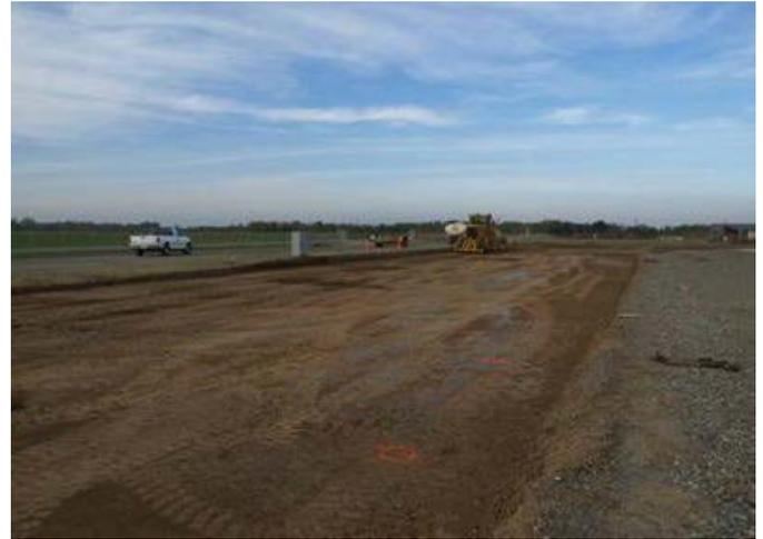
**Figure G.8. Initial leveling and rolling of test track subgrade.**
