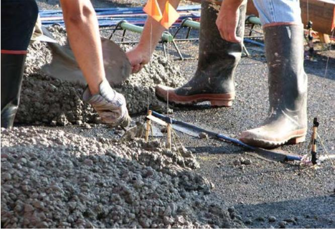
**Figure G.28. Hand packing concrete around instrumentation.**
