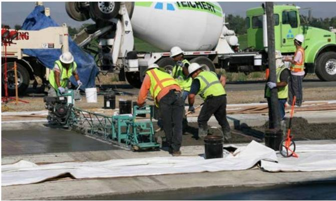
**Figure G.33. Burlene in place on Lanes A and C, while Lane B is paved on Day 2 (Burlene has been temporarily pulled back to allow screed to pass).**
