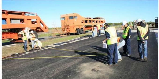
**Figure G.43. Measurement of the positions of CTL strain gauges on first lift of PG 64-28PM, before placement of second lift.**
