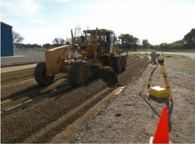
**Figure G.9. Aggregate base grading.**
