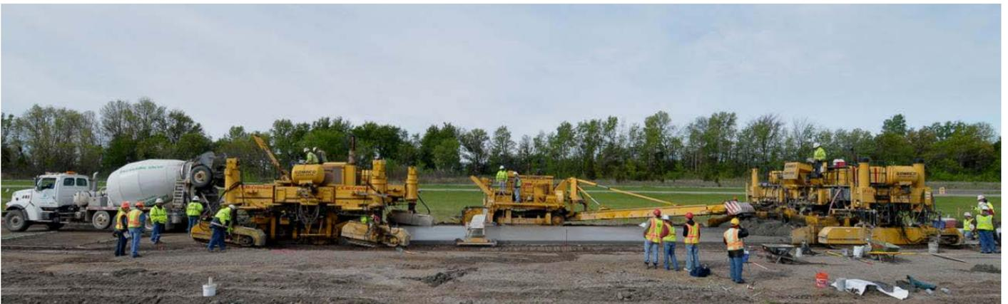
**Figure F.25. Paving train constructing R21 test sections along I-94 at MnROAD. Pictured from left to right are the mixer truck, first paver, belt placer, and second paver.**
