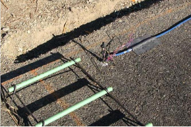
**Figure G.23.** Cable-fastening process showing a combination of Bituthene and nail methods.
