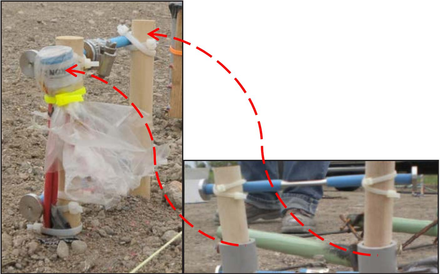
**Figure H.12. Technique for installing the static strain gauge in the upper concrete layer for Cells 71 and 72.**
