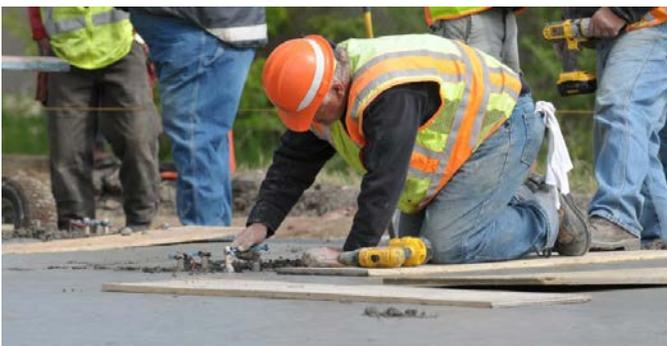
**Figure H.13. Installation of the static strain gauge for the upper concrete layer for Cells 71 and 72.**
