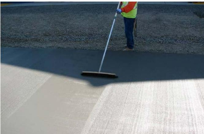
**Figure G.30. Texturing the concrete surface.**
