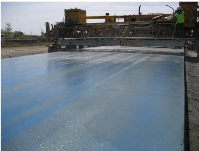
**Figure V.15.** *Streaked application of MBT Reveal on the demonstration slab.*
