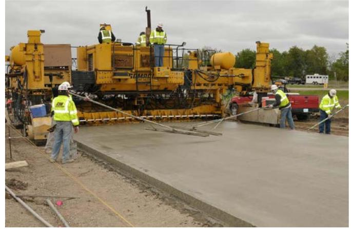
**Figure F.21. Finishing the PCC surface to remove surface irregularities.**
