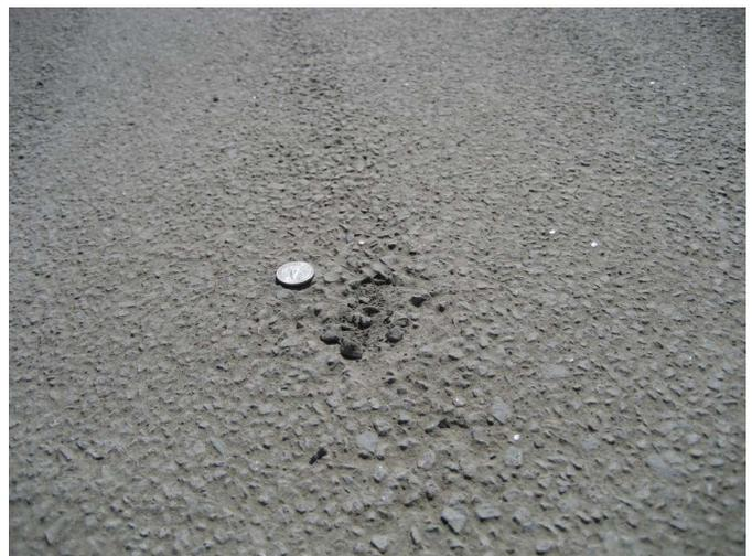
**Figure V.19.** Area of EAC surface that was not closed before brushing.
