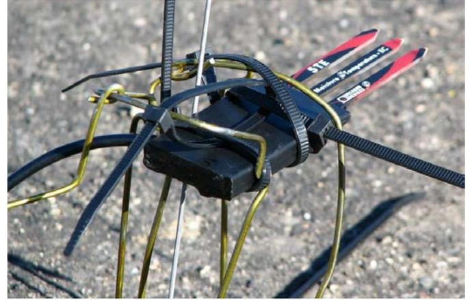
**Figure G.20. Moisture sensor in place before PCC placement.**
