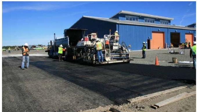
**Figure G.45. Paving top lift 2-in. (50-mm) RHMA-G in Lane D, Section 1.**
