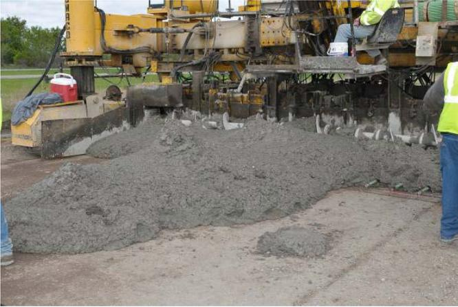
**Figure F.20. Placement of PCC layer on the aggregate base.**
