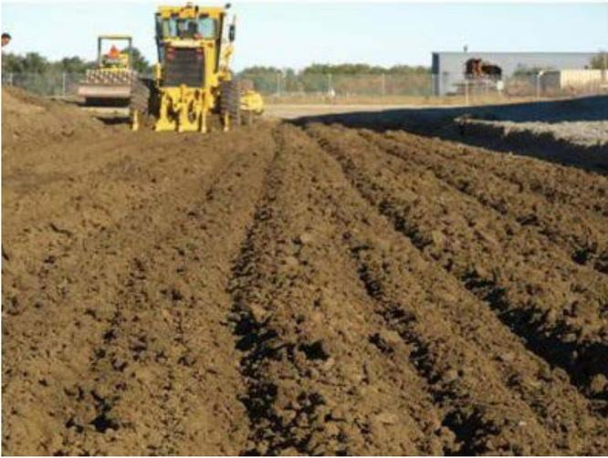
**Figure G.6. Scarification and drying of test track subgrade before grading and compaction.**
