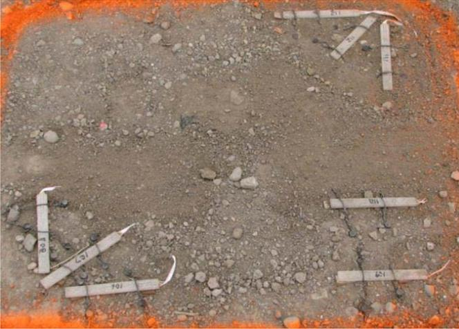
**Figure H.14. Dynamic strain gauge installation for Cell 70.**
