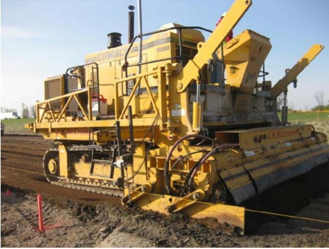
**Figure F.11. Trimming the subgrade using a string line and trimmer.**
