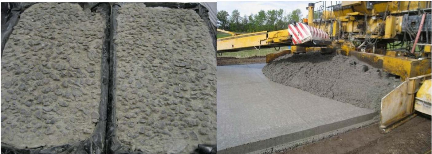
**Figure F.29. At left, PCC specimens cast in preparation for the paving and brushing of the PCC/PCC demonstration slab. At right, top surface PCC mix being placed in front of the second paver on site at MnROAD.**
