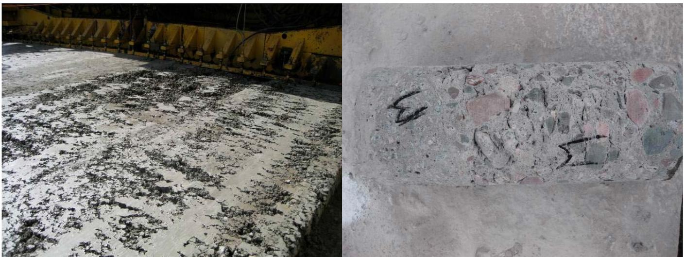
**Figure F.26.** At left, “torn” edges and surface caused by concrete setting on various parts of the paver; at right, coring showed poor mix consolidation in the lower PCC at select locations.
