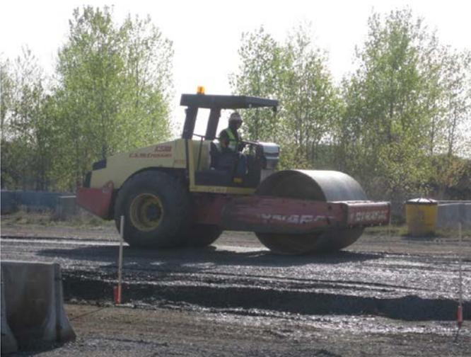
**Figure F.12. Compacting the subgrade using a steel drum roller.**
