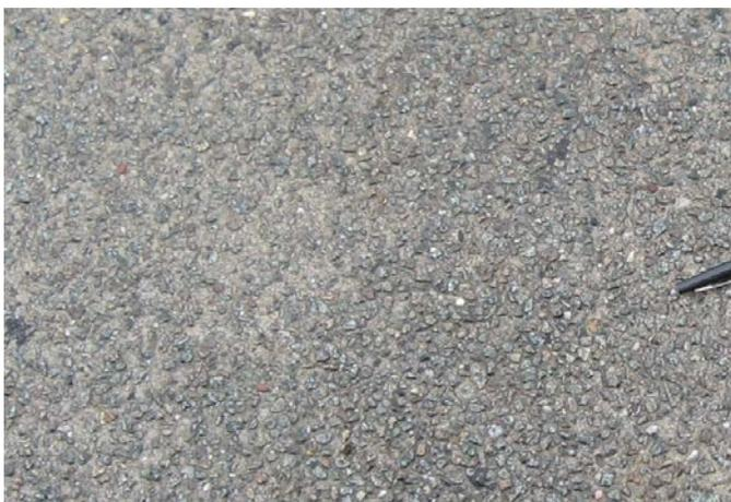
**Figure B.2.** An exposed aggregate PCC surface with pen cap at right for scale.
