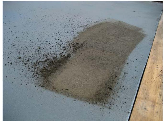
**Figure V.16.** *Evaluating brushing readiness of the EAC surface with a push broom.*
