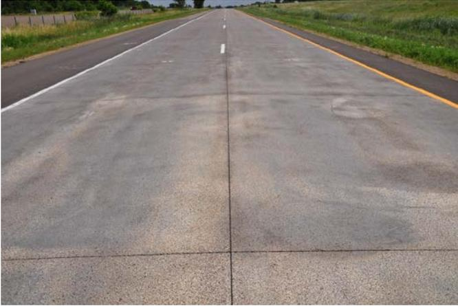
**Figure V.20. Streaked appearance of EAC surface caused by caking of paste by brush machine wheels.**
