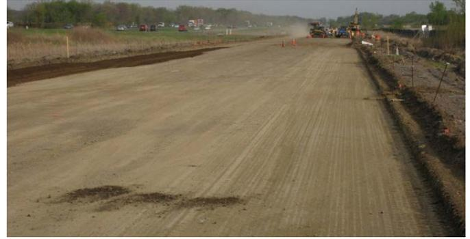
**Figure F.13. Trimmed and compacted subgrade.**
