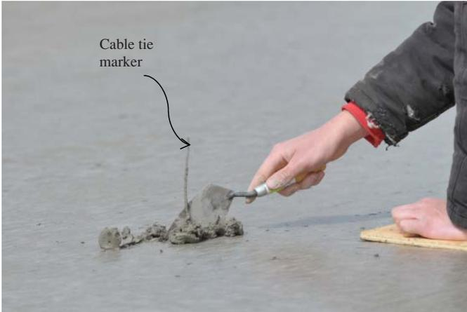
**Figure H.3.** Cable ties attached to the dowel so that the sensor locations could be easily located.
