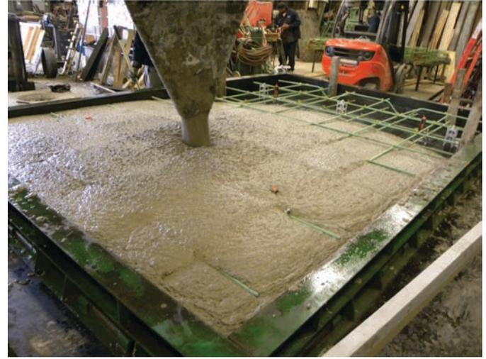
**Figure 9.7. Placement processes for slump concrete and SCC.**
