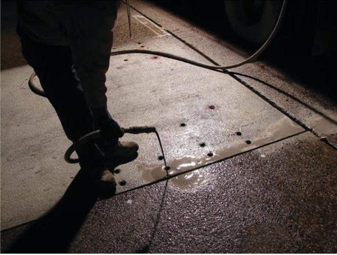
**Figure 10.7. Dowel slot grouting.**
