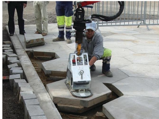
**Figure 2.17. Installation of keyed hexagonal panels in France.**
