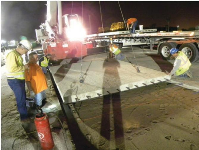
**Figure 6.3. Footprints indicate a poorly compacted fine-grained bedding layer.**
