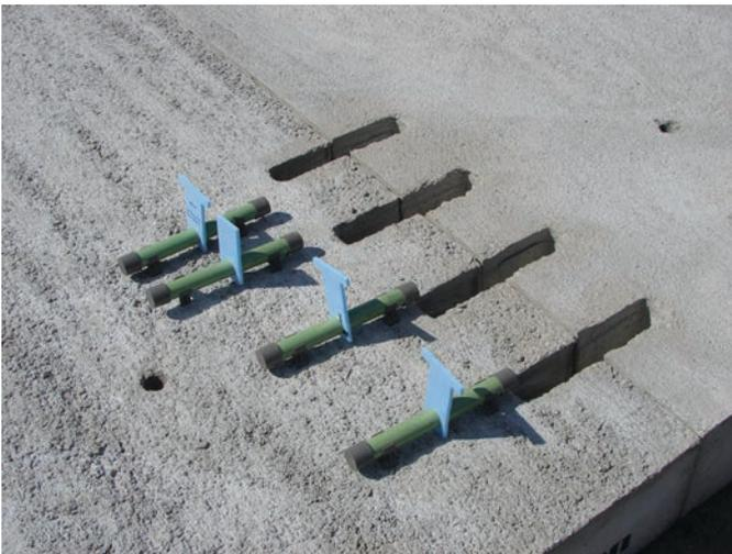
**Figure 10.8. Slot patching for DBR.**
