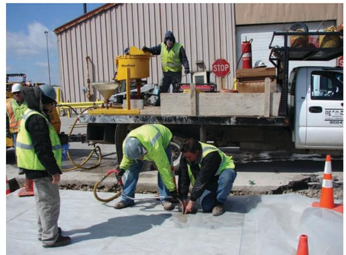
Figure 10.9. Undersealing grout pump and grouting operation.
