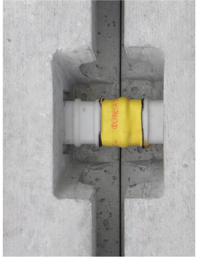
**Figure 7.2.** Shrink-wrap coupler use with the double keyway detail.
