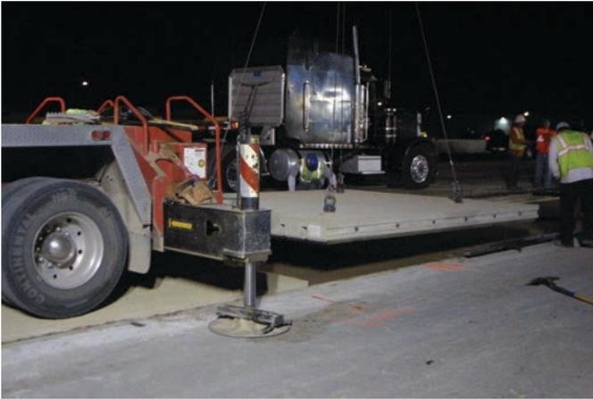
**Figure 15.6. Crane stabilization requires 2 to 3 additional feet away from the rehabilitation lane on each side.**
