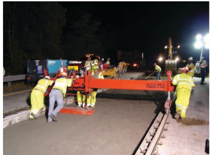
**Figure 6.1. Auger-based granular base grading system.**
