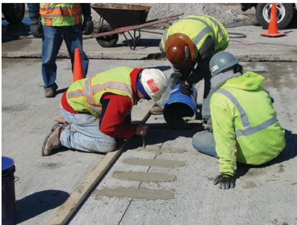
**Figure 2.4.** Variation of intermittent repair technique with dowel bars installed after panel installation using DBR method.
