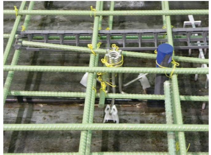
anchors to pull out under load. In addition, any dynamic loading during lifting and installation at the work site should be accounted for in the design of the anchorage system. A static analysis should also be conducted using the proposed lifting system to ensure that the tensile stresses that develop in the panel are within acceptable limits, especially during the initial lift soon after casting.
