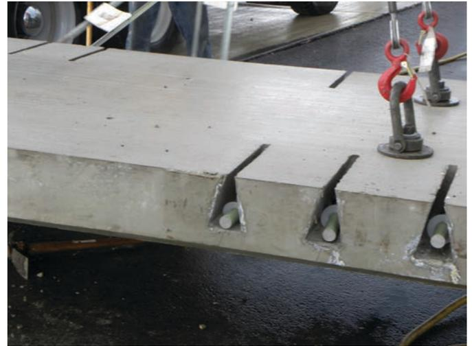
**Figure 14.5. Narrow-mouth surface dowel slots.**
