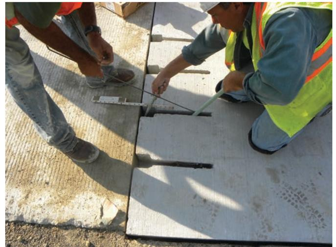
**Figure 14.6. Narrow-mouth dowel slot use for repair applications.**
