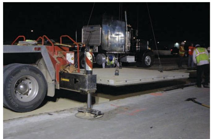
Figure 4.4. Outrigger positioning of lifting crane.
