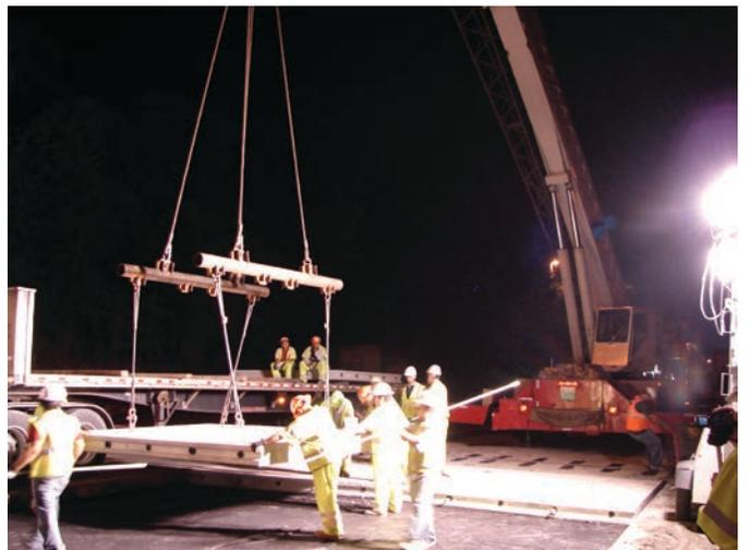
Figure 15.5. Typical panel-lifting equipment.
