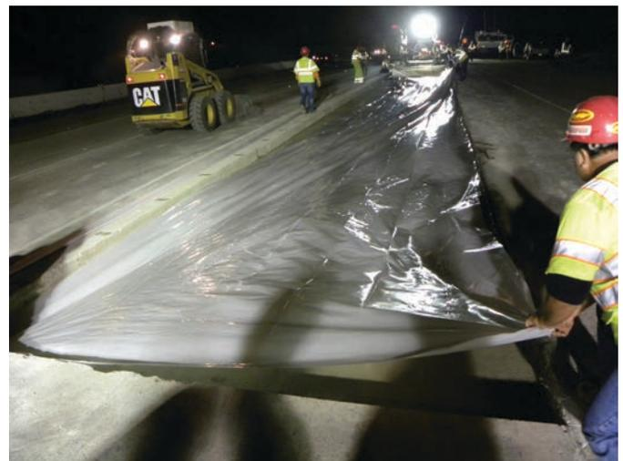
**Figure 12.1.** Placement of polyethylene sheet or geotextile fabric.
