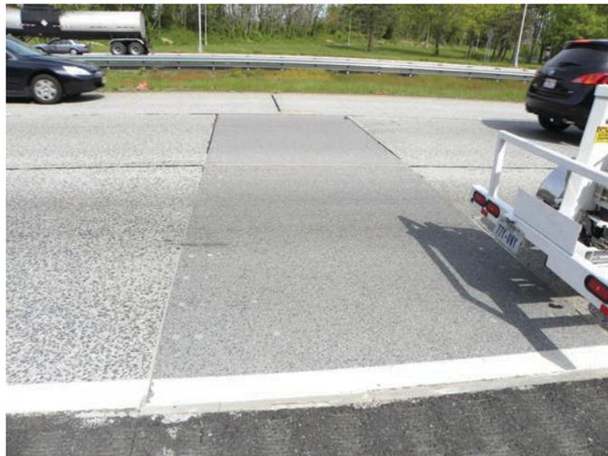
The project was tested during the nighttime in April 2010. Ten precast panels and 10 existing JRCPC slab panels (adjacent to the precast panels) were tested. At the time of testing the project had been milled in anticipation of an AC overlay. Overall condition of the repair panels tested appeared to be good, considering the surface had been milled. The joint condition could not be determined because of the milling and the nighttime condition. The pavement condition is shown in Figure 3.4.
