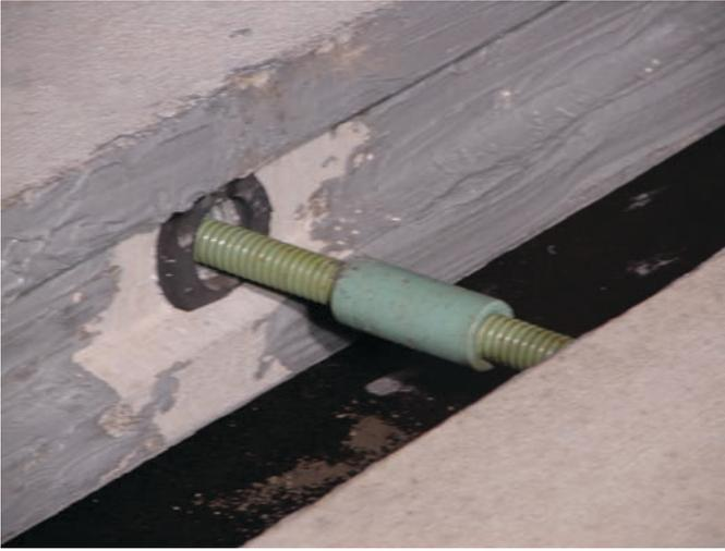
**Figure 12.4. Gasket placed on tendon duct.**
