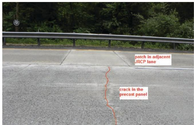
**Figure 3.11. Crack in a precast panel associated with a patch in the adjacent lane on I-66 in Virginia.**
