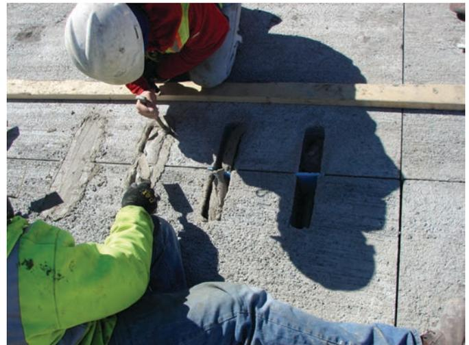
Whether a grout material or a rapid-setting patching material is used for the dowel slots, the material should attain the required strength, typically 2,500 lbf/in.<sup>2</sup> (17.2 MPa), before opening the repair area to traffic.
