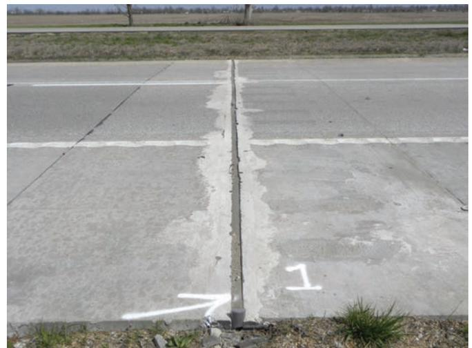
Figure 3.18. PPCP-reconstructed expansion joint on I-57 in Missouri.
