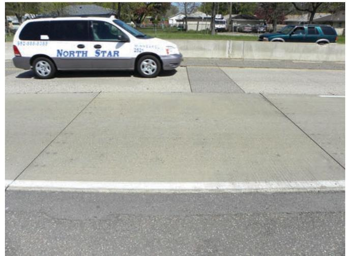
**Figure 3.9. Views from the Minnesota TH-62 project (precast panels in right-hand lane).**
