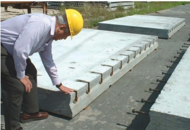
**Figure 2.12. Kwik Slab joint interlocking system.**
