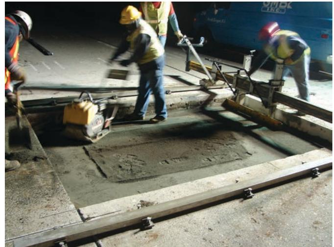
**Figure 10.2.** Base being graded and compacted within the repair area.
