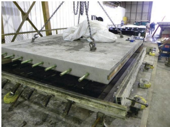
**Figure 4.2. Typical four-point lifting of a precast panel.**
