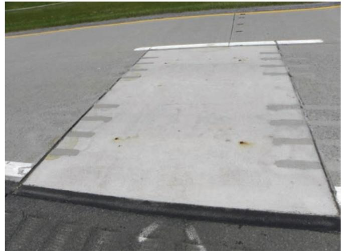
**Figure 3.5. Views of the precast panels at the Route 27 project in New York.**
