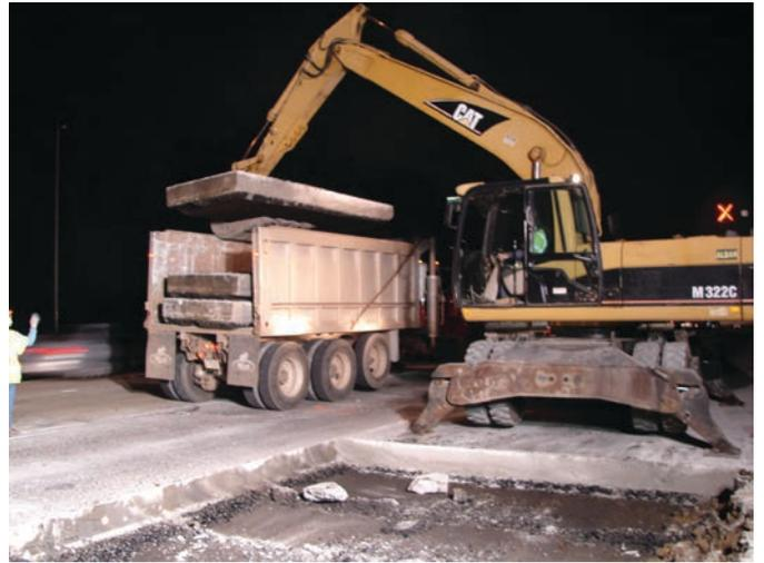
Figure 15.4. Different types of pavement removal equipment.
