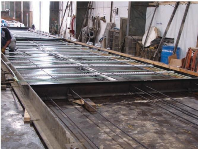
**Figure 9.2. Formwork modified to allow for pretensioning strands.**
