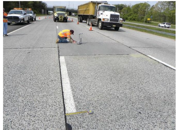
**Figure 3.3. Views of the I-295 precast panels in New Jersey.**
