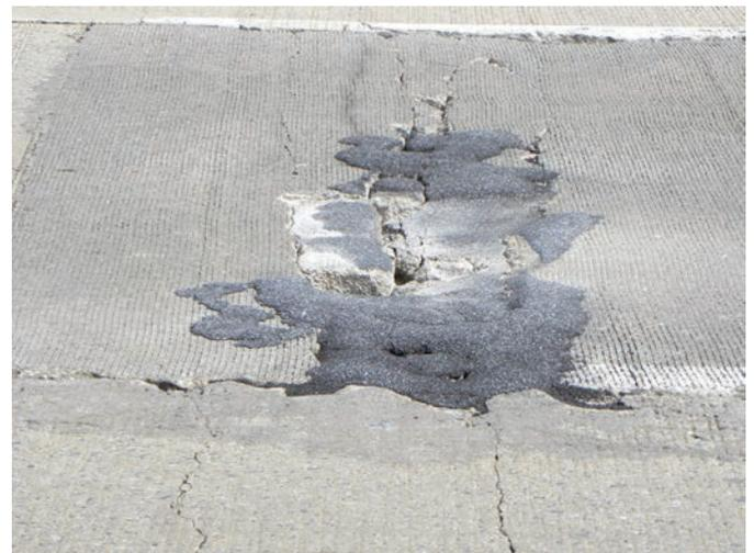
**Figure 14.3. Failed FDRs in CRCP.**
