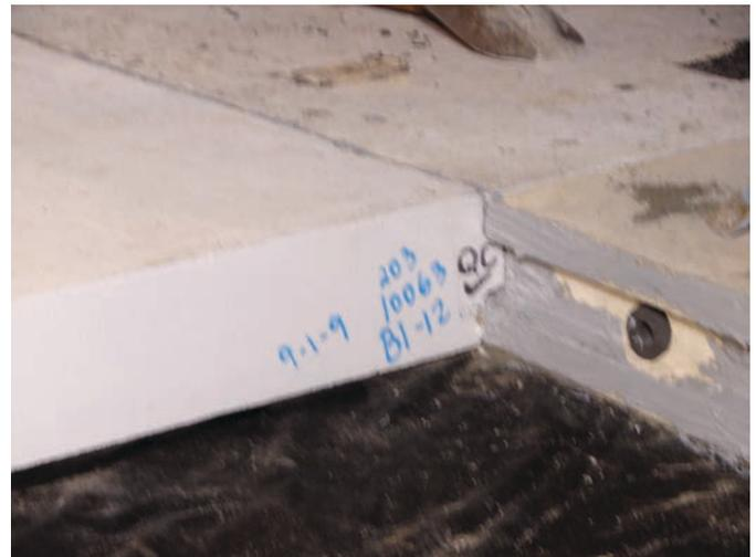
**Figure 12.5. Intermediate keyway joint.**
