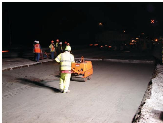
Figure 11.1. Manual base grading.
