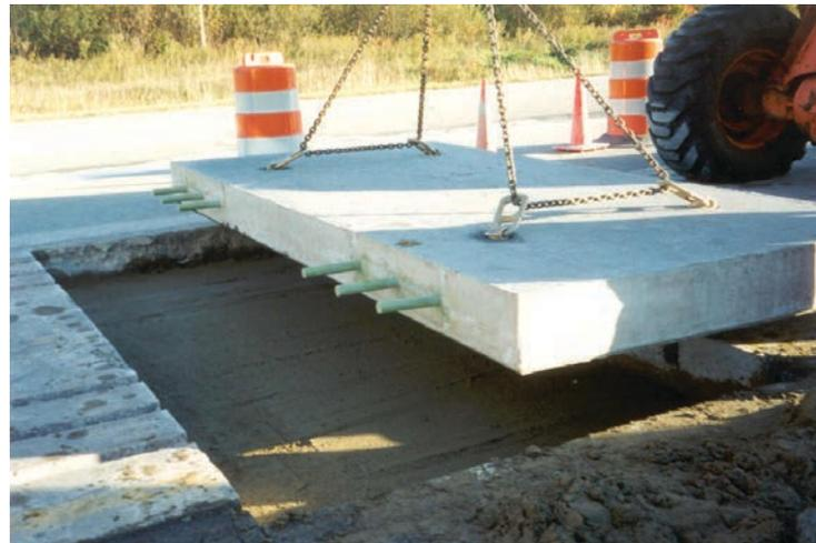
**Figure 2.3.** Variation of intermittent repair technique with slots for dowel bars cut in existing concrete pavement.
