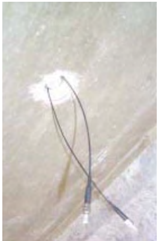
Figure 4: Fiber optic sensor fully installed
