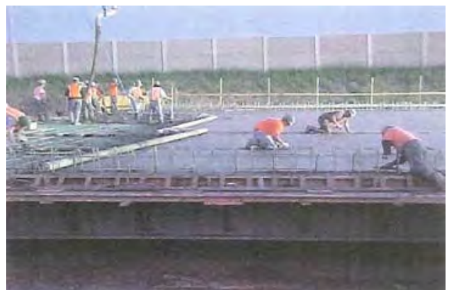
Figure 3: Placement of concrete at prefabricated structure at same off-site location
