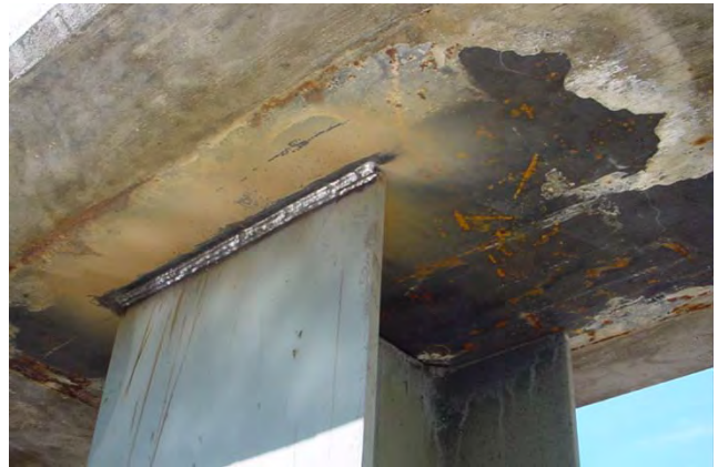
Figure 8: H-pile welded to plate cast into the underside of the abutment, as shown in Figure 1
