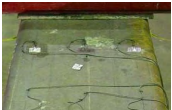
Figure 5: Linear strain gauges installed on top flange
