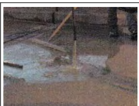
Figure 4: Spreading of epoxy onto concrete deck surface
