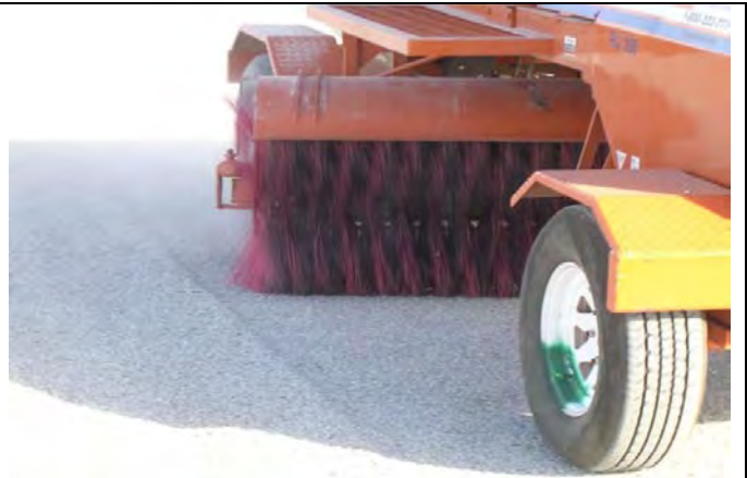
Figure 7: Sweeping of overlay after curing
