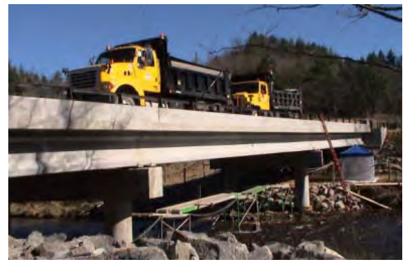
Figure 6: Load testing of bridge
