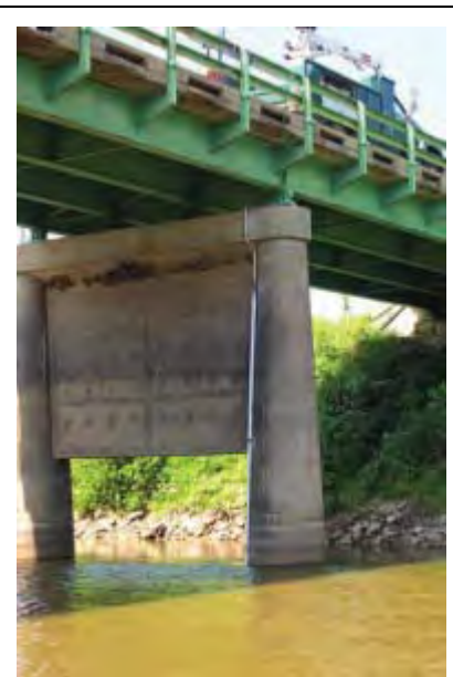
Figure 2: Installed conduit for RCBM at structure L-344, pier 4
