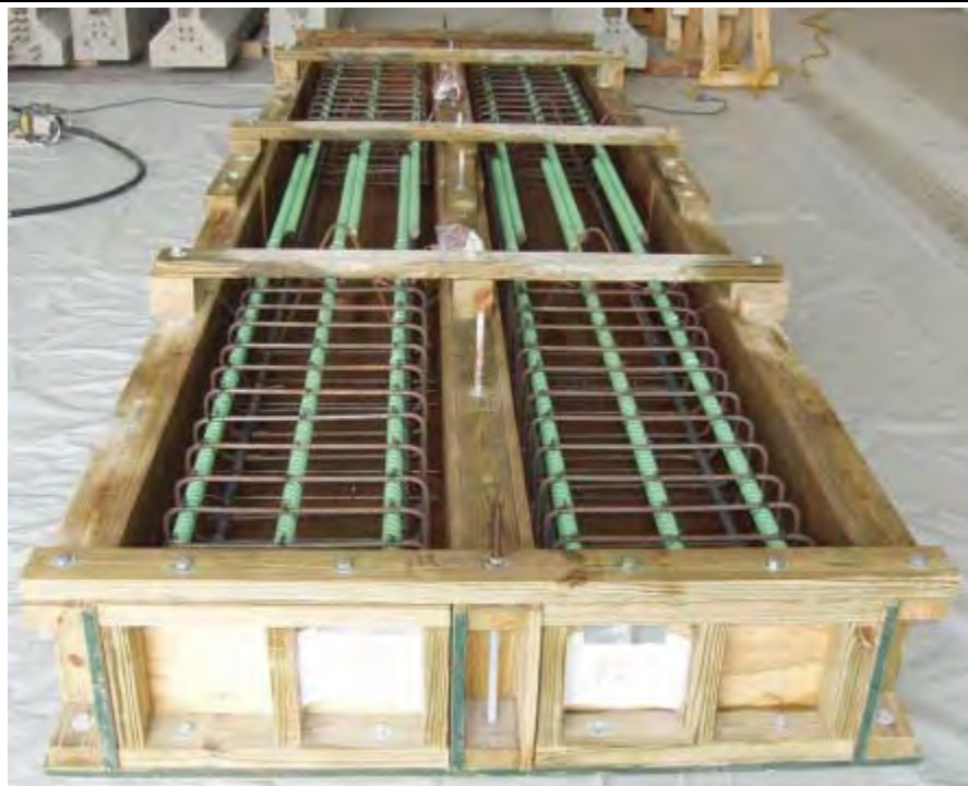
Figure 1: Epoxy coated rebar used during testing
