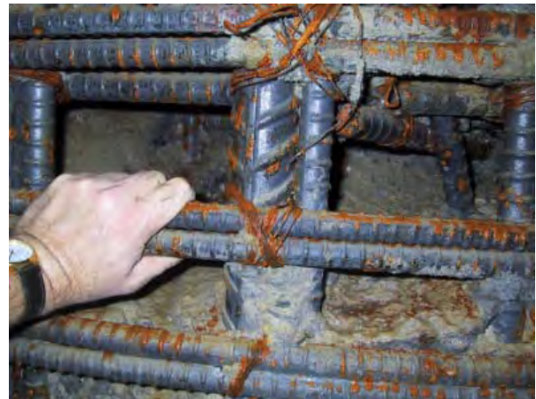
Figure 1: Various defects in drilled shafts, throughout the United States, due to loss of workability
