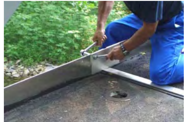
Figure 11: Aluminum connector plates installed at panel edges to join adjacent panels
