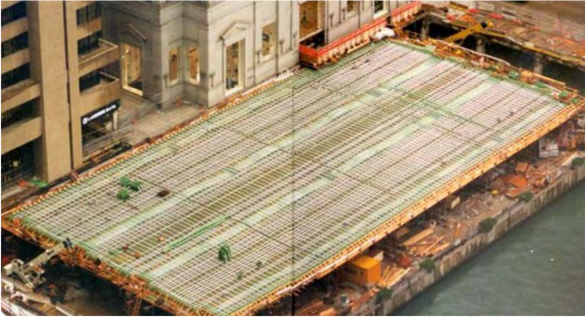
Figure 4: Aerial photo of deck construction during rebar placement
