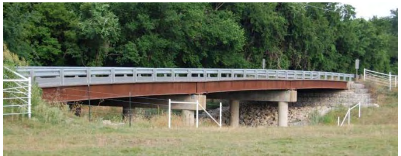
Figure 1: Completed Eighteen Mile Creek bridge
