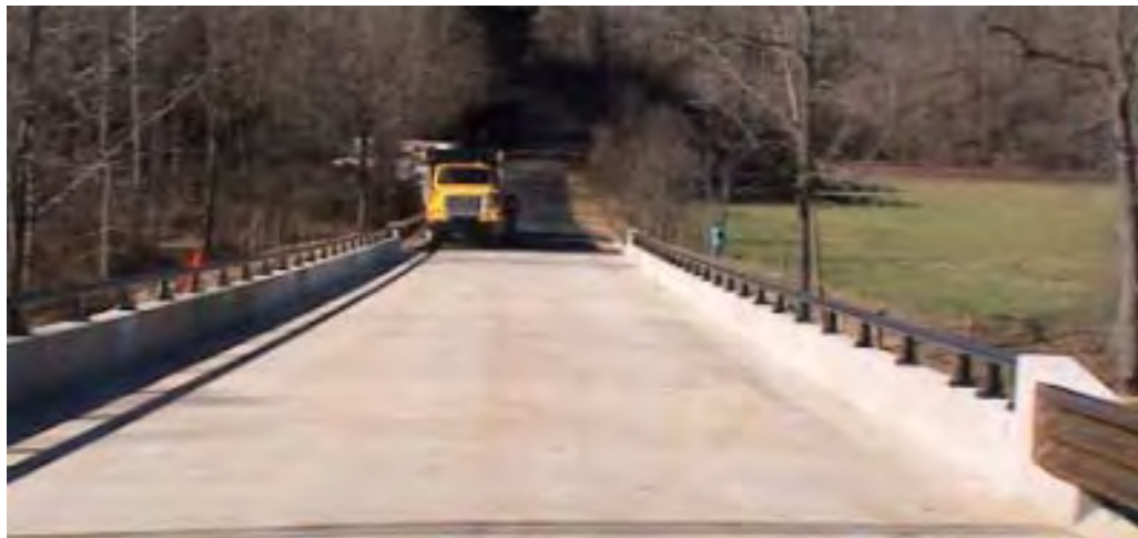
Figure 1: Completed bridge deck at SR 1470 over Cartoogechaye Creek
