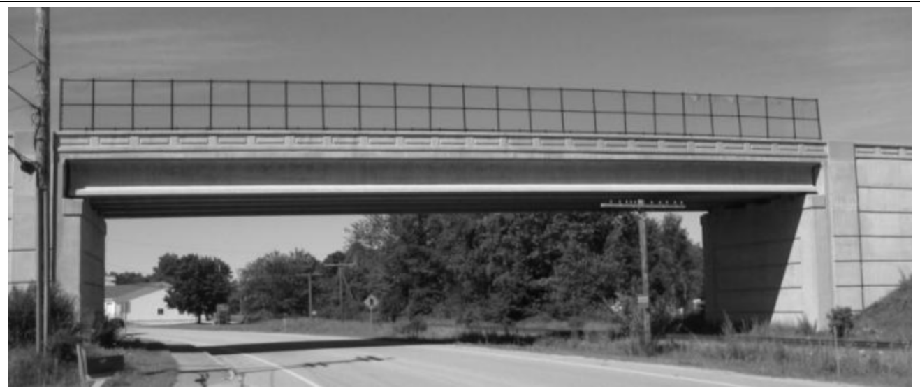
Figure 1: Completed Rolling Road Bridge in the year 2000
