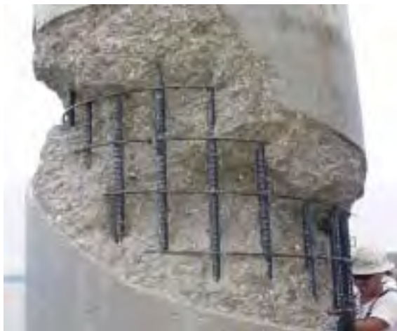
Figure 1: Various defects in drilled shafts, throughout the United States, due to loss of workability
