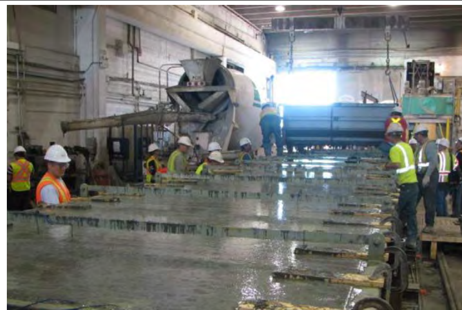
Figure 6: Pi-girder fabrication process at plant
