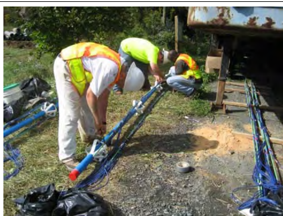
Figure 3: Assembly of the inclinometer and strain gages
