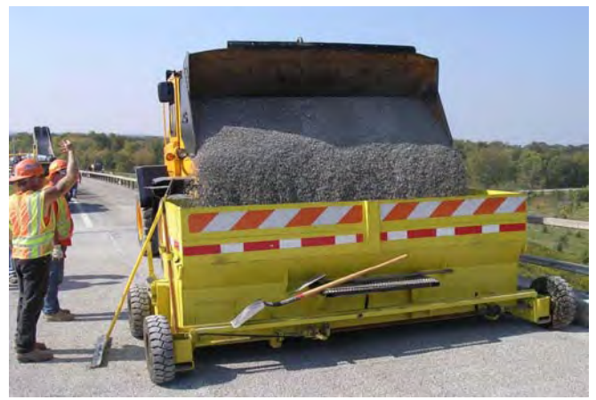
Figure 5: Aggregate spread over epoxy surface using spreader box
