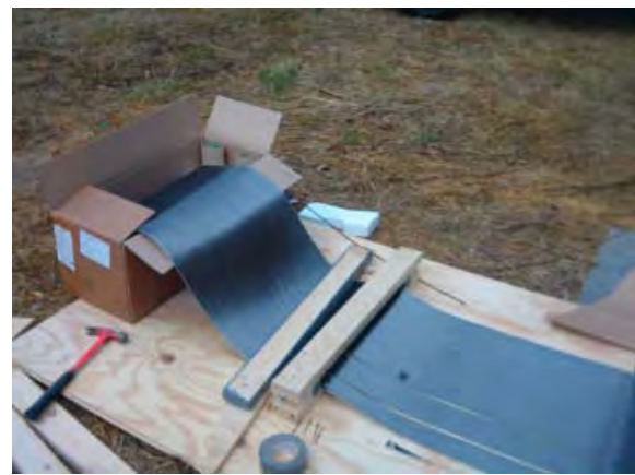
Figure 2: Manual lay-up CFRP Sheets
