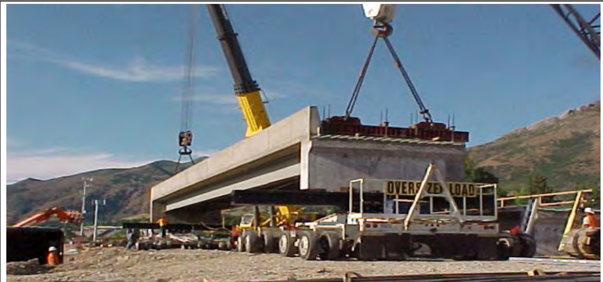
Figure 1: Bridge lowered onto SPMT for transport to bridge site
