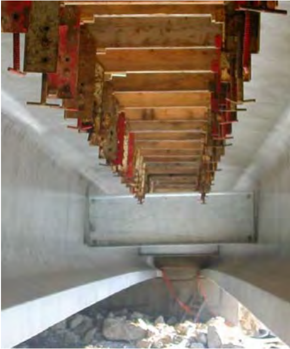
Figure 4: Small formed span between flanges
