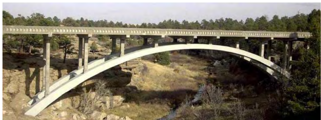
Figure 1: Renovated Castlewood Canyon Bridge rib arches
