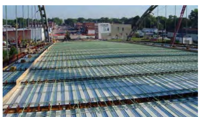
Figure 13: Deck slab reinforcement installation
