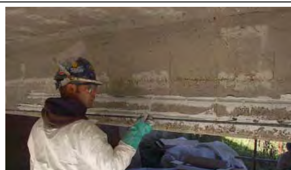
Figure 4: CFRP NSM mounted bars
