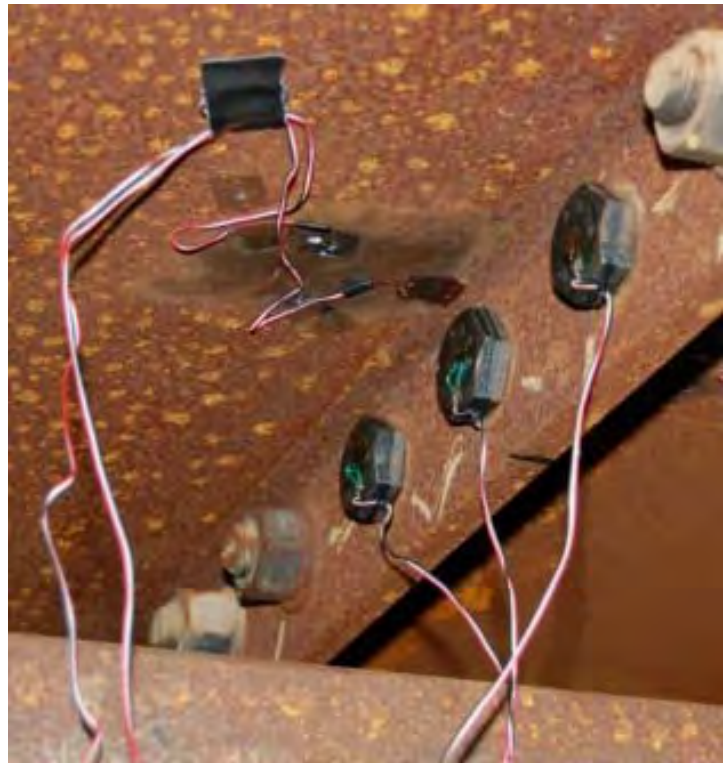
Figure 6: Strain gauges installed to bolted connections
