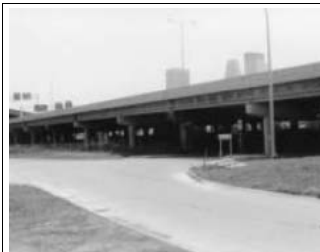
Figure 1: Bridge No. 27831 on I-394 over Dunwoody Boulevard
