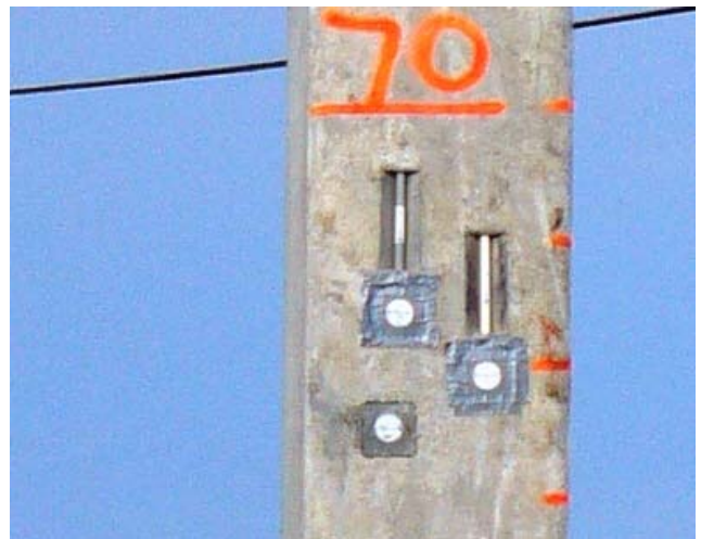
Figure 5: Installed data collectors used during pile driving
