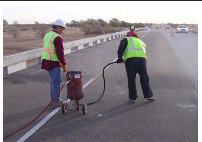
Figure 3: Sand blasting of existing surface to remove any dust, contaminants or other loose material
