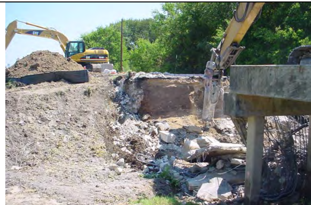
Figure 3: Demolition and removal of existing bridge
