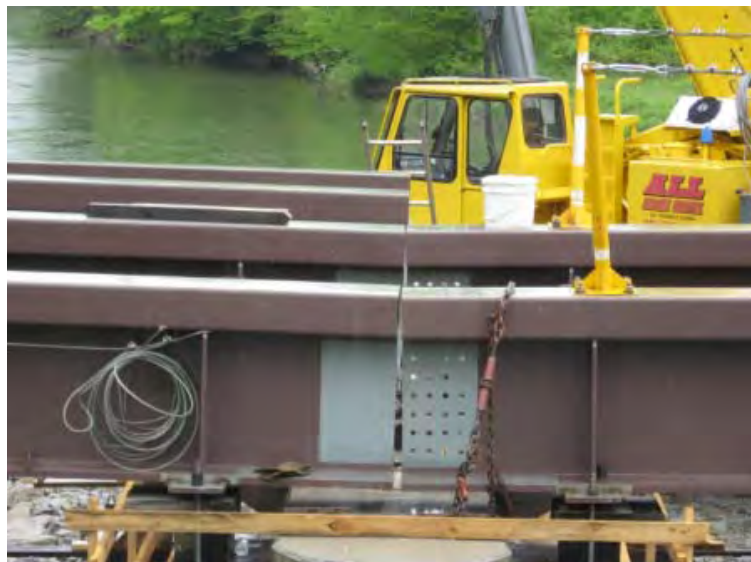
Figure 3: Field splice at pier
