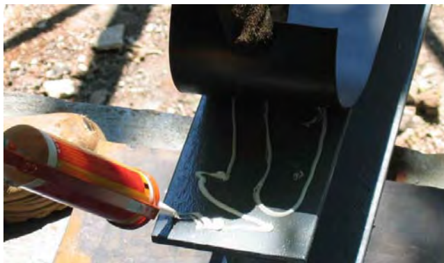
Figure 8: Isolating sheet adhered to top flange
