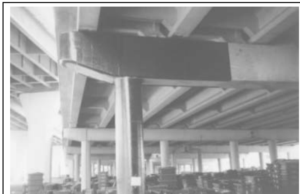
Figure 6: Installed wraps at pier cap
