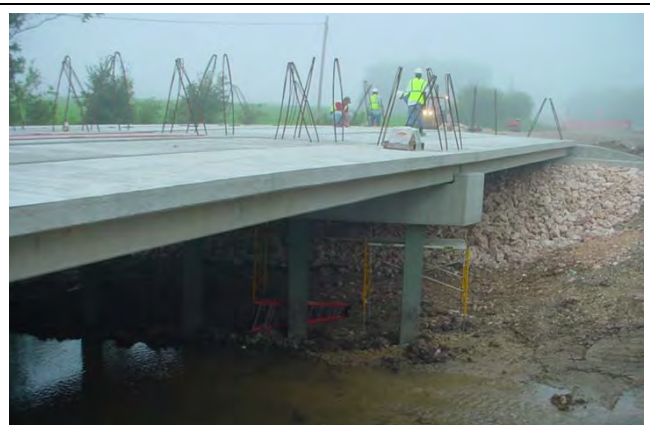
Figure 12: Final placement of girders
