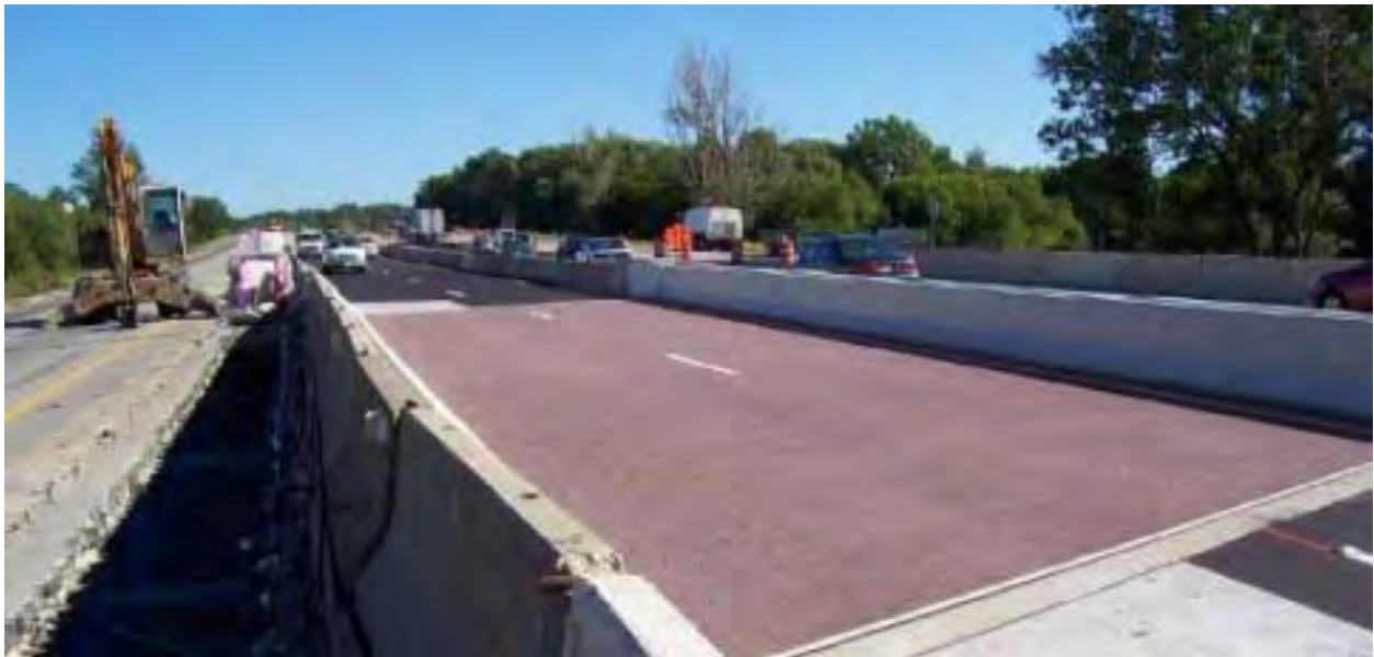
Figure 1: Completed deck surface at Door Creek Bridge
