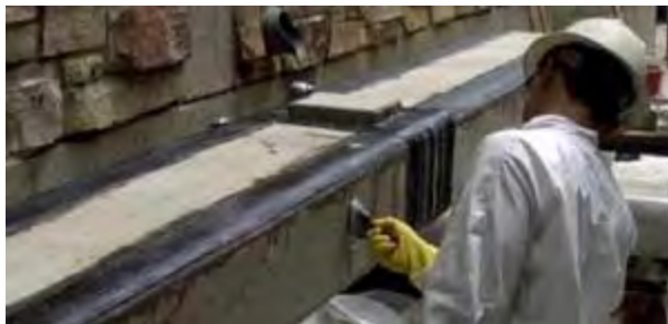
Figure 3: Epoxy overcoating in progress
