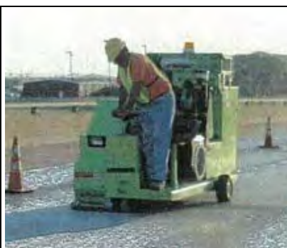
Figure 3: Shot blasting of existing concrete deck surface
