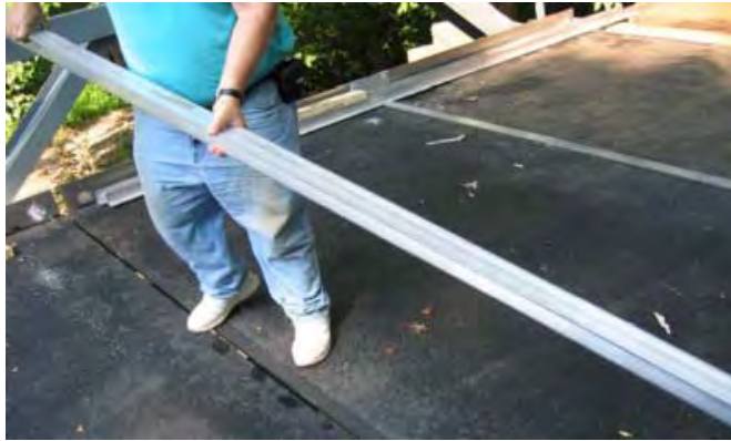
Figure 12: Inserting T-sections between panels
