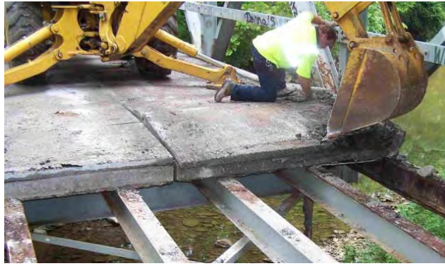
Figure 4: Removal of existing deck and damaged/corroded members
