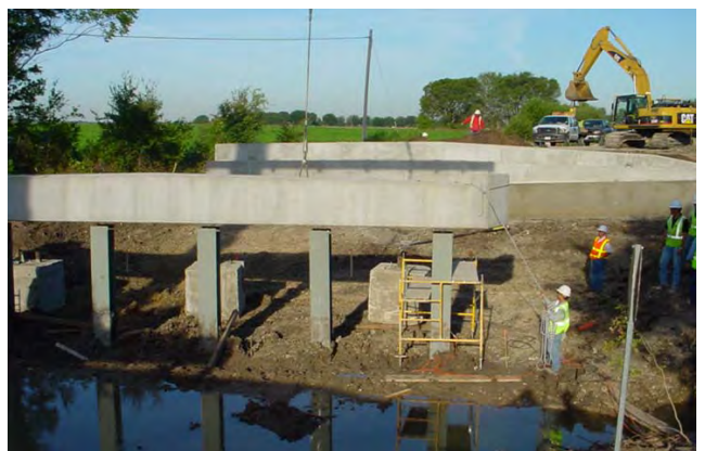
Figure 10: Bent cap and other abutment constructed
