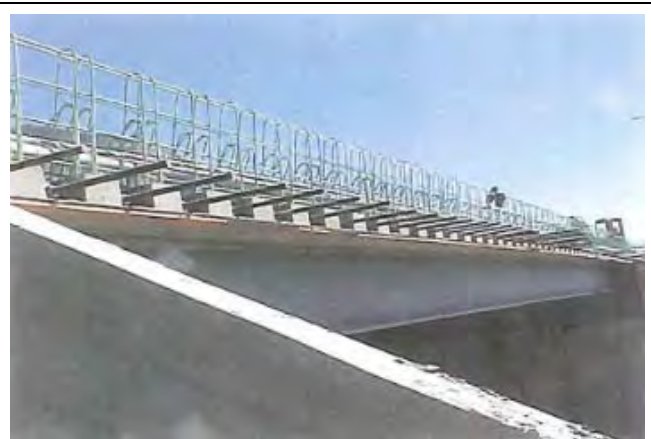
Figure 7: Post tensioning bars installed and ready for tensioning
