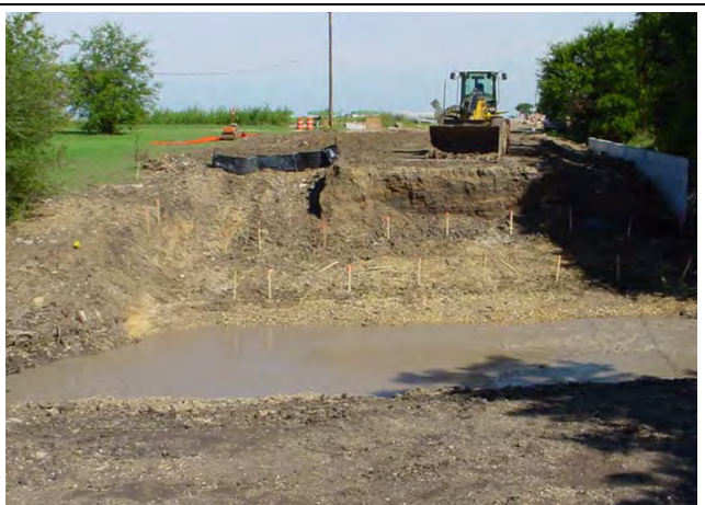
Figure 4: Site grading after bridge removal
