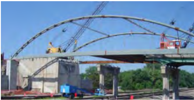
Figure 8: Arch bracing with temporary horizontal supports
