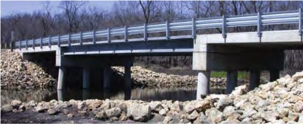
Figure 1: Completed Jakway Park Bridge, pi-girders used for middle span only
