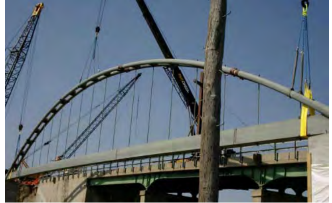
Figure 7: Installation of arches
