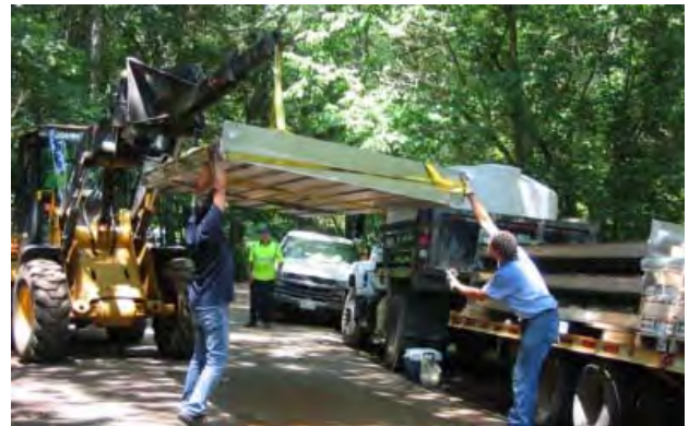
Figure 9: Panels delivered to site
