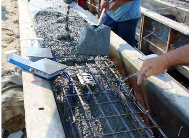
Figure 4: Placement of concrete in the pile molds
