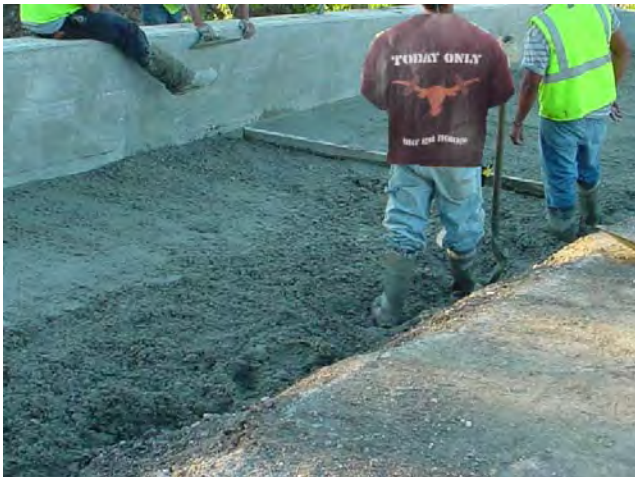
Figure 9: Abutment header at the back face of the abutment cast with flowable concrete fill
