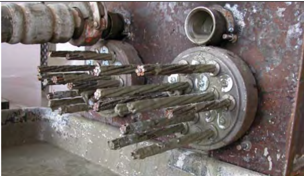
Figure 2: End of bottom chord
