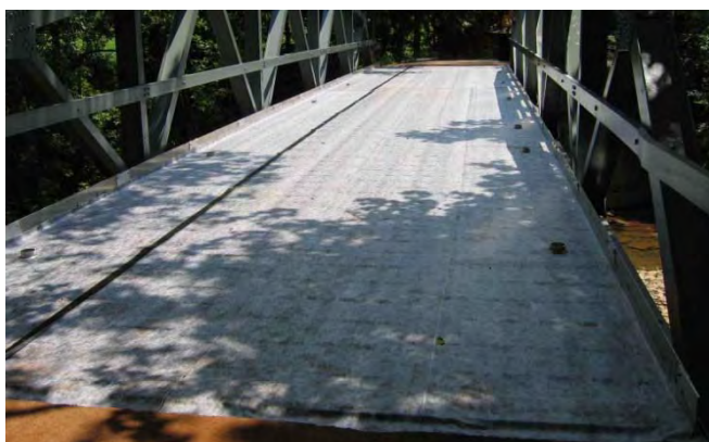
Figure 15: Water proofing laid on top of aluminum deck panels
