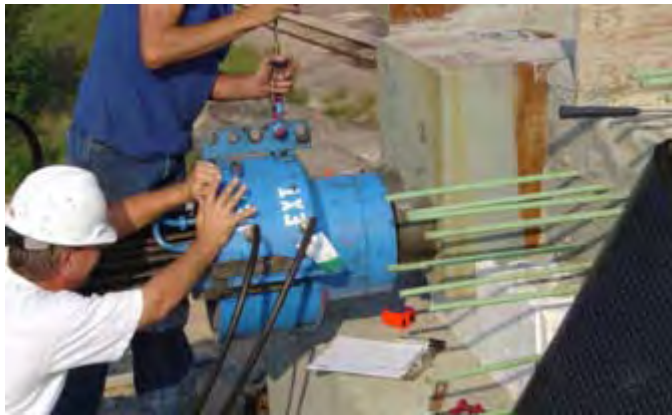
Figure 12: Ties being post-tensioned
