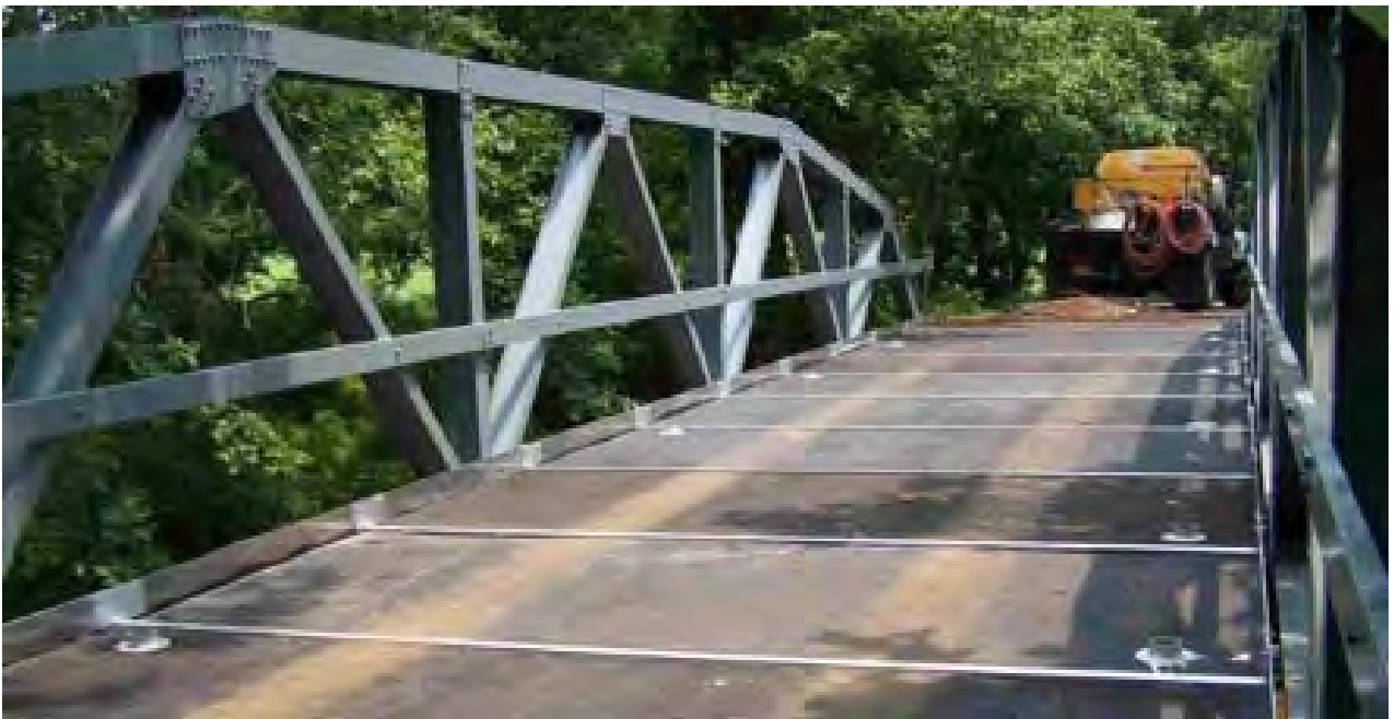
Figure 14: Finished installation of aluminum deck panels before overlay
