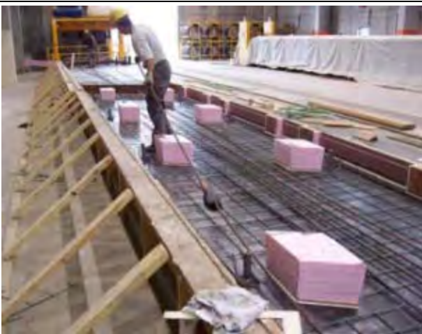
Figure 4: Prestressing strand being placed between foam blockouts and wire fabric prior to tensioning
