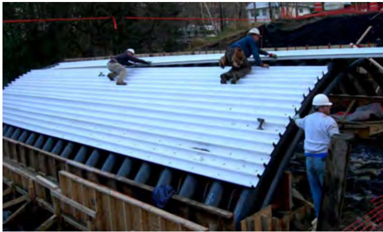
Photo 7. Final arch placement with corrosion resistant decking being installed
