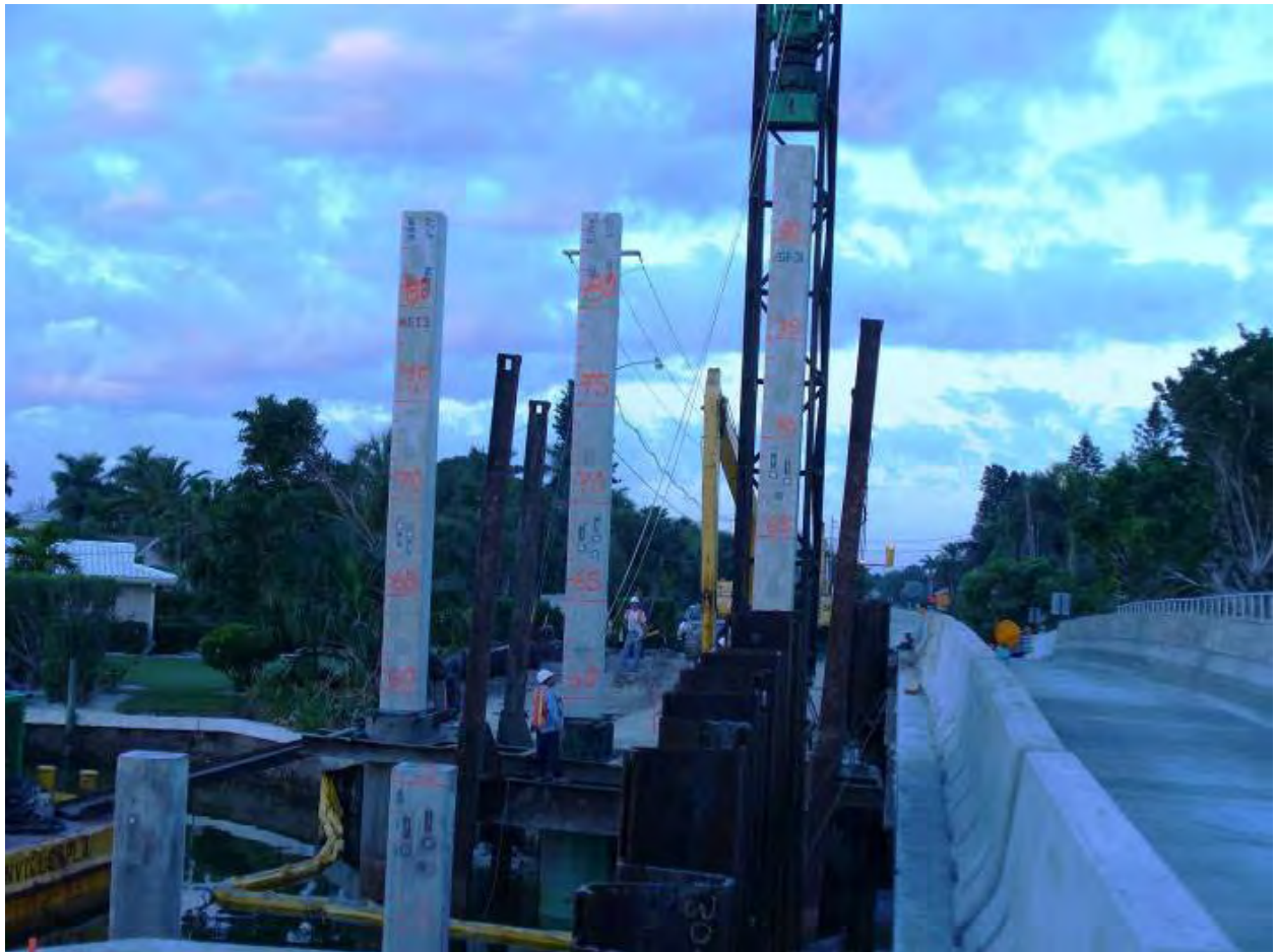
Figure 6: Piles being driven
