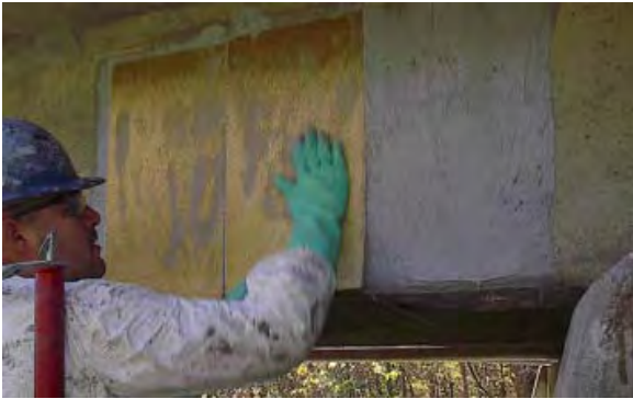
Figure 5: Manual lay-up SRP
