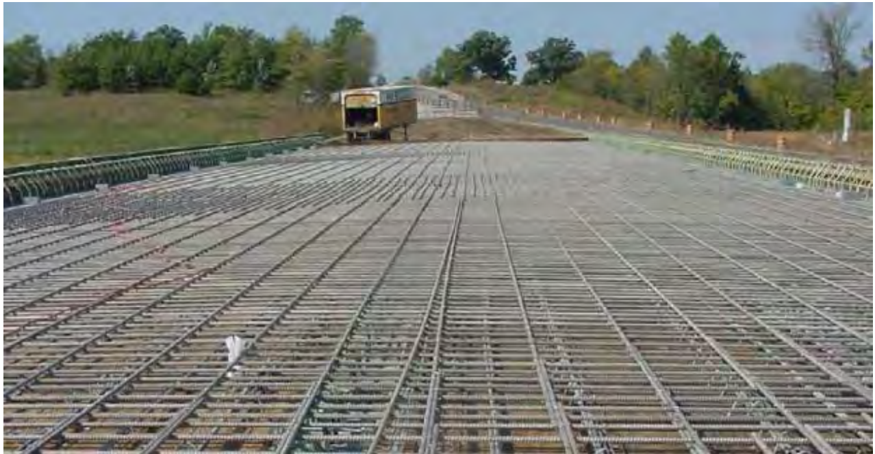
Figure 1: Stainless steel reinforcing at bridge A6059
