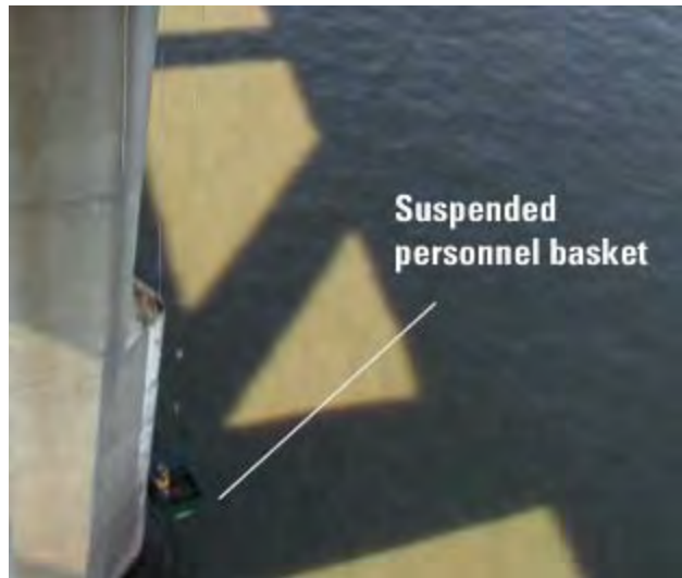
Figure 6: Basket used for RCBM installation
