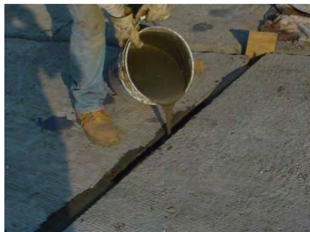
Figure 15: Non-shrink cementitious grout placed in longitudinal joint between girders
