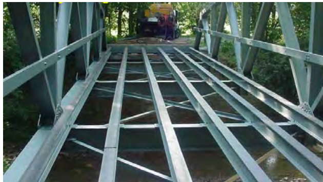
Figure 6: All steel members sand blasted/repainted
