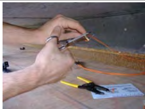
Figure 5: Cable spliced into new system for newly installed sensors
