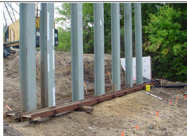
Figure 5: Driving of the H-piles, template used to align piles to abutment plate
