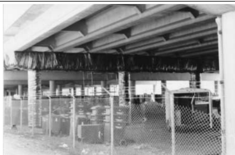
Figure 5: ECE system in place at Pier 37
