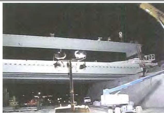
Figure 6: Positioning bridge element into final location
