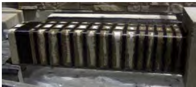
Figure 4: Finished wrap application
