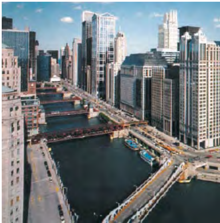
Figure 1: Wacker Drive project site
