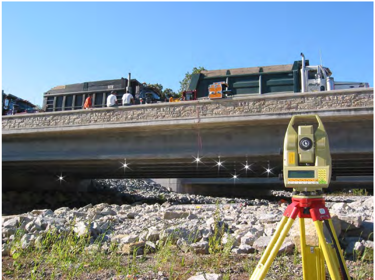
Figure 1: De Neveu Creek Bridge during load testing
