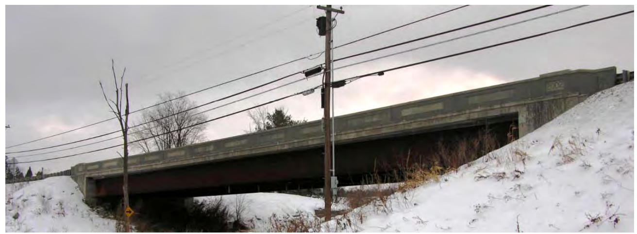
Figure 1: Completed Morristown Bridge in December 2005
