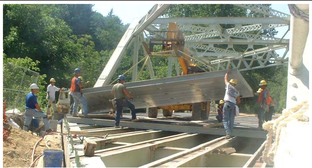
Figure 3: Forklift lowering deck panel into place near the end of the bridge
