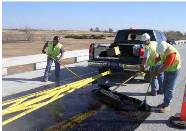
Figure 4: Epoxy mixed on site and applied using squeegees to the existing pavement surface
