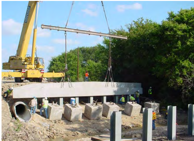
Figure 7: Placement of abutment onto H-piles by crane
