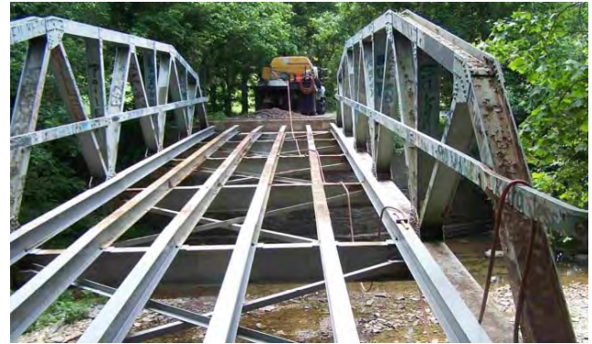
Figure 5: Repair and replacement of removed members
