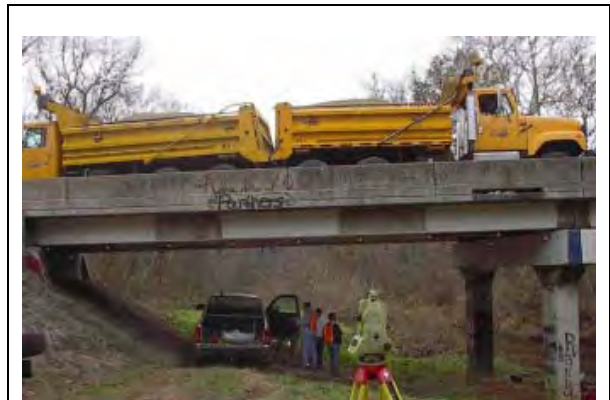
Figure 7: Two loaded H20 design trucks used for load testing
