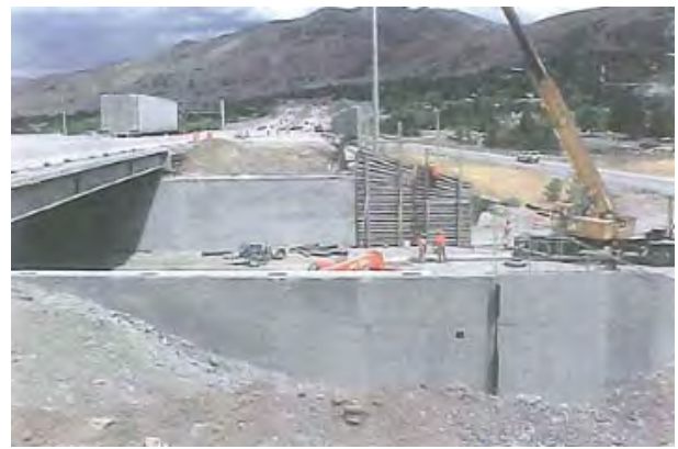
Figure 5: Existing northbound structure removed bridge
