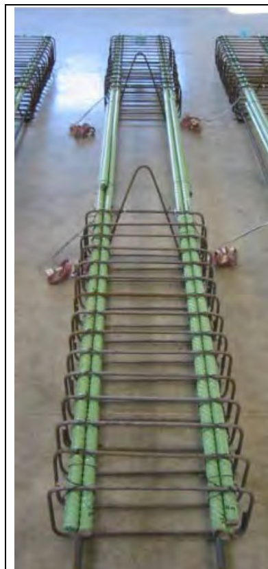
Figure 4: Reinforcement cage
