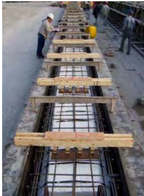
Figure 9: SCC beam with wooden void restraints installed and ready to be cast
