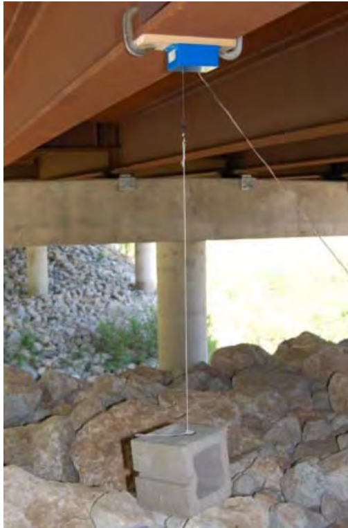
Figure 5: Potentiometers installed at midspan
