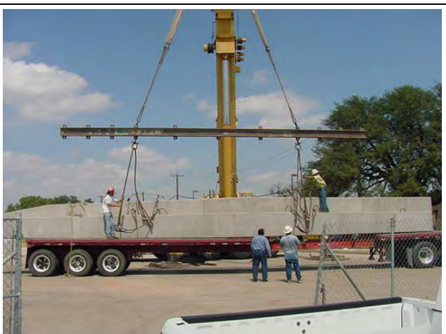
Figure 6: Abutment delivered to bridge site
