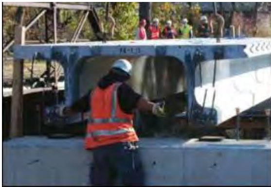
Figure 2: Second generation pi-girder
