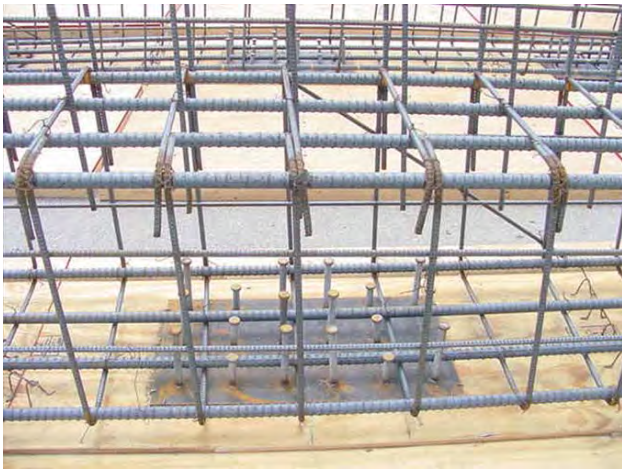
Figure 1: Rebar cages formed, H-pile connection plate with shear studs shown on bottom
