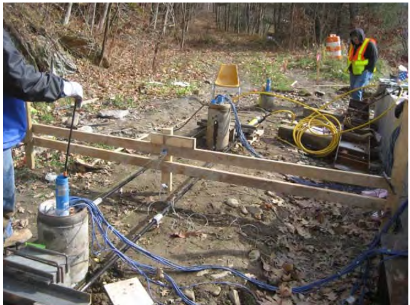
Figure 1: Load test showing load frame, reference beams, and actuators
