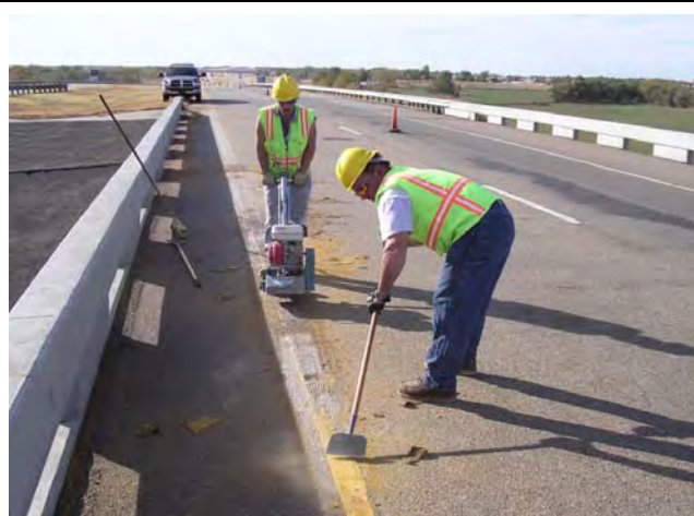
Figure 2: Grinding off existing striping
