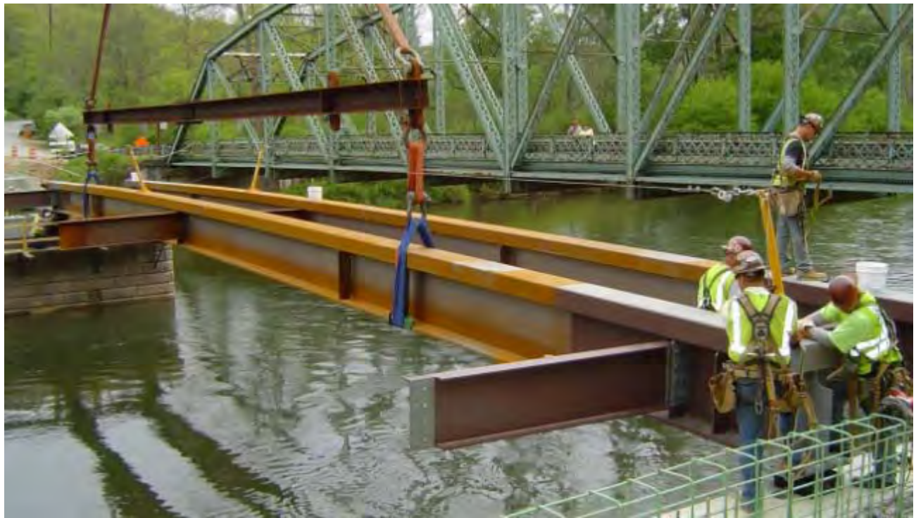
Figure 4: Construction of bridge on SR 1003 over Tionesta utilizing CFTFGs
