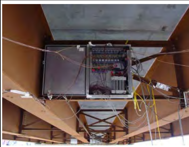
Figure 4: Data acquisition box at midspan
