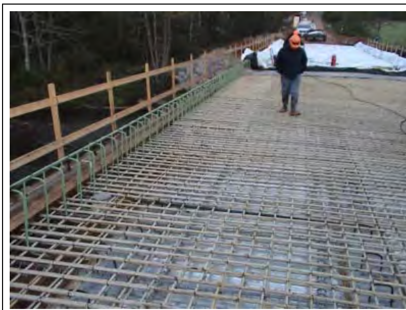
Figure 5: Completed deck reinforcement grid
