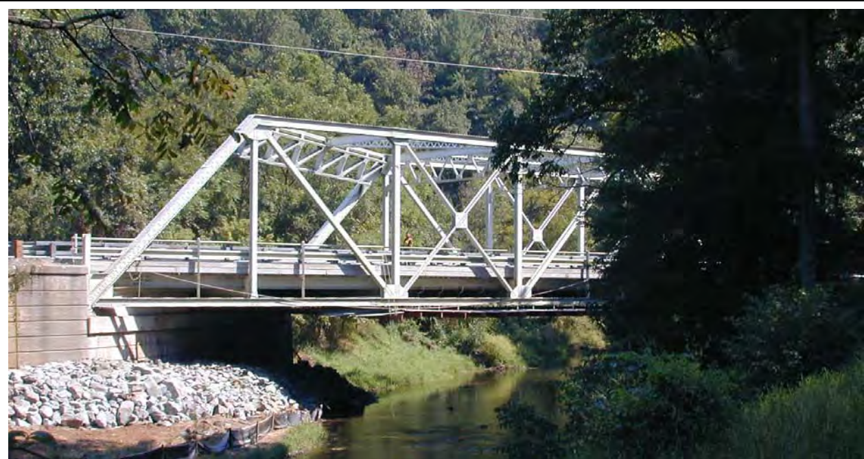
Figure 1: Rocks Steel Truss Bridge over Deer Creek
