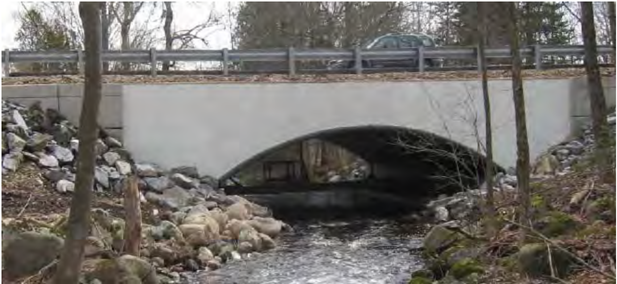
Photo 1: Completed Neal Bridge
