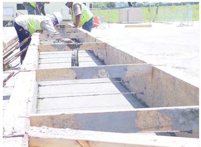
Figure 2: Fabrication of the abutments at off-site location, bent cap similar
