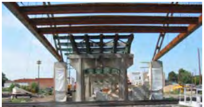
Figure 9: Floor beam placement
