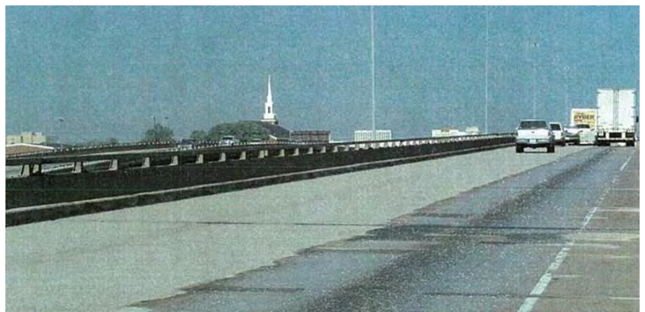
Figure 1: Westbound bridge with one lane treated with polymer overlay
