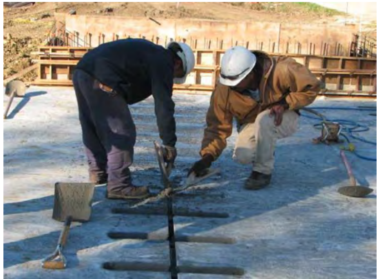
Figure 7: Grout pockets being filled
