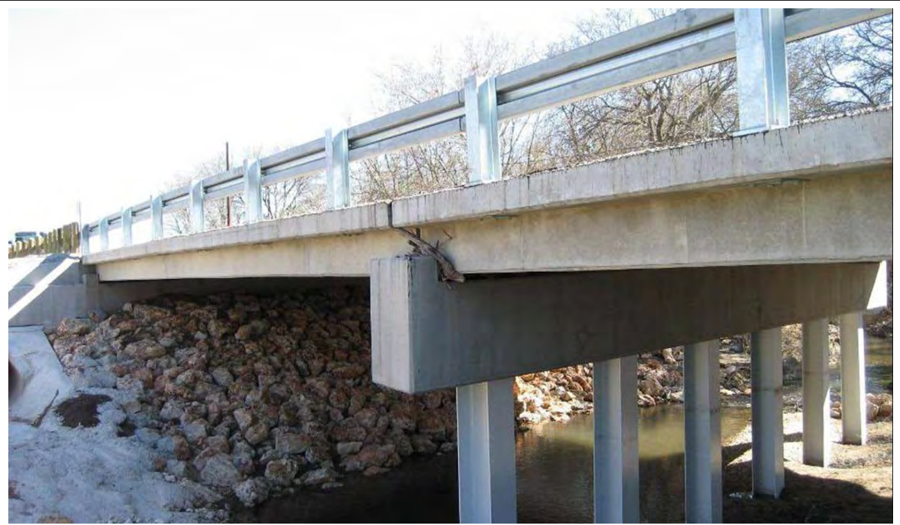
Figure 1: Completed Cottonwood Creek Bridge
