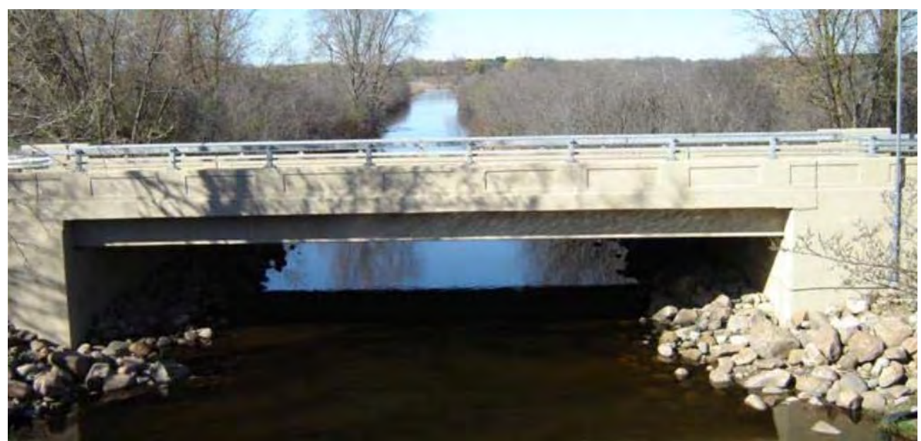
Figure 1: M-50/US-127 demonstration bridge using SCC beams
