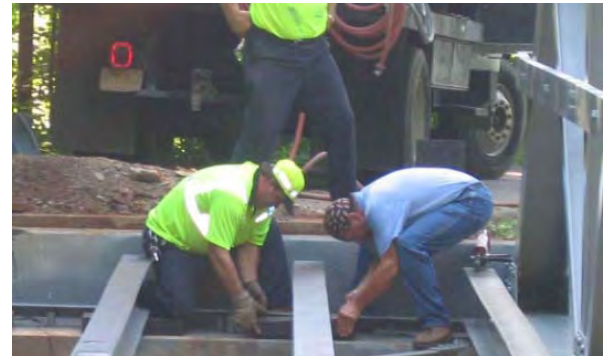
Figure 7: All bearings replaced
