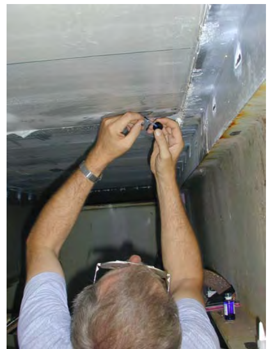
Figure 5: Installation of strain transducer at the underside of deck near girder
