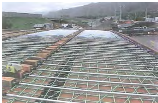
Figure 2: Construction of bridge at off-site location; post-tensioning ducts, block-outs, reinforcement, and formwork over steel girders shown
