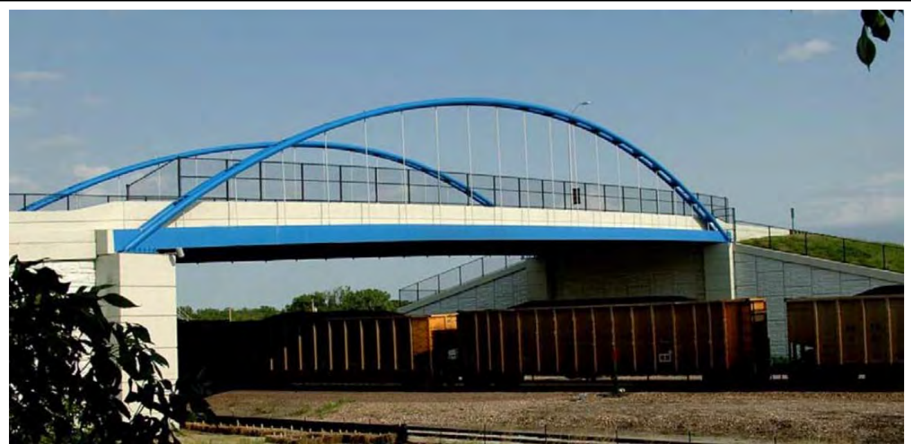
Figure 1: Ravenna Viaduct tie arch bridge after construction
