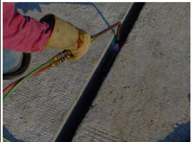
Figure 14: Weld at one inch diameter lateral connector rod to girder plate
