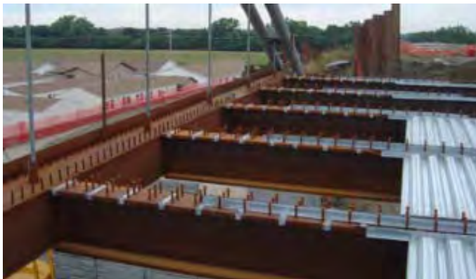
Figure 10: Metal decking installation
