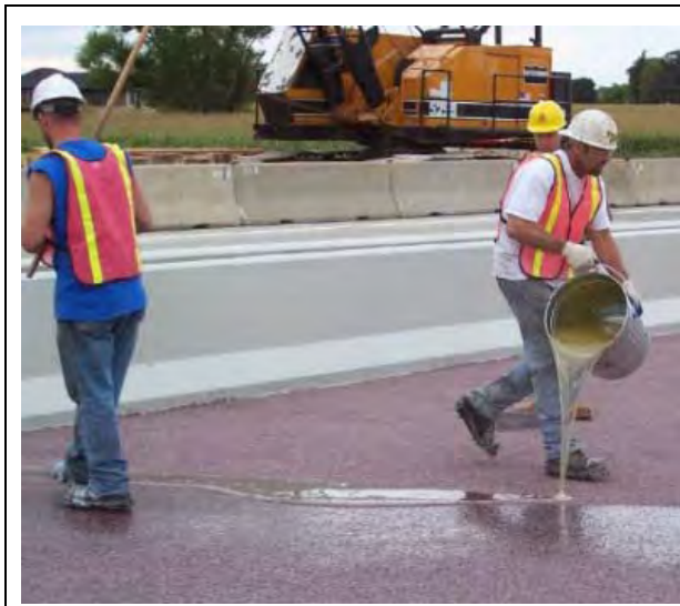
Figure 8: Application of epoxy overlay
