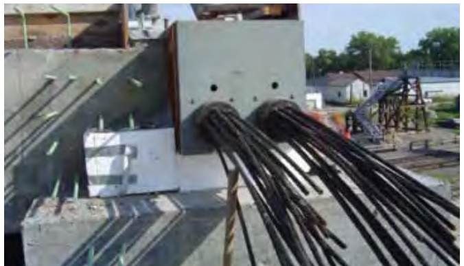
Figure 11: Post-tensioning ties at beam
