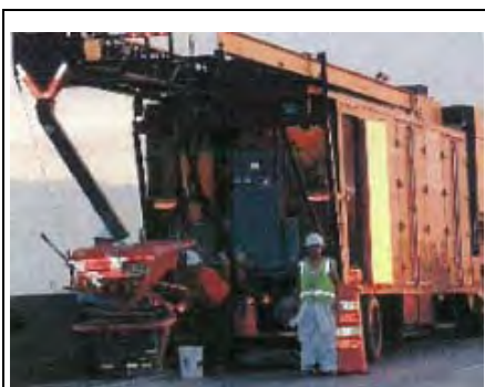
Figure 2: Truck mounted epoxy dispenser with mechanical spreader
