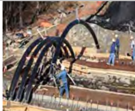
Photo 6. FRP Arches being lowered into place
