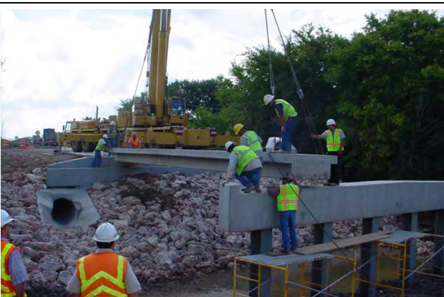
Figure 11: First girder being set into place by crane
