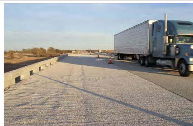
Figure 6: Surface is allowed to cure and is weather dependant – with an 85 degree air temperature curing time took 3 hours, a 60 degree air temperature would have taken 6.5 hours
