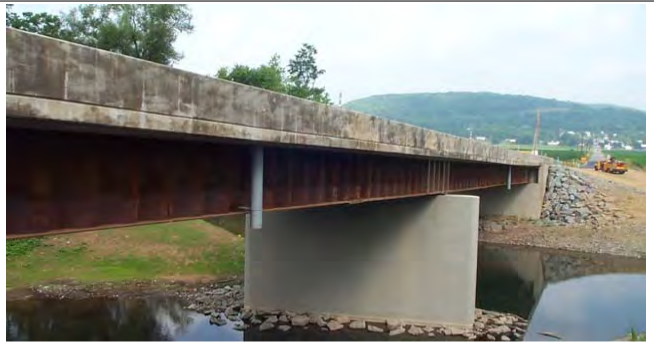
Figure 1: Completed demonstration bridge on SR-2024 over Towanda Creek
