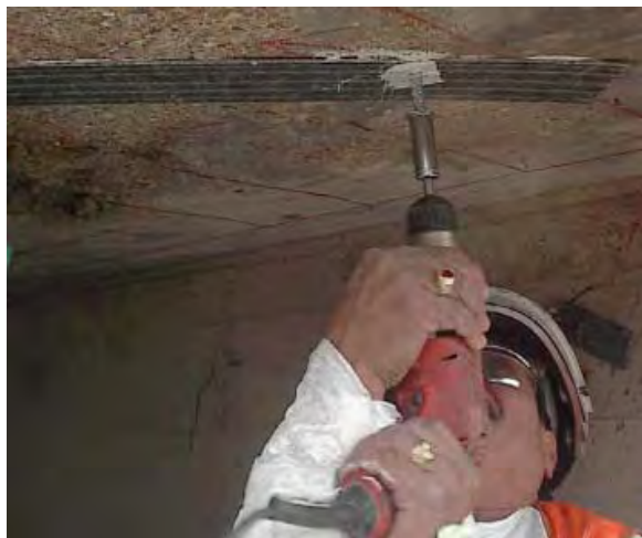
Figure 6: Mechanically fastened FRP laminates
