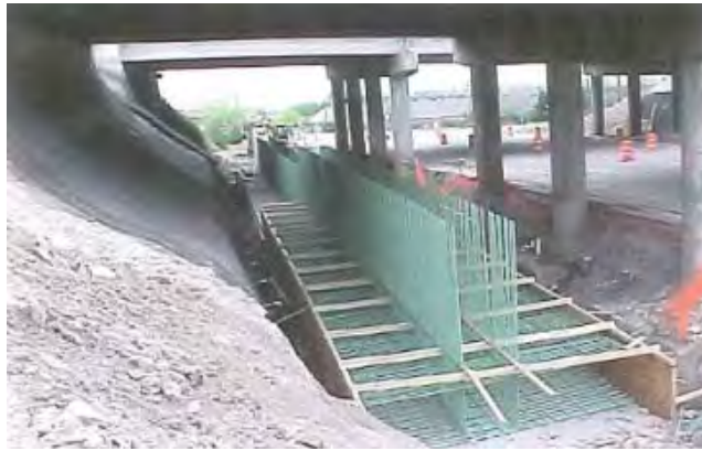
Figure 4: Formwork for spread footing under existing bridge
