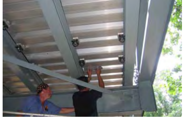
Figure 13: Panels attached to stringers with mechanical clamps
