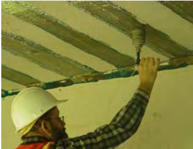
Figure 14: Pull-off test performed in field
