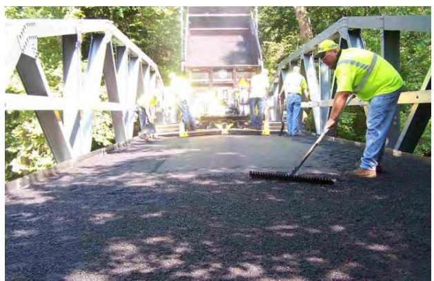
Figure 16: Placement of asphalt overlay
