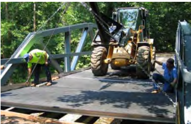
Figure 10: Panels lowered into place
