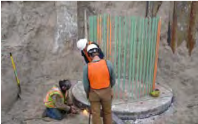
Figure 6: Construction of substructure
