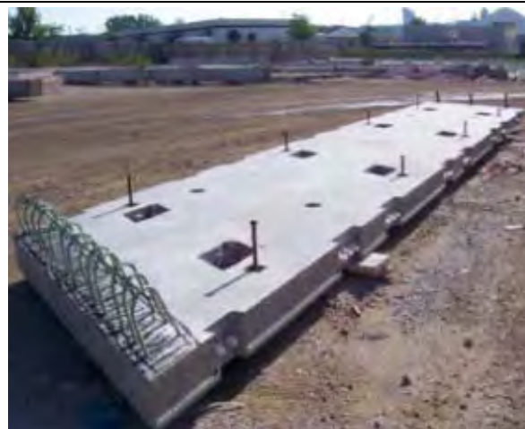
Figure 5: Completed precast concrete deck panel
