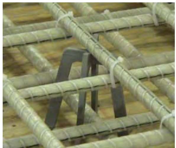
Figure 2: GFRP reinforcement
