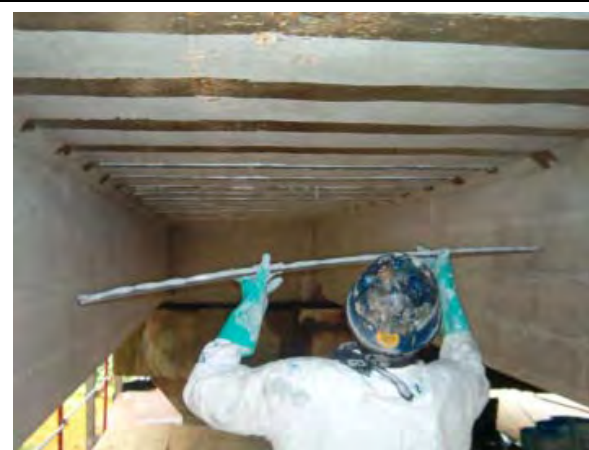
Figure 3: Pre-cured FRP Laminate Plates
