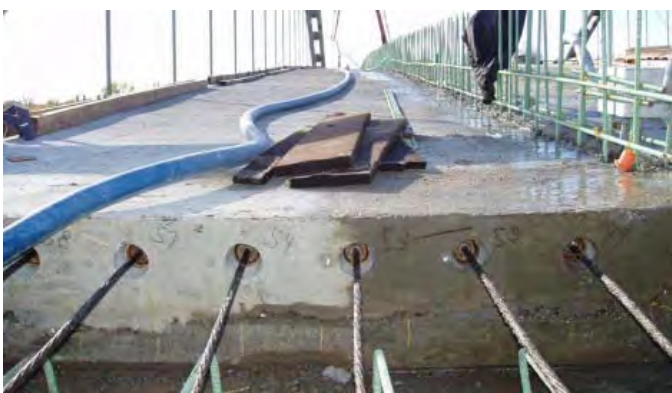
Figure 14: Deck slab post-tensioning
