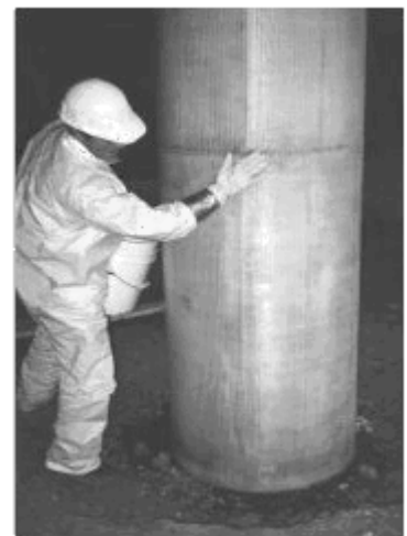
Pier concrete column after wrapping.
