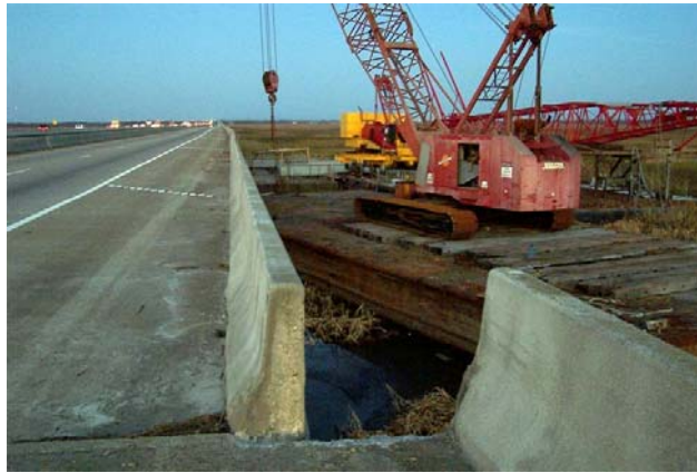
FIGURE 9 Runaway barge and damage on I-10 – Pascagoula, Mississippi.
