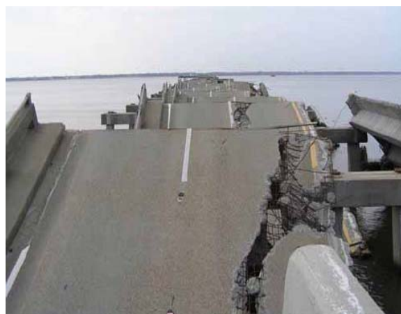
FIGURE 13 Spans split in half and fallen from piers (Bay St. Louis Bridge).
