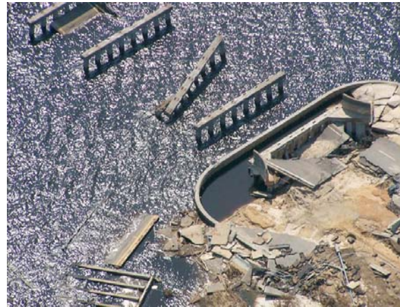
FIGURE 15 Undermined western approach, broken spans and piers (Bay St. Louis Bridge).
