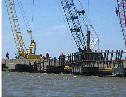
FIGURE 24 Cranes used to right the rails on NS bridge.
