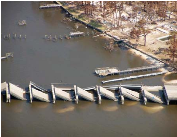
FIGURE 14 Cracked and displaced spans (Bay St. Louis Bridge).
