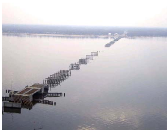
FIGURE 12 Bascule Span (lower right), lost spans (center) (Bay St. Louis Bridge).
