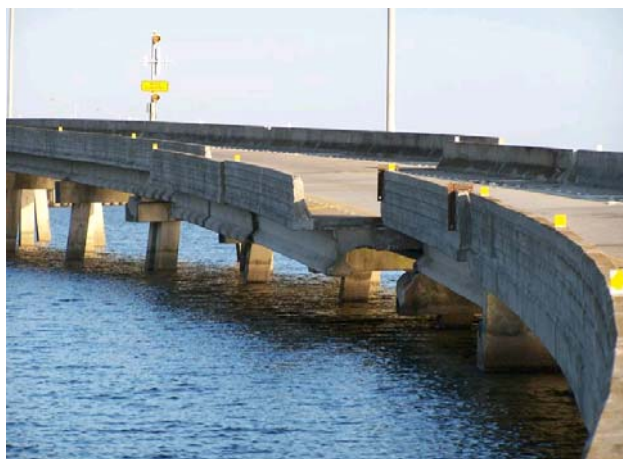
FIGURE 10 Displaced segments on I-10 – U.S. 90 ramp in Mobile Bay.
