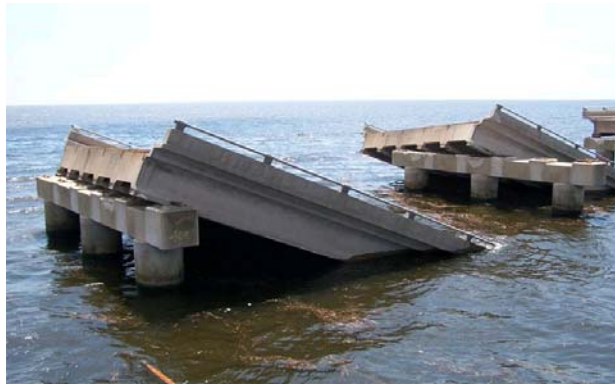
FIGURE 8 Damaged segments of the Twin Span Bridge.
