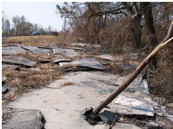
FIGURE 11 Pavement washout on U.S. 90 near Slidell, Louisiana.
