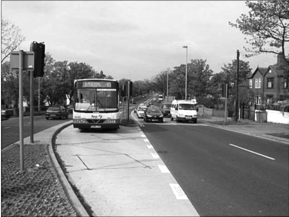
Figure 5: Busway Pre-signals (Traffic Signals Located Some 50 m Before Main Signals)
