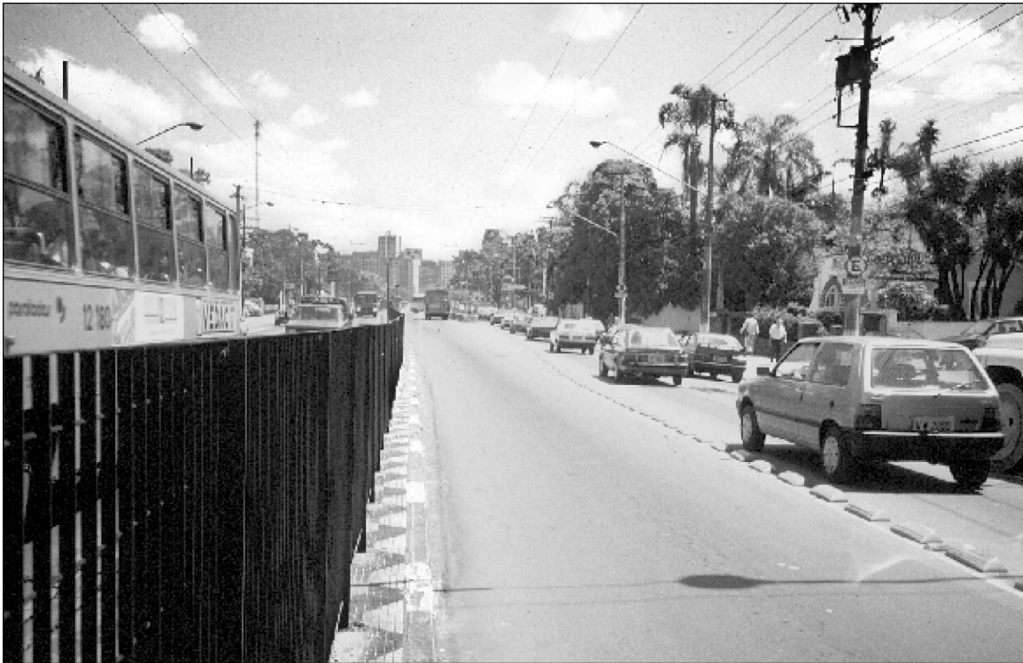
Figure 1: General View of Busway (Showing Heavy Weight Road Studs as Bus-traffic Dividers)
