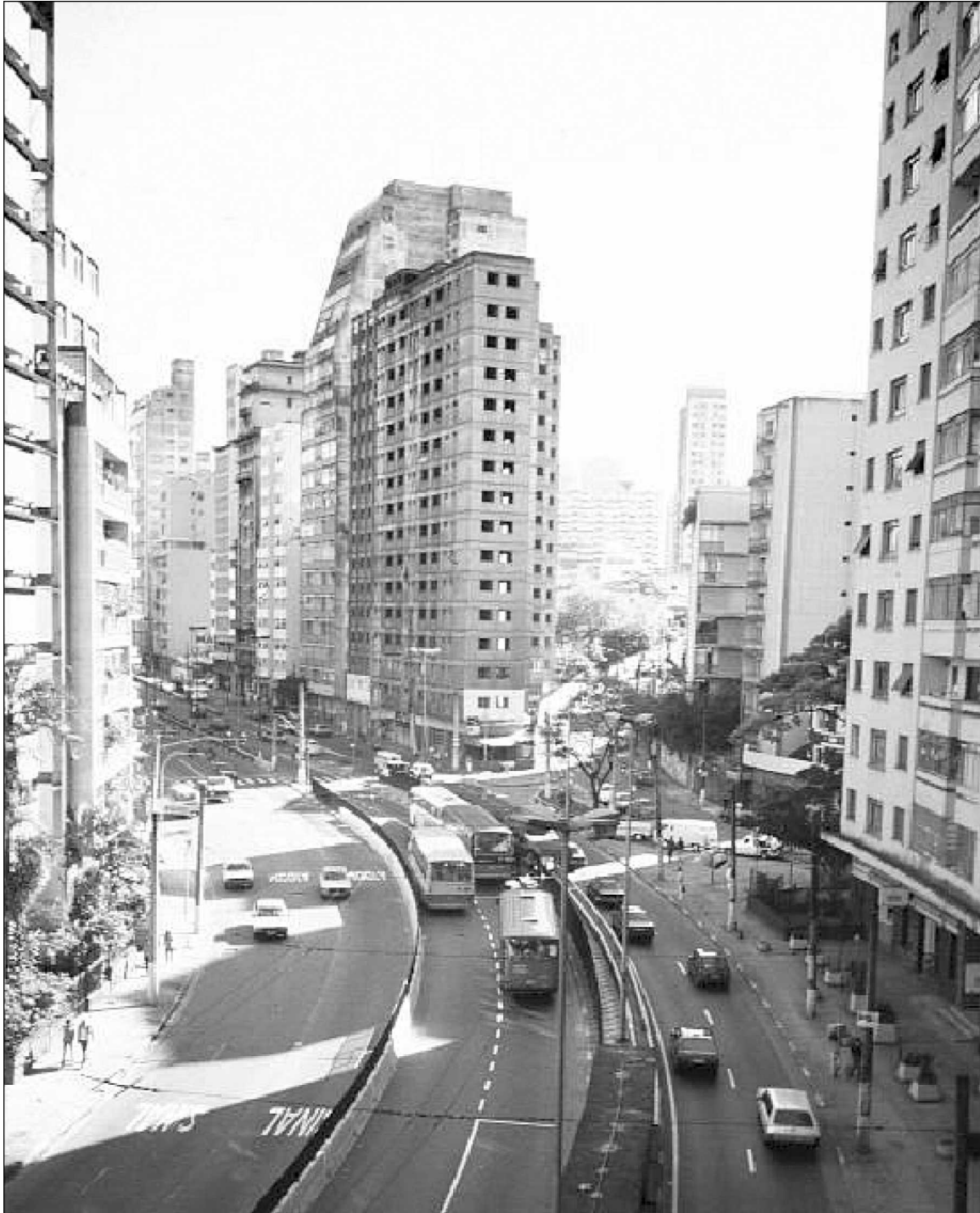
Figure 3: Busway Showing Double Width Lane at Stops to Allow Bus-on-bus Overtaking (Location Near Start of Busway and Busway Is Only One Way at this Point)
