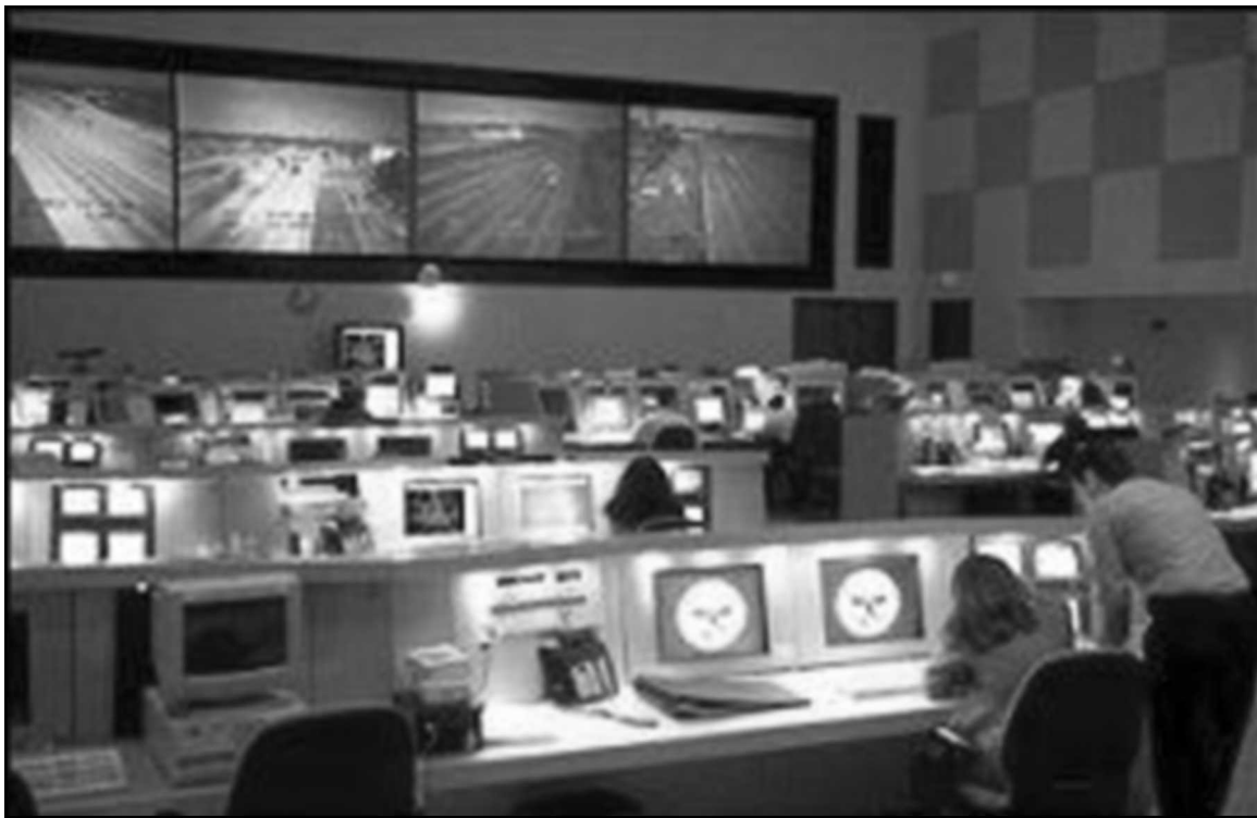
Figure 5: TranStar Control Room
