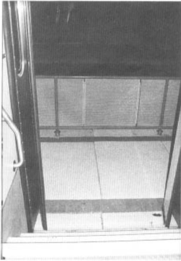
Figure 20. University Center/Baltimore St. station railing.
