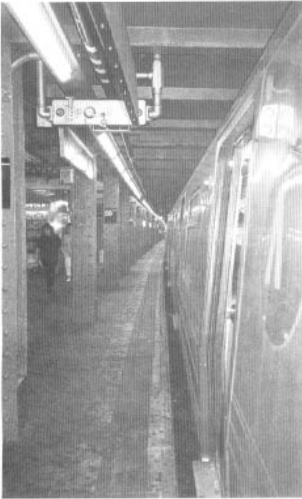
Figure 5. Columns near platform-edge obscuring conductor's vision on MTA-NYCT train.
