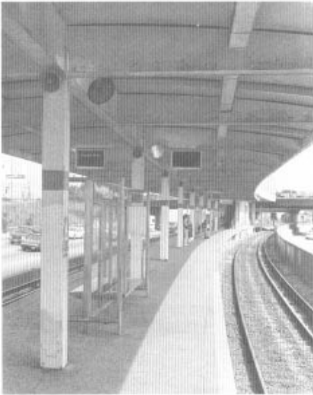
Figure 66. CTA Addison station with minimal platform column obstruction.
