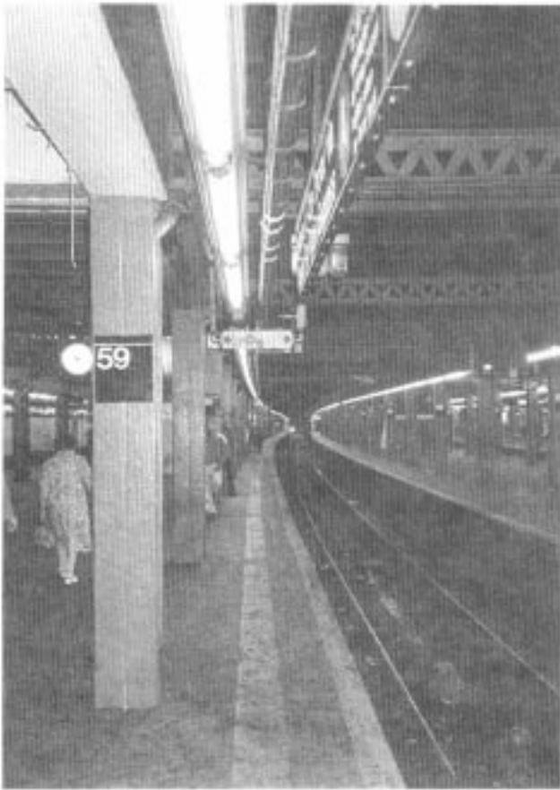
Figure 71. MTA-NYCT double line edge marking.
