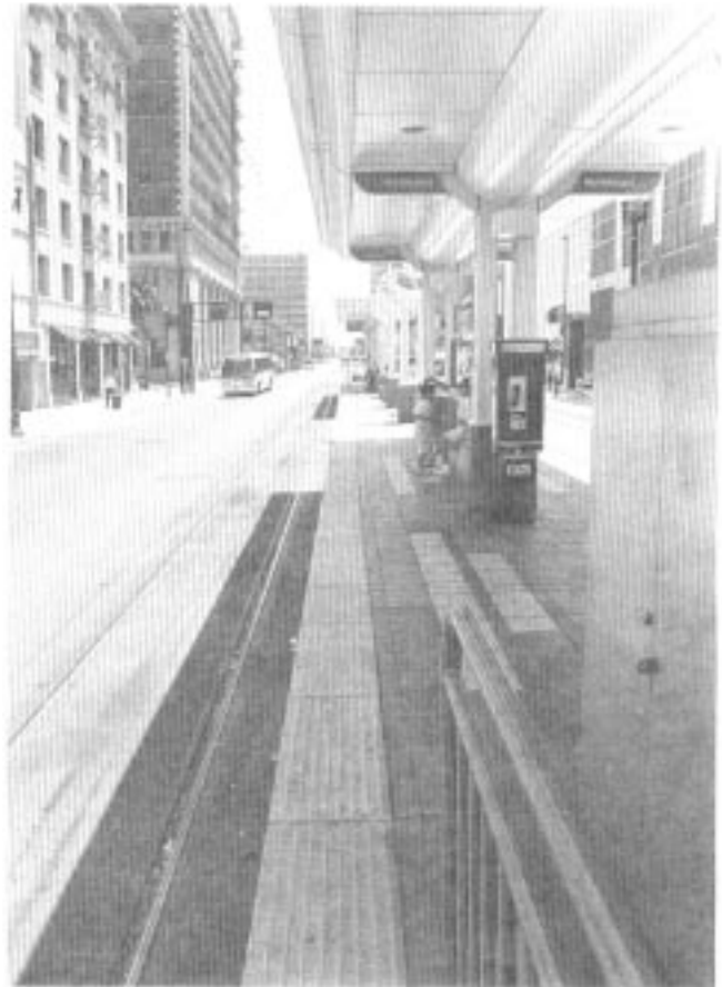
Figure 72. LACMTA Blue line scalloped concrete detectable edge warning.
