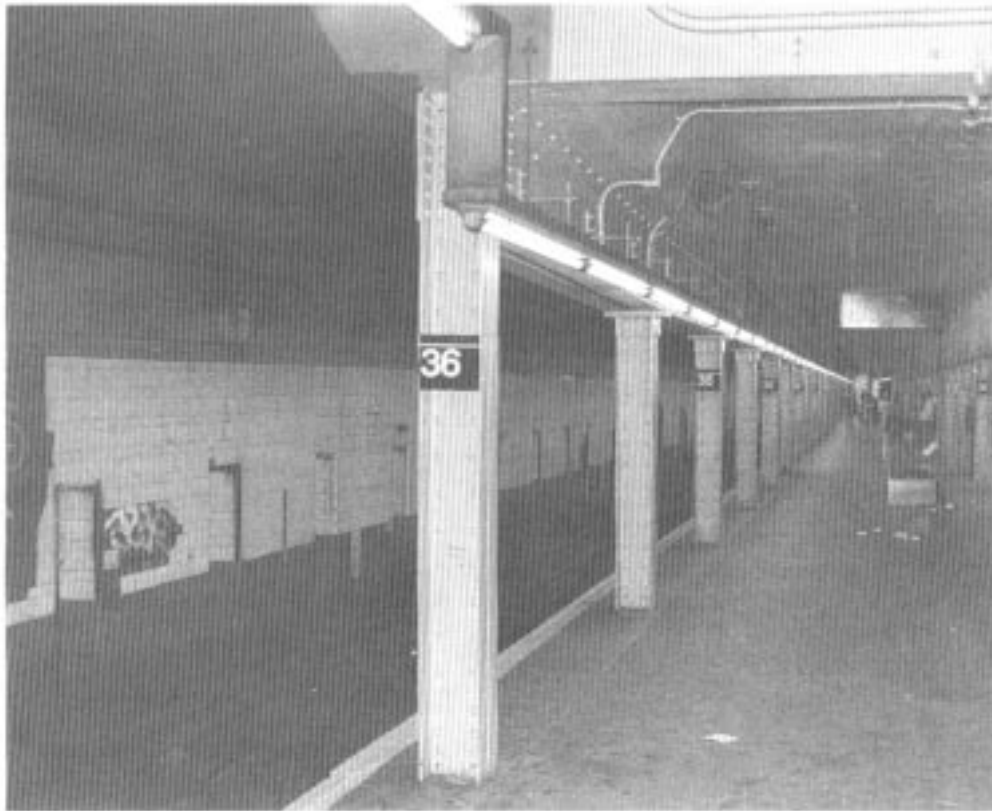
Figure 65. MTA-NYCT columns close to platform edge.
