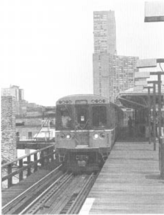
Figure 68. CTA outlying station with wood platform.
