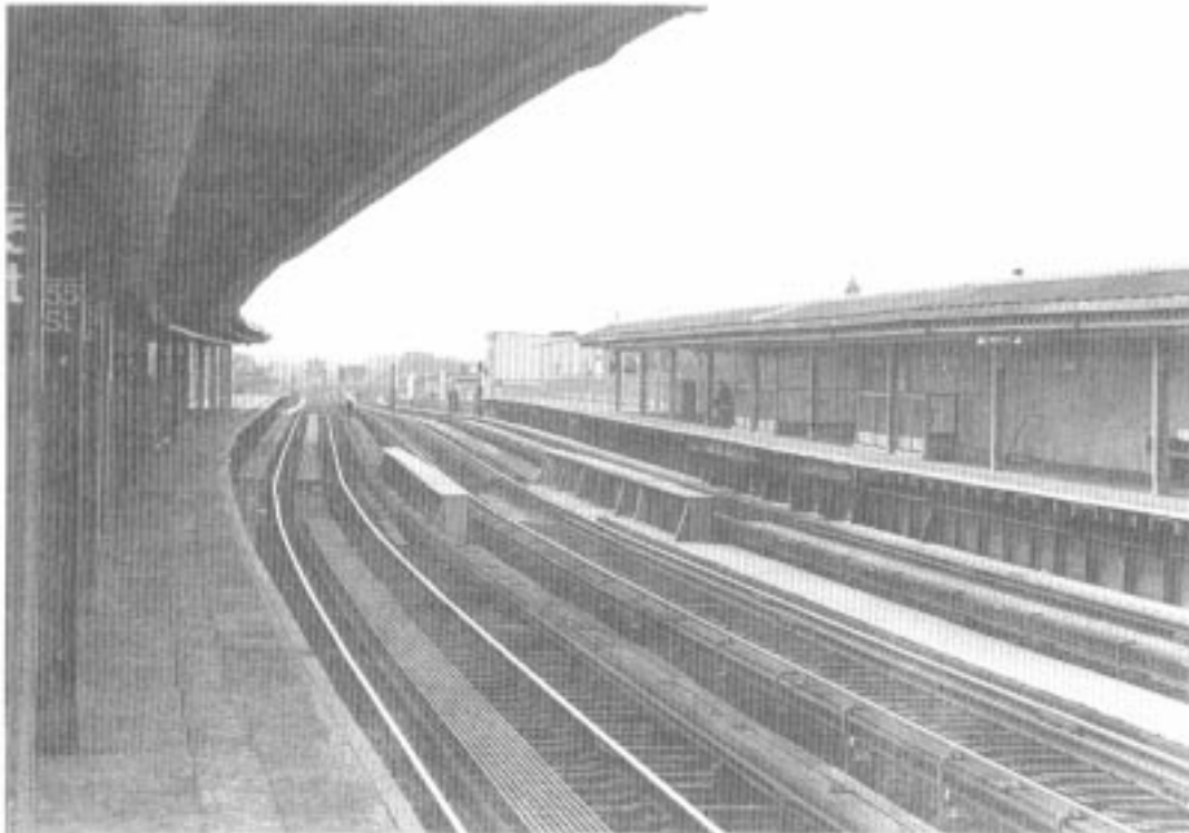
Figure 63. MTA-NYCT 55th Street station (B line) with minor curvature.
