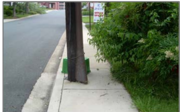
Common Problems: Utility Pole Blocks the Sidewalk and Overgrowth Restricts Usable Area
