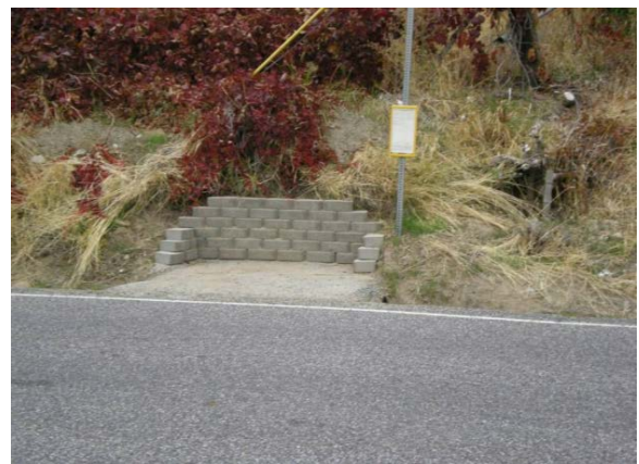
Link Transit: Improved Rural Bus Stop Using “Rhino Snot”
