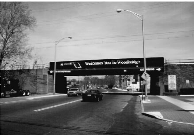
Figures 10-10 through 10-12. Case Study 10-3, Woodbridge Train Station, Woodbridge, New Jersey. The goal of this project shown here, before (Figure 10-10) and after renovation (Figure 10-11), was to create a “sense of place” for the station and to make the station more appealing to and function better for transit passengers. NJ Transit worked with the Township to turn this railroad trestle into a message of welcoming for the town and the transit facility as well. (Credit: NJ Transit Corporation)
