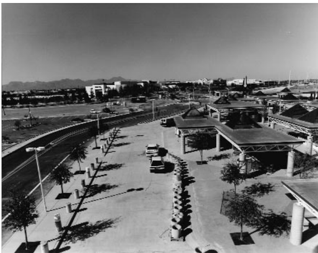
Figure 8-1. The Tohono Tada Center, Tucson, AZ, provides a focal point for development near the Tucson Mall. (Credit: Steven Haines)
