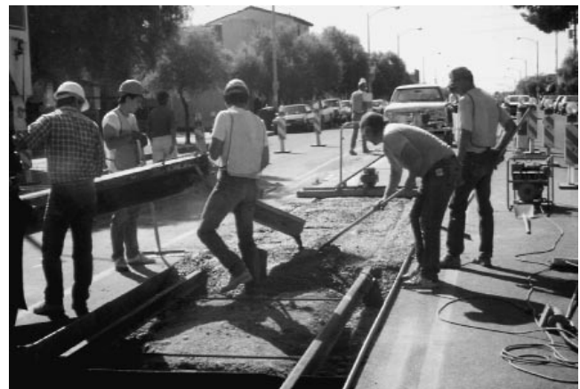
Figures 10-6 and 10-7. Case Study 10-1. Tucson's Old Pueblo Trolley was rebuilt entirely by volunteers, who continue to fundraise for its expansion as well as serve as conductors (Figure 10-6). Volunteers from the International Brotherhood of Electrical Workers uncover the original buried tracks (Figure 10-7). (Credit: Old Pueblo Trolley)
