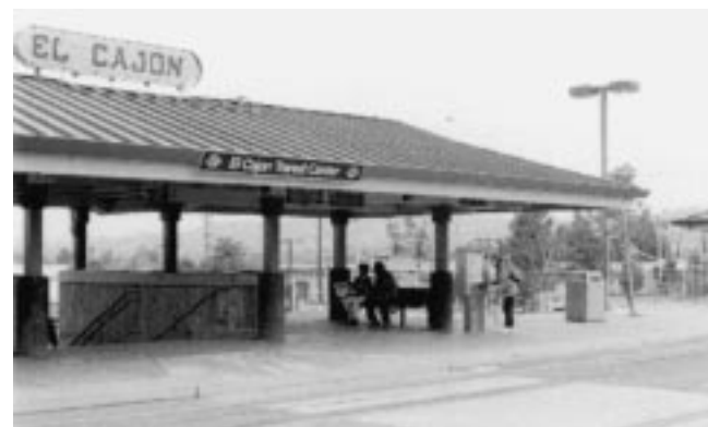
Figure 40. El Cajon Station intermodal transfer point between the San Diego Trolley and local buses and paratransit.
