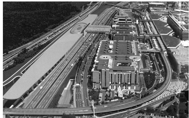
Figure 4-20. Frankfurt International Airport is now served by a new second rail station (left), which provides high-speed rail service.
