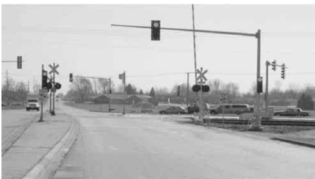
Figure 4-4. Gougar Road, Illinois. (Above: before presigned testing. Below: after.)
