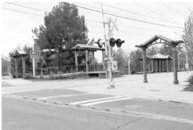
Figure 2-25. Raised steel bars in the roadway median. (Sacramento, California, 48th Street crossing.)
