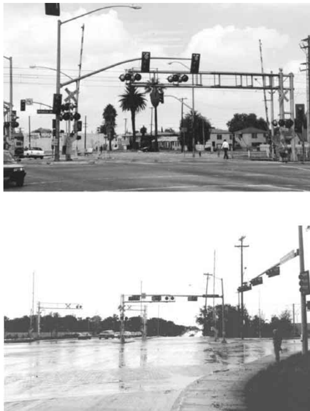
Figure 3-14. LRT crossings with cantilevered flashing light and traffic signals. (Above: Los Angeles, California. Below: Dallas, Texas.)
