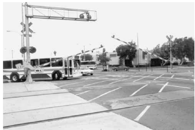
Figure 2-30. Cross-hatched striping in an LRT crossing. (San Diego, California, Broadway crossing.)
