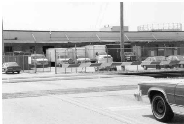
Figure 2-28. Larger lights for the top of automatic gate arms. (St. Louis, Missouri, Boyle Ave. crossing.)
