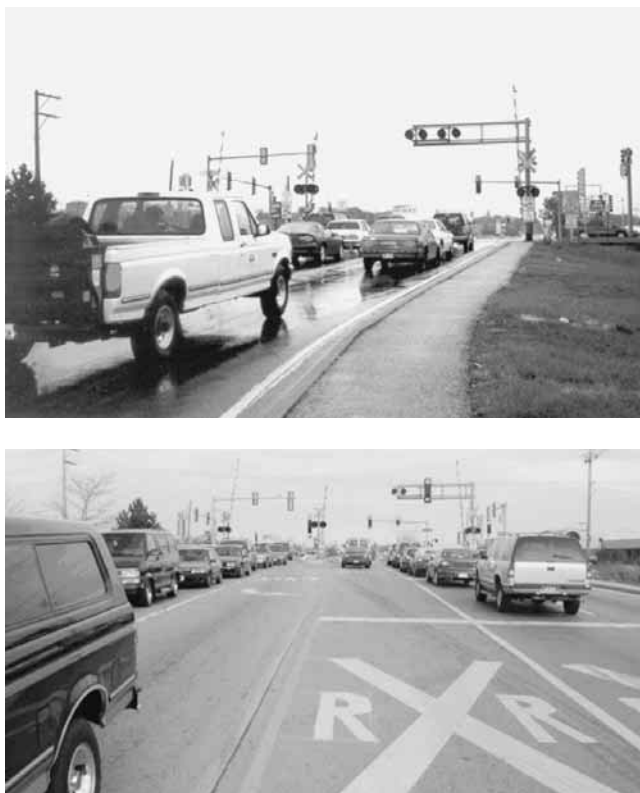
Figure 4-5. Rollins Road, Illinois. (Above: before presigned testing. Below: after.)
