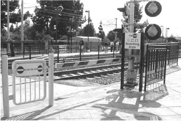
Figure 3-30. Pedestrian automatic gate and swing gate combination.
