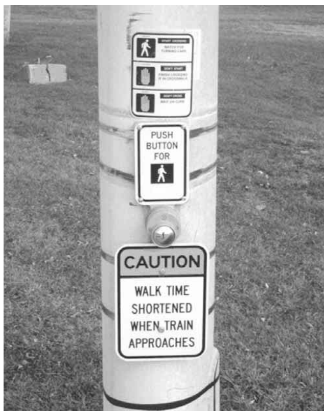
Figure 3-16. Pedestrian phase truncation sign. (Chicago, Illinois.)
