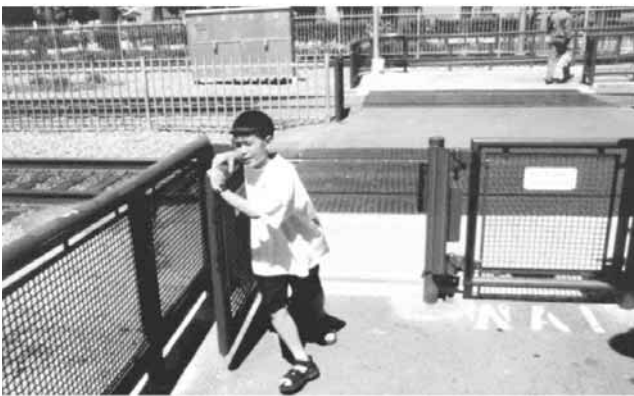
Figure 3-31. Example manual swing gates. (Above: Calgary, Alberta. Below: Los Angeles, California.)
