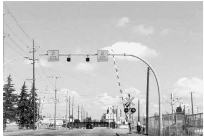
Figure 2-16. Motor vehicle queue prevention system. (Edmonton, Alberta, 66th Street crossing.)
