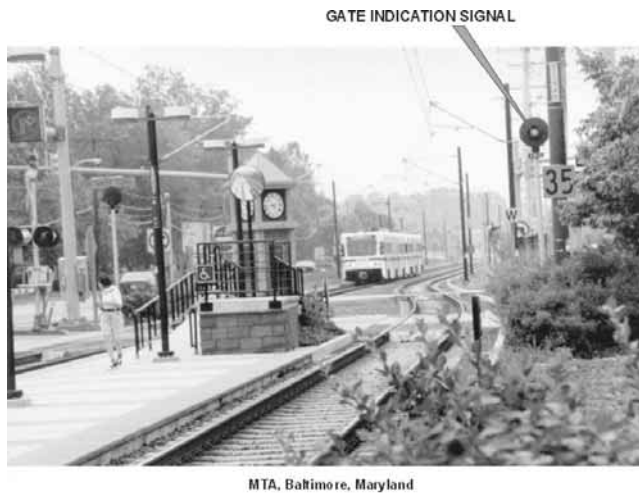
Figure 3-4. Example gate indication signal. (Baltimore, Maryland.)
