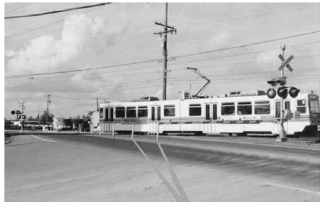
Figure 2-24. Motor vehicle channelization. (Sacramento, California.)
