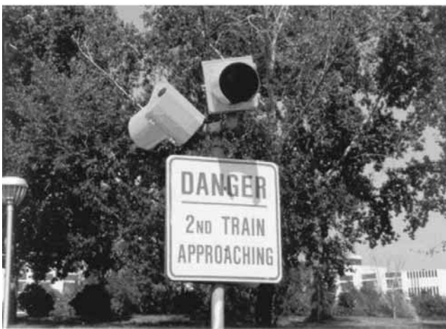
Figure 2-9. Second Train Approaching sign. (Calgary, Alberta, Canada, Southern Alberta Institute of Technology pedestrian-only crossing.)
