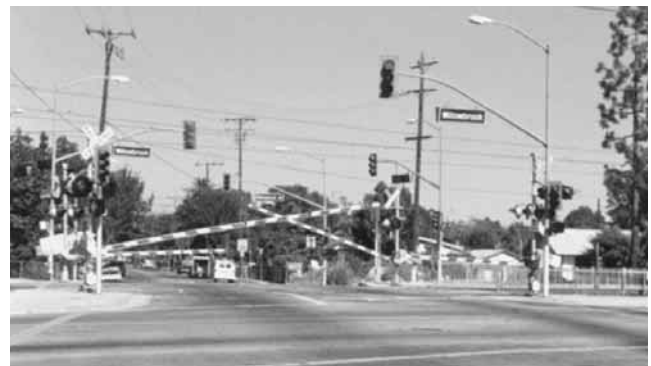
Figure 2-19. Four-quadrant gate system installation. (Los Angeles, California, 124th Street crossing.)
