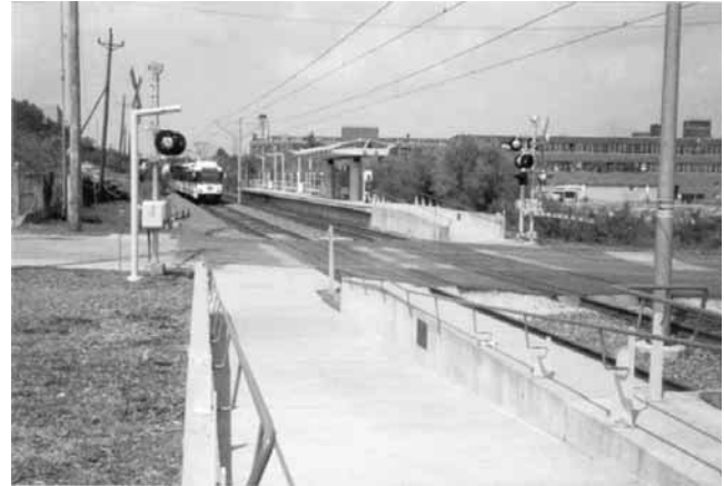
Figure 2-3. Example semiexclusive type b.1 right-of-way. (St. Louis, Missouri, LRT system, Plymouth Ave. crossing.)
