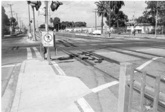
Figure 2-4. Example semiexclusive type b.2 right-of-way. (Los Angeles, California, LRT system, 55th Street crossing.)
