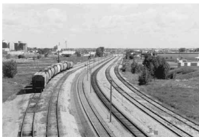
Figure 2-5. Examples of parallel LRT and railroad right-of-way. (Above: Denver, Colorado. Below: Edmonton, Alberta, Canada.)
