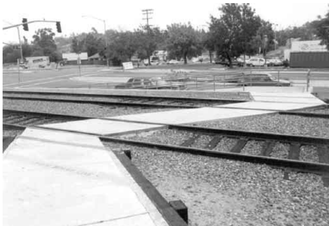
Figure 2-31. Pedestrian Z-crossing. (City of Lemon Grove, California.)
