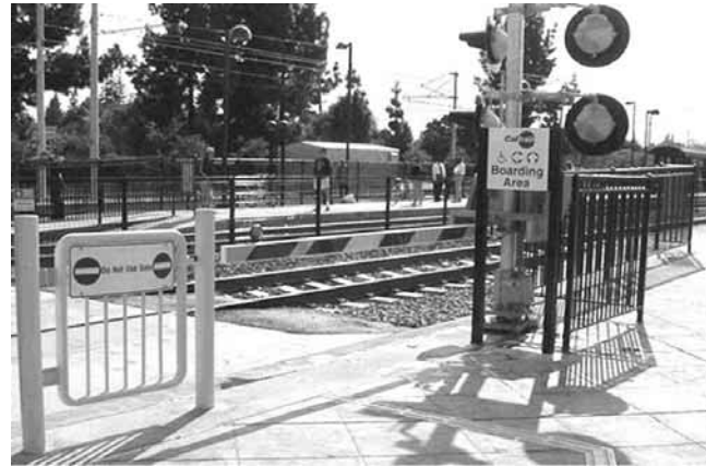
Figure 2-35. Pedestrian automatic gate and swing gate combination.
