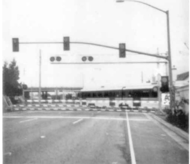
Figure 2-34. VTA barrier gate.
