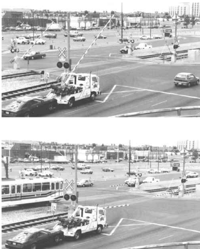
Figure 3-25. Example quasi-four-quadrant gate system. (Calgary, Alberta.)
